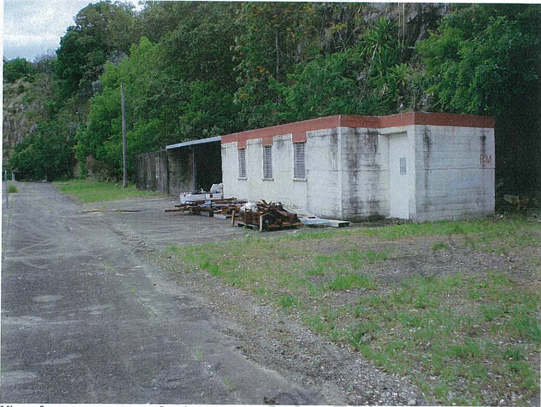
View of masonry structure on Lot 4
