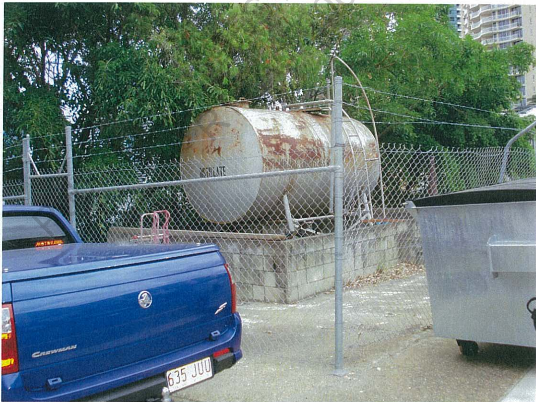
View of disused diesel AST (Lot 3).
