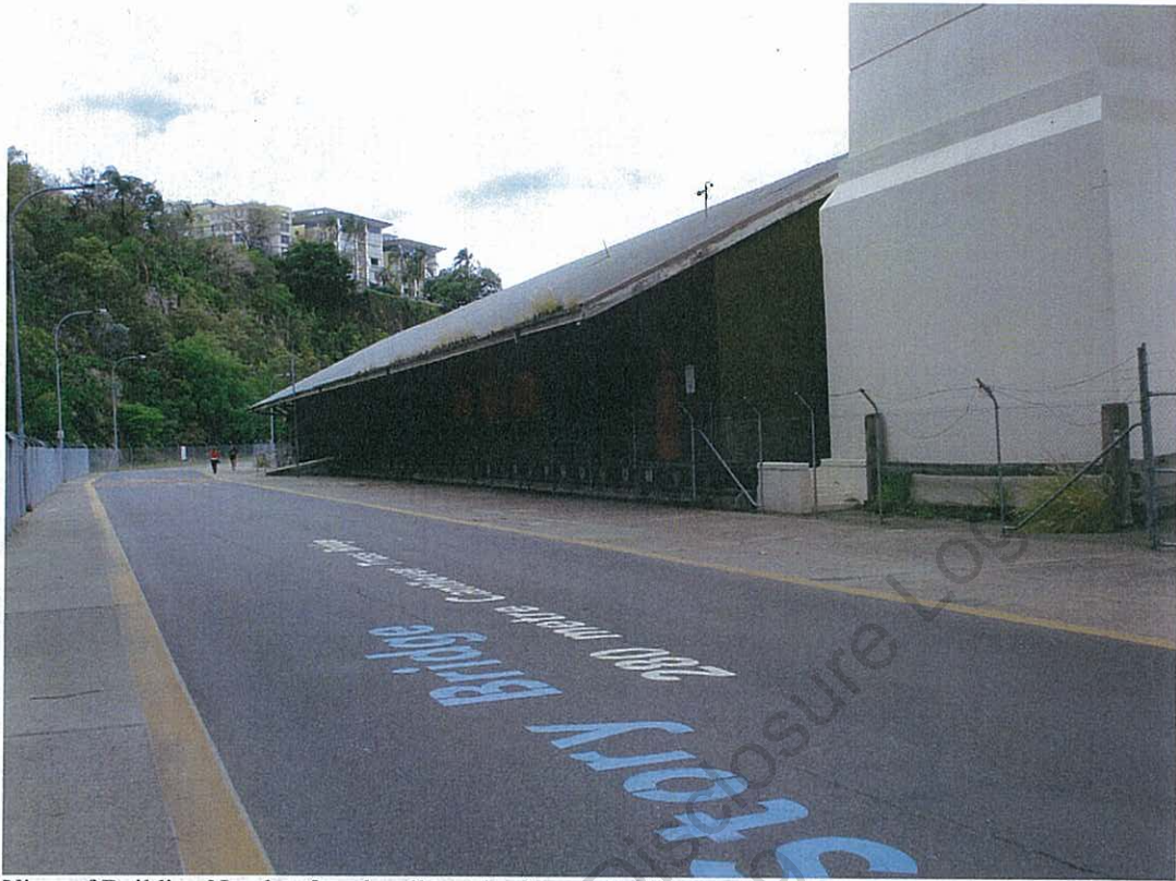
View of Building Number 3 and walkway/cycle way looking east.
