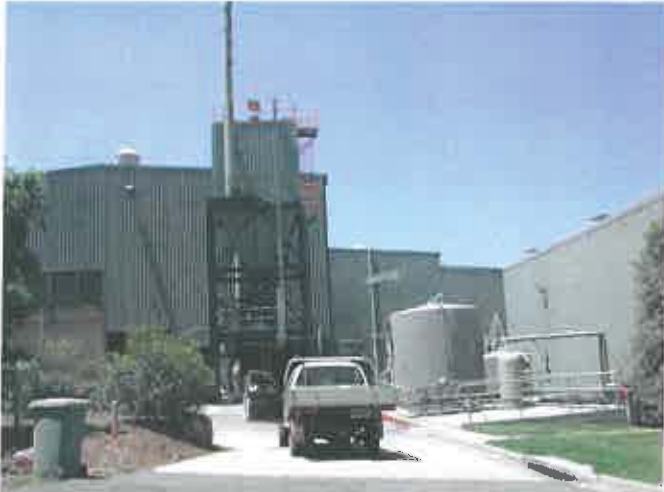
Photo 3 – New baghouse installation on the Finafire coal-fired Boiler.
