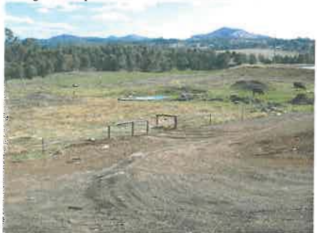
Photo. 29: Main "catch dam" servicing the hardstand surrounds to the gelatine processing plant, which acts as a "first-flush" catchment holding pond, prior to processing in the Aerobic Pond of the effluent treatment system. The facility was noted to be holding minimal accumulated material at the time of the site inspection.
