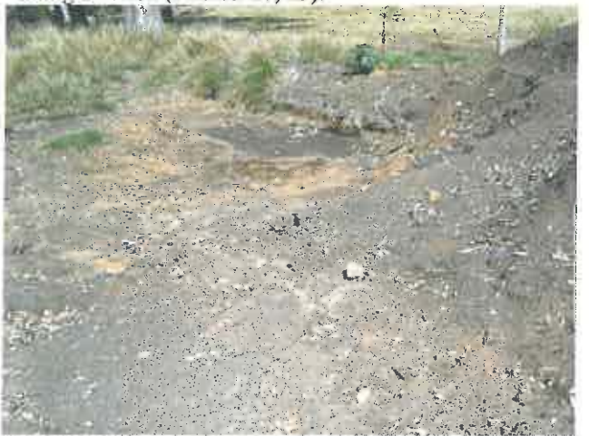
Photo. 25: An example of a sediment detention basin, which accepts runoff from the formed perimeter drainage swale surrounding the asphalt-sealed composting area (Photo. 18), prior to overtopping to the downstream "catch dams" (Photo. 28).
