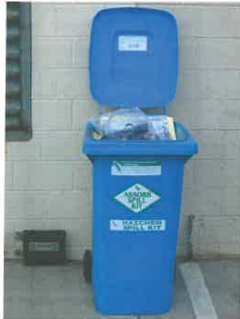
Photo. 33: Example of a site Spill Kit showing adequately stocked "clean-up" materials and unit servicing log attached to the inner surface of the lid.
