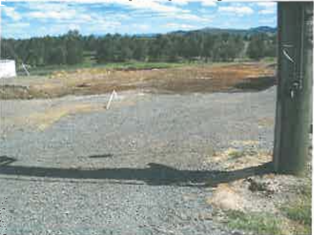
Photo. 2: Previous location of the "Stables" chemical store, demolished to make way for a new site Workshop facility.
