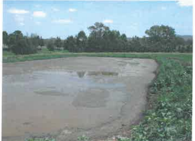
Photo 6 – New salted hides washings collection / evaporation pond, some of which highly saline material will be reused for "raw" hides salting purposes.
