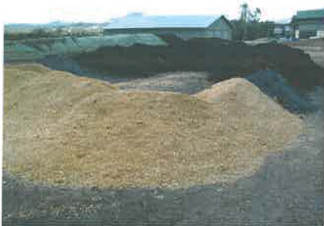
Photo. 22: Raw materials placed for a compost mixing "batch" showing a circular belt press sludge, sawdust, fly ash, paper ash and green waste mixing "dam" prior to "scutch" addition to the centre "dam" area.
