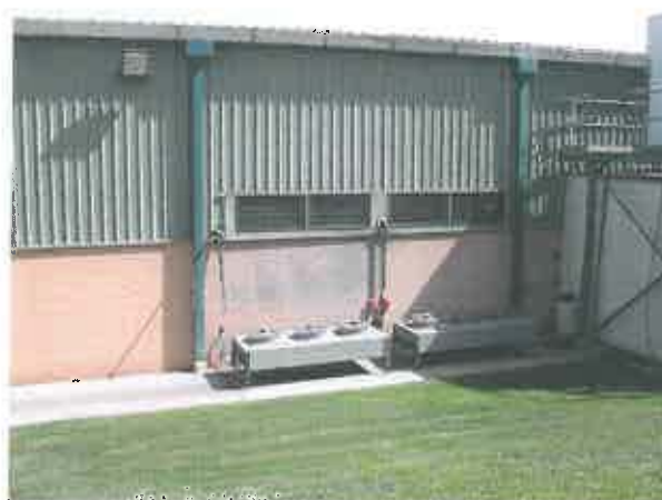
Fig 4: Refrigeration motors are located away from any potential complainant. This area backs onto an incline which assists in controlling noise from these motors.
