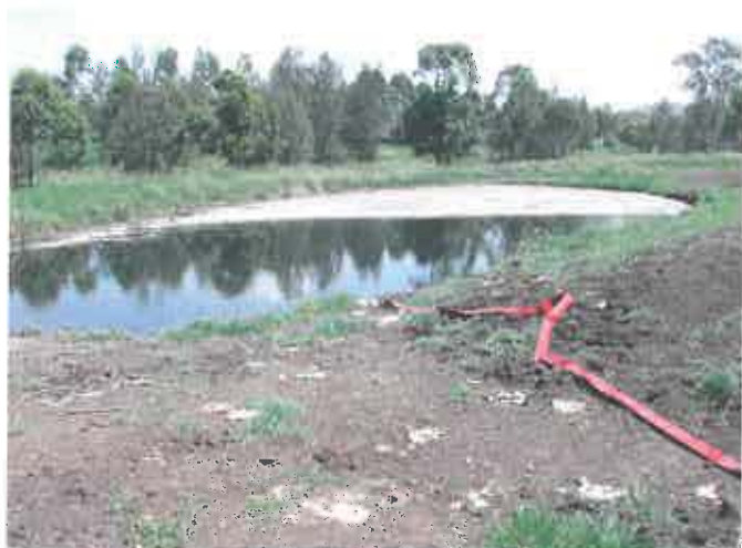
Photo 7 – New backup "catch dam" adjacent to the salted hides washings collection / storage / evaporation pond.
