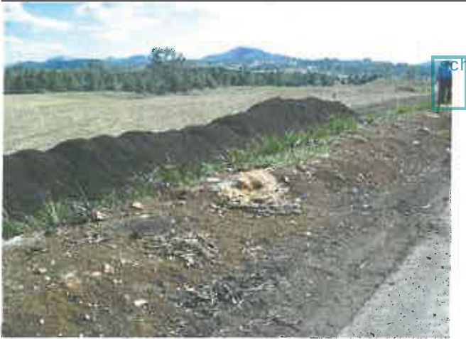
Photo. 26: "Finished" compost maturing stockpile accumulated on a "packed clay" storage area adjacent to the mixing pad awaiting use. No odour was noted with this material. Runoff from this area also drains to the dedicated surrounding swale, sediment basin and "catch dam" system on site.
