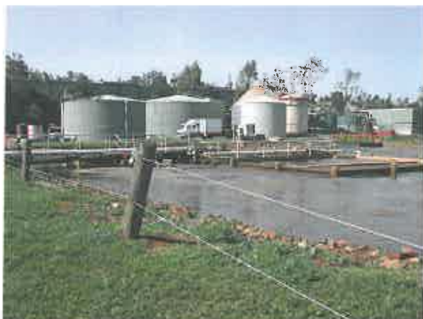
Fig 15: Overview of the wastewater treatment plant and Aerobic Pond 1.
