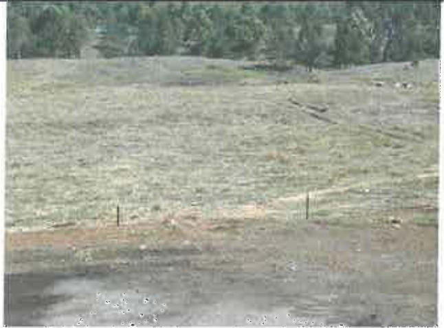
Photo. 28: Main "catch dam" servicing the composting area to collect runoff directed by the perimeter drainage and sediment basin system (Photos. 18, 25) for holding prior to processing in the Aerobic Pond of the effluent treatment system. This facility was noted to be empty during a subsequent "drive-tour" of the site.
