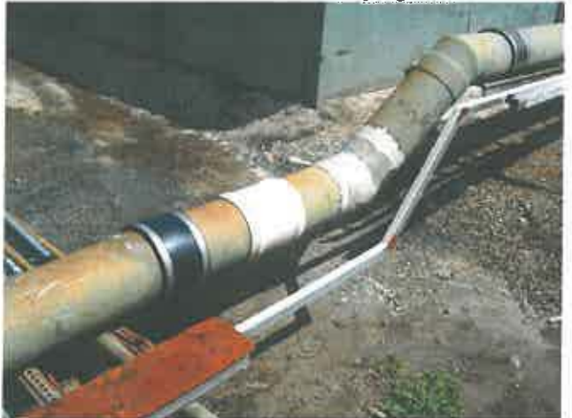
Photo. 5: Further gas supply line maintenance completed to minimise odorous gas releases to atmosphere, showing new expansion joint sleeves (black), together with a replaced/repaired line bend (centre). Many metres of corroded cable trays and covers (bottom, left) have also been replaced throughout the effluent treatment plant as a safety "due diligence" measure.
