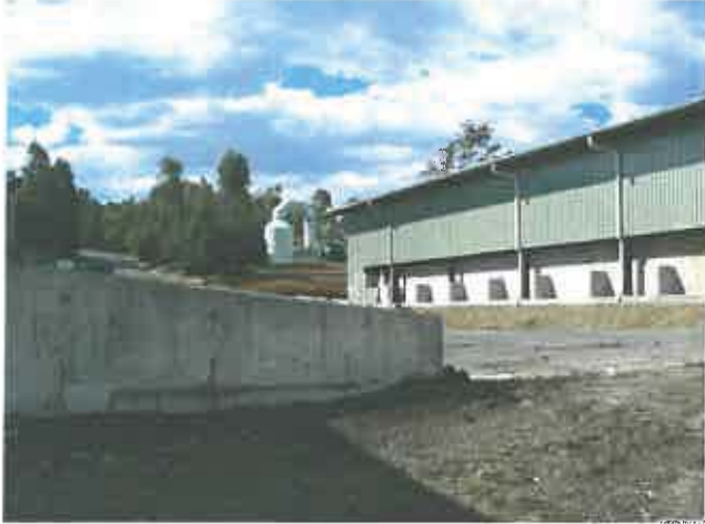
Photo. 30: New Hide Storage Shed recently put into use at Josephville. The company proposes to progressively transfer "back-up" material from rental storage in Redbank to this on-site facility. The new store is situated between the belt press shed (left) and the composting operation (far right) and below the large Biofilter (centre).
