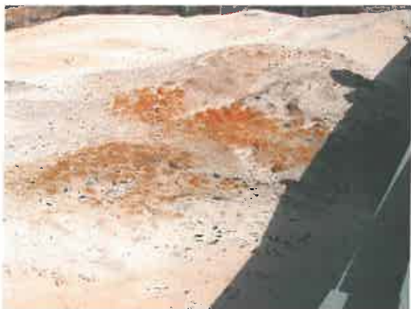
Fig 13: Sulphur crystals forming on the top of the biofilter media.
