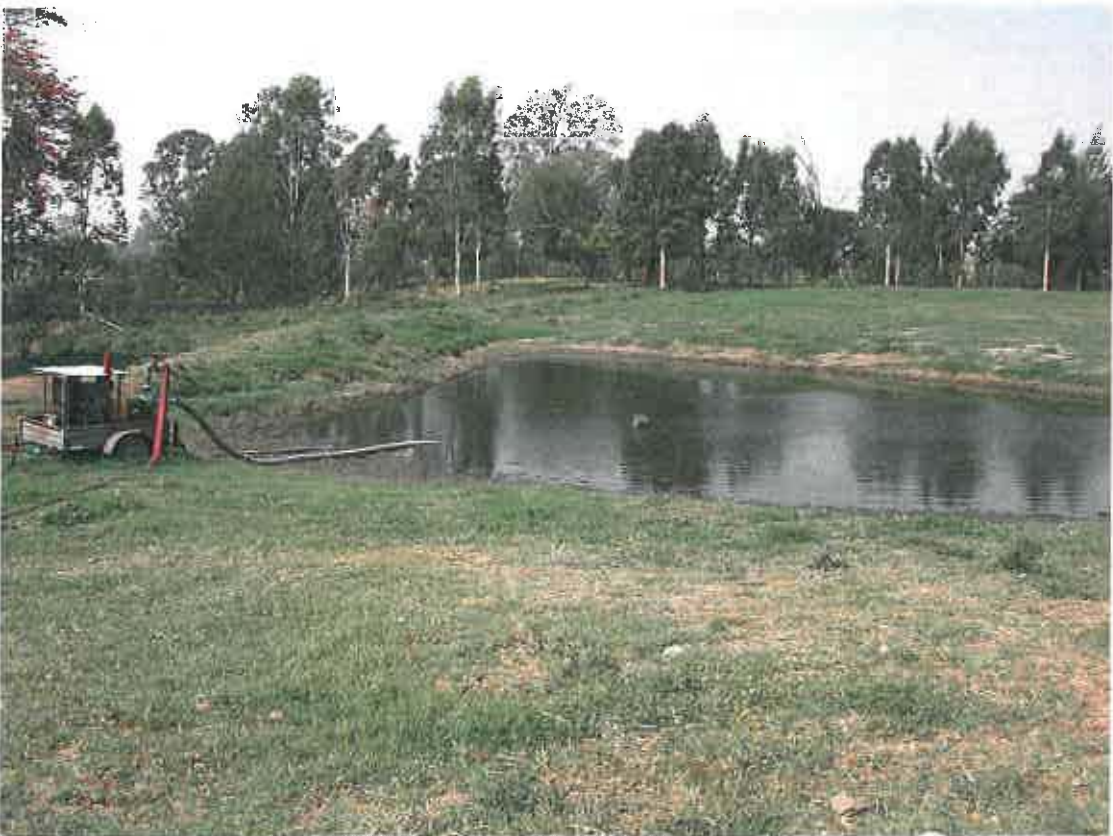
Figure 20: Various trap dams such as this are located around site
