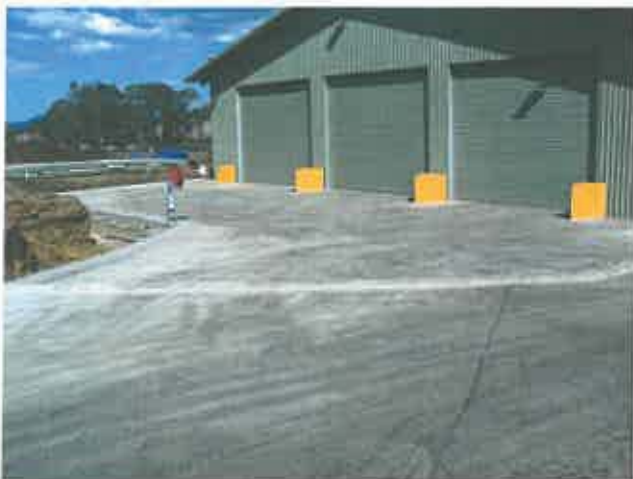
Photo. 31: Front view of the new Hide Storage Shed showing stormwater diversion, roll-over bunds surrounding the front of the facility. The composting operation is visible in the distance at the top left corner.
