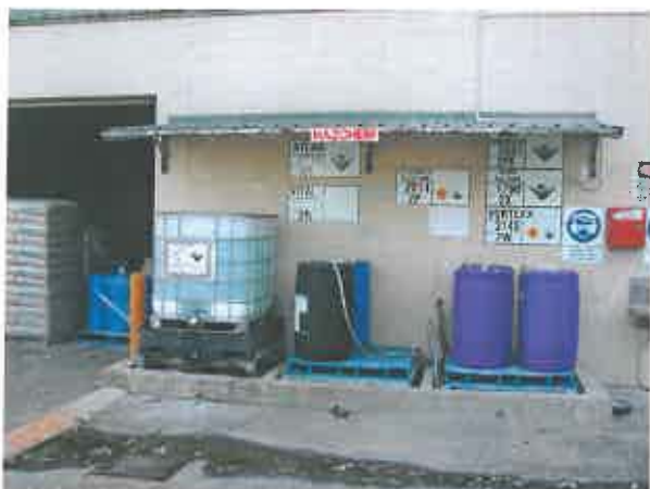
Fig 9: Bunded cleaning chemical storage area and bunded unloading pad.
