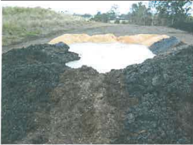
Photo. 21: Raw materials placed for a compost mixing "batch" showing a circular belt press sludge, sawdust, fly ash, paper ash and green waste mixing "dam" with wet/semi-liquid "skutch" unloaded into the centre for mixing/incorporation with the dry solids. "Scutch" is transferred from the gelatine plant using a tractor-hitched enclosed tanker.
