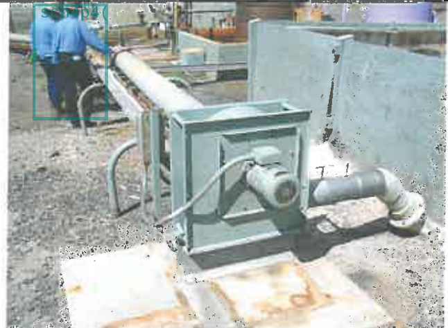
Photo. 4: The Hybractor Technology Biofilter gas supply fan was replaced in December 2003 with a sealed unit to obviate leakage of odorous and corrosive air to atmosphere. Such on-going maintenance measures have significantly minimised local odour leakage, compared to previous audits/inspections. Portion of the upgraded Biofilter media box is visible at the top right.
