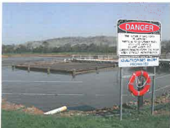
Fig 14: Aerobic wastewater treatment pond.
