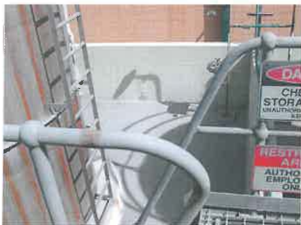
Fig 2: Shows the interior of the bulk materials storage bund. The interior is lined with a resistant polymer to prevent the material eroding the bund wall.
