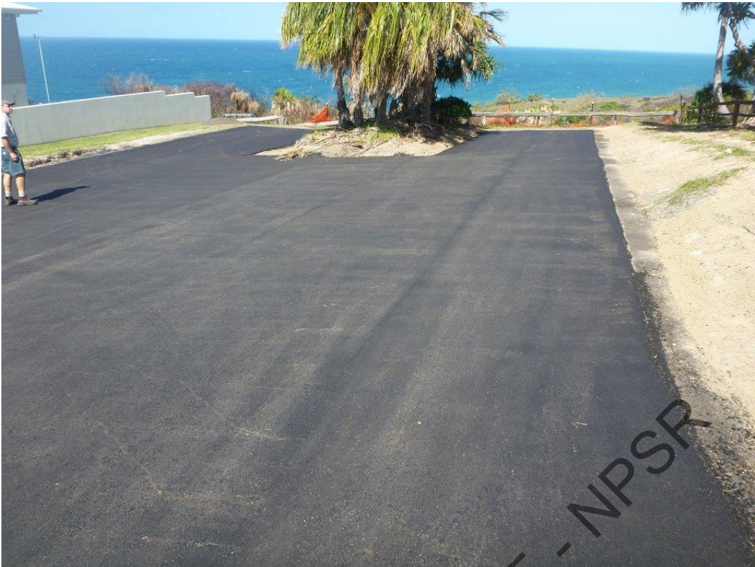
Image 1 – Tupia Street Car Park (under construction by Gladstone regional Council) commencement of track.
