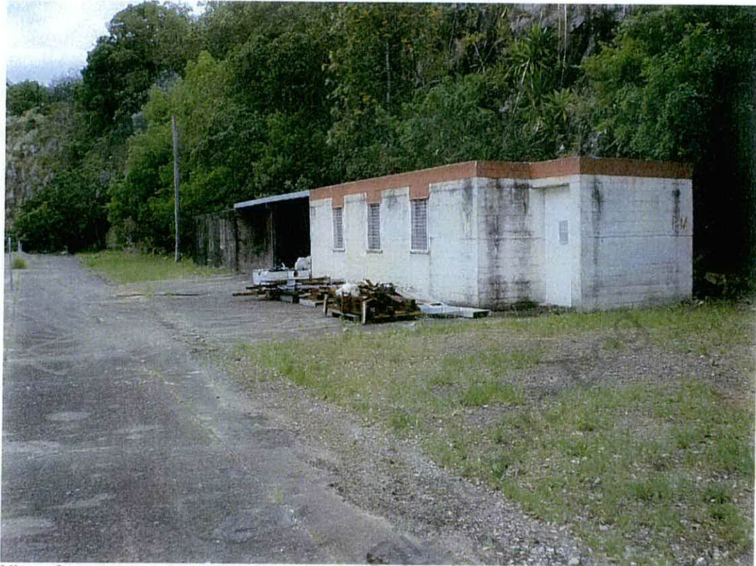
View of masonry structure on Lot 4
