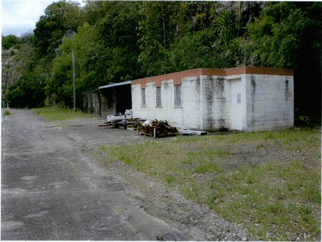
View of masonry structure on Lot 4
