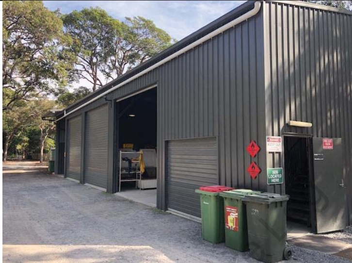
Image 3: Front entrance to the depot which appeared in excellent condition.
