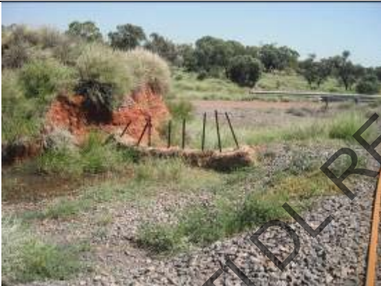
Figure 3: Release point/spillway of stormwater settling pond.
