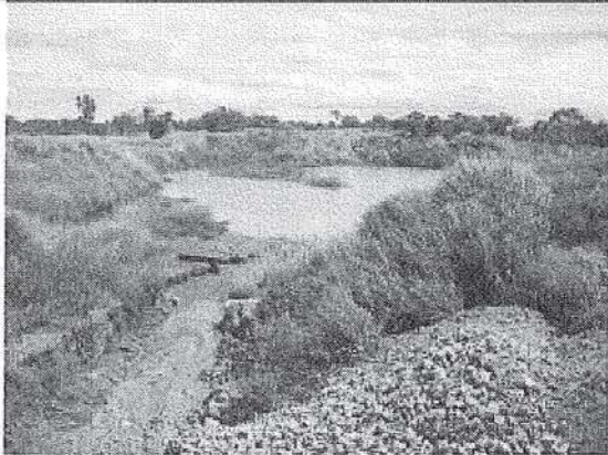
Figure 1: Stormwater settling pond.
