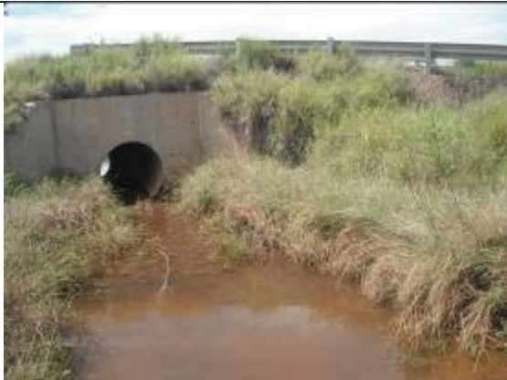
Figure 4: Downstream of the creek, about 30~40m from spillway of stormwater settling pond.
