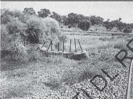
Figure 3: Release point/spillway of stormwater settling pond.
