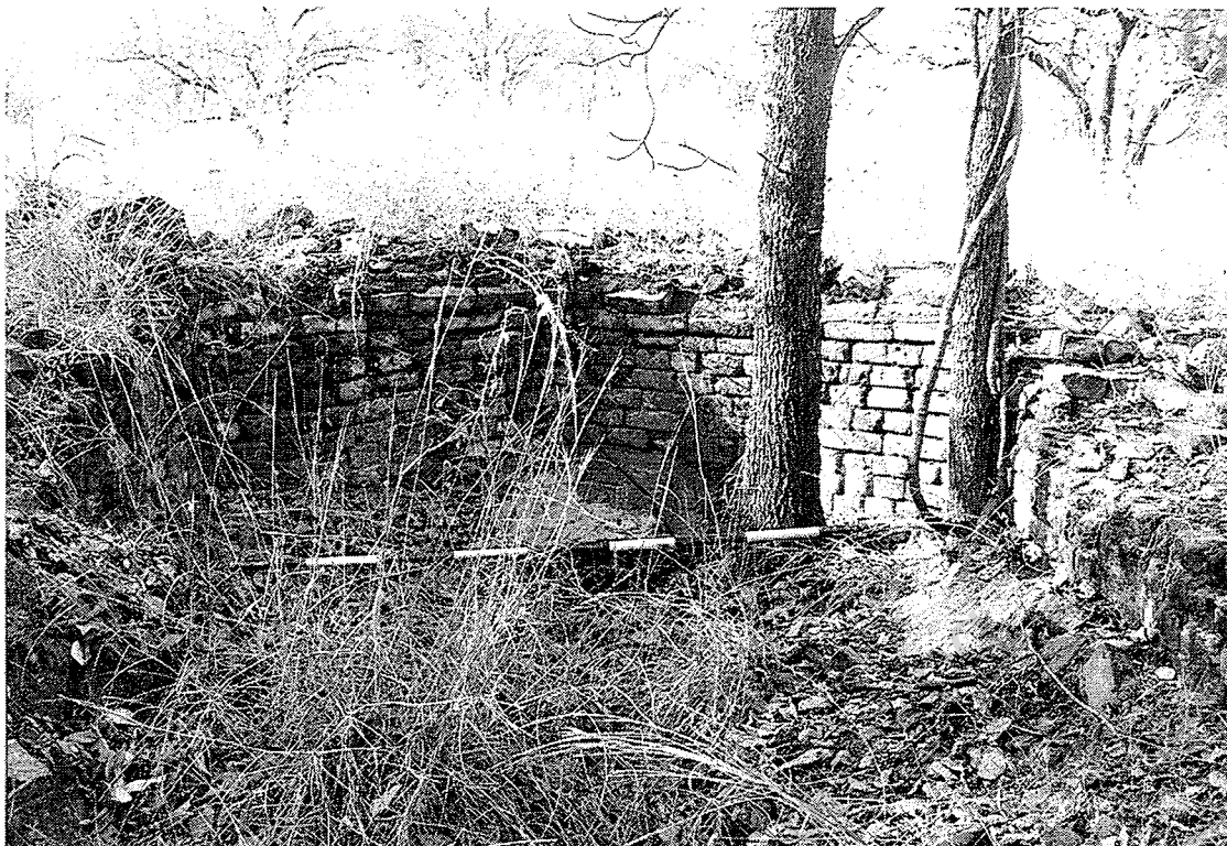
Cornish boiler mount showing firebrick retaining wall and flue. Looking NE.
