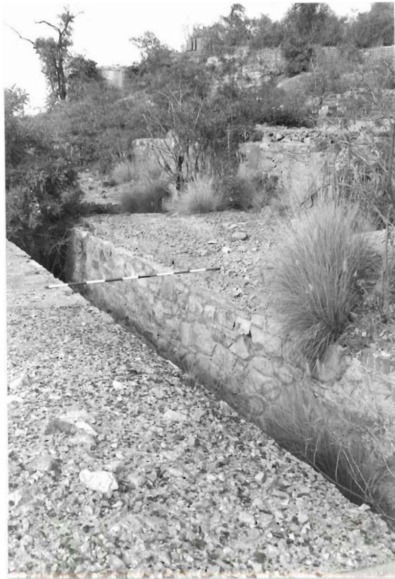
Chlorination plant foundations with broken glass scatter, looking S.
