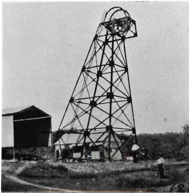
Steel headframe and winding engine shed (left) at the Louisa mine. Q.G.M.J. 15 May 1915, p.216.
