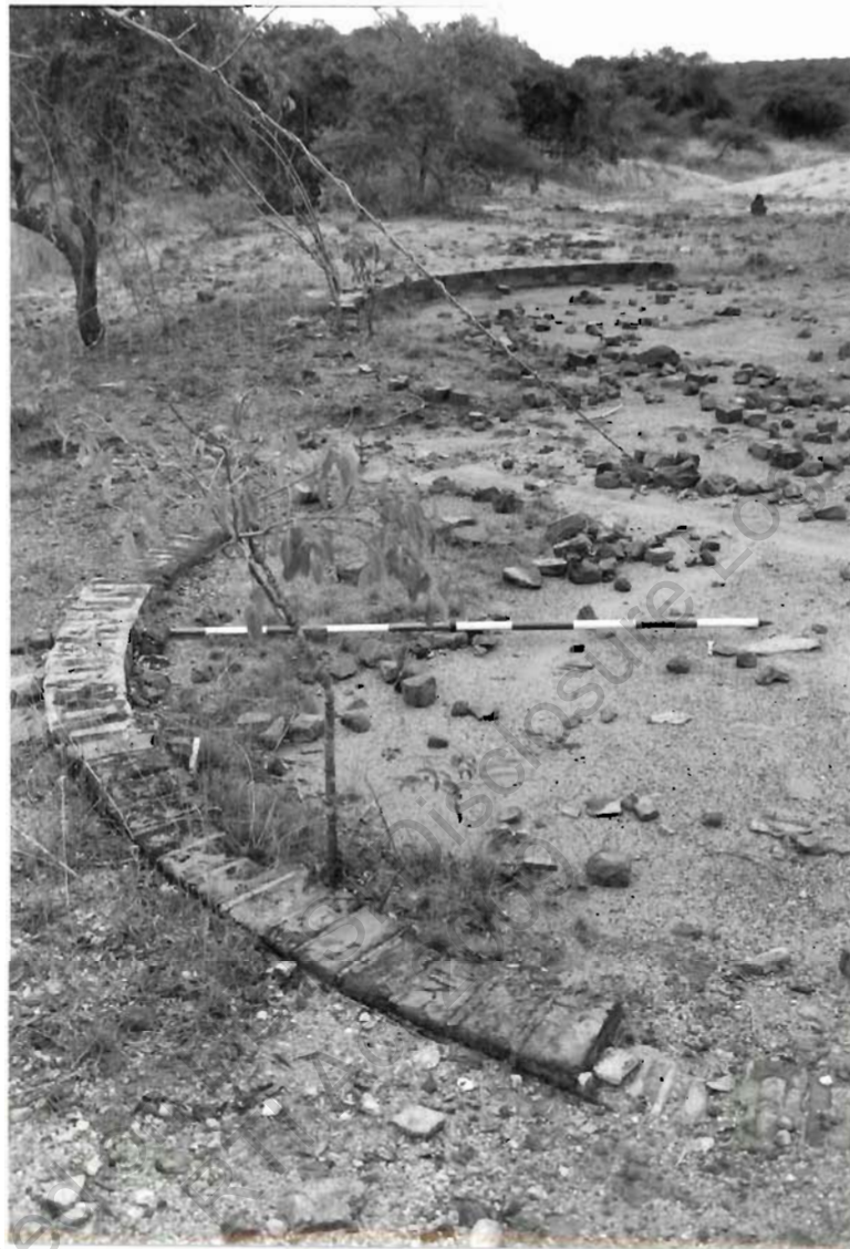
Tank base brickwork, looking S.
