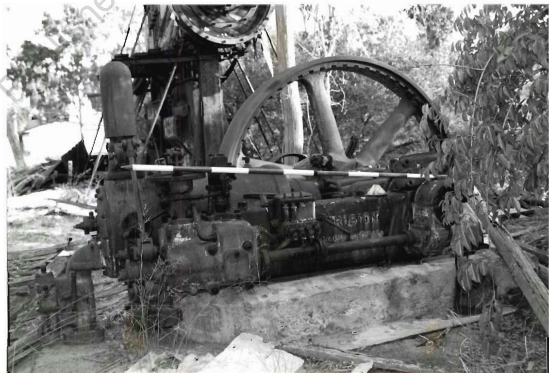
Ruston gas engine, looking S.
