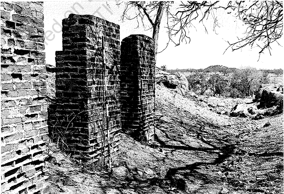
Tramway formation with brick piers.
