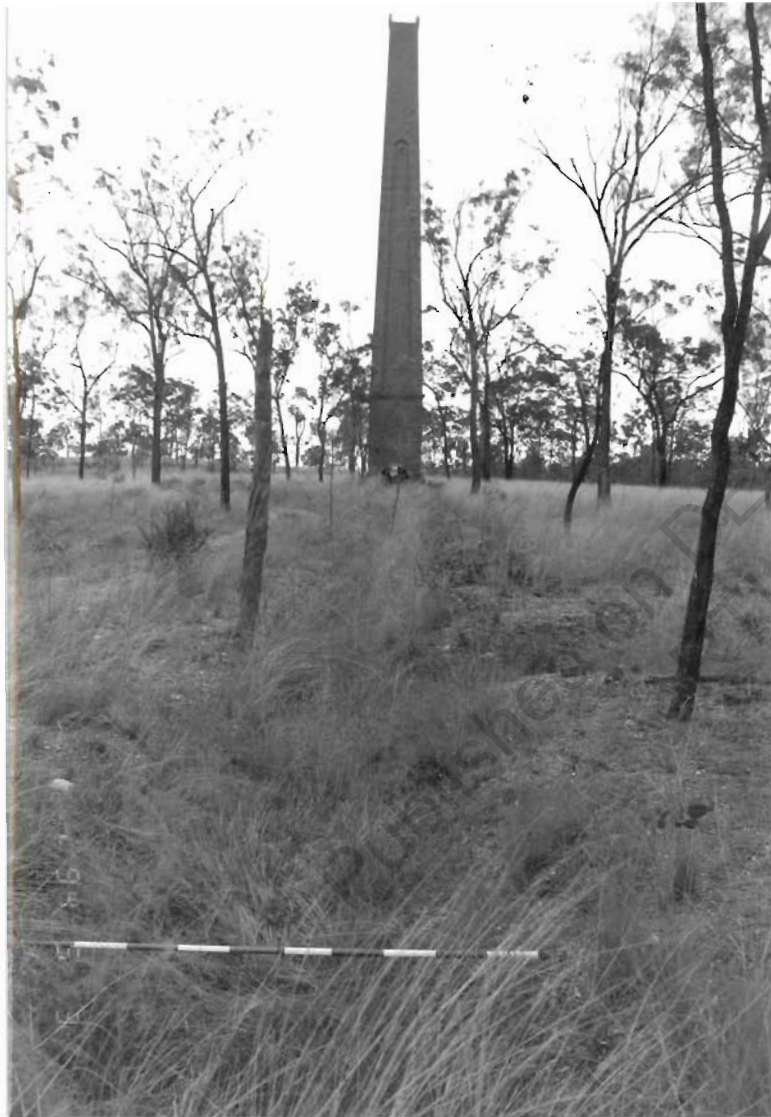
Collapsed flue (foreground) looking SW.
