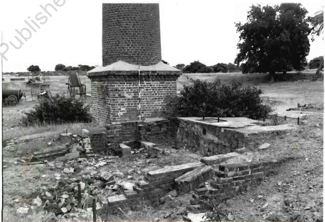
Mabel Mill: Boiler house site, showing brick flues and chimney base. Looking NW.
