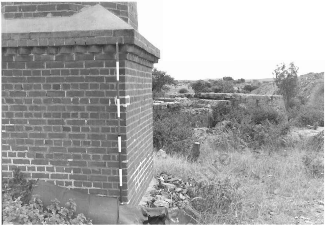
Chimney base with winding engine and air compressor foundations (background). Looking NW.
