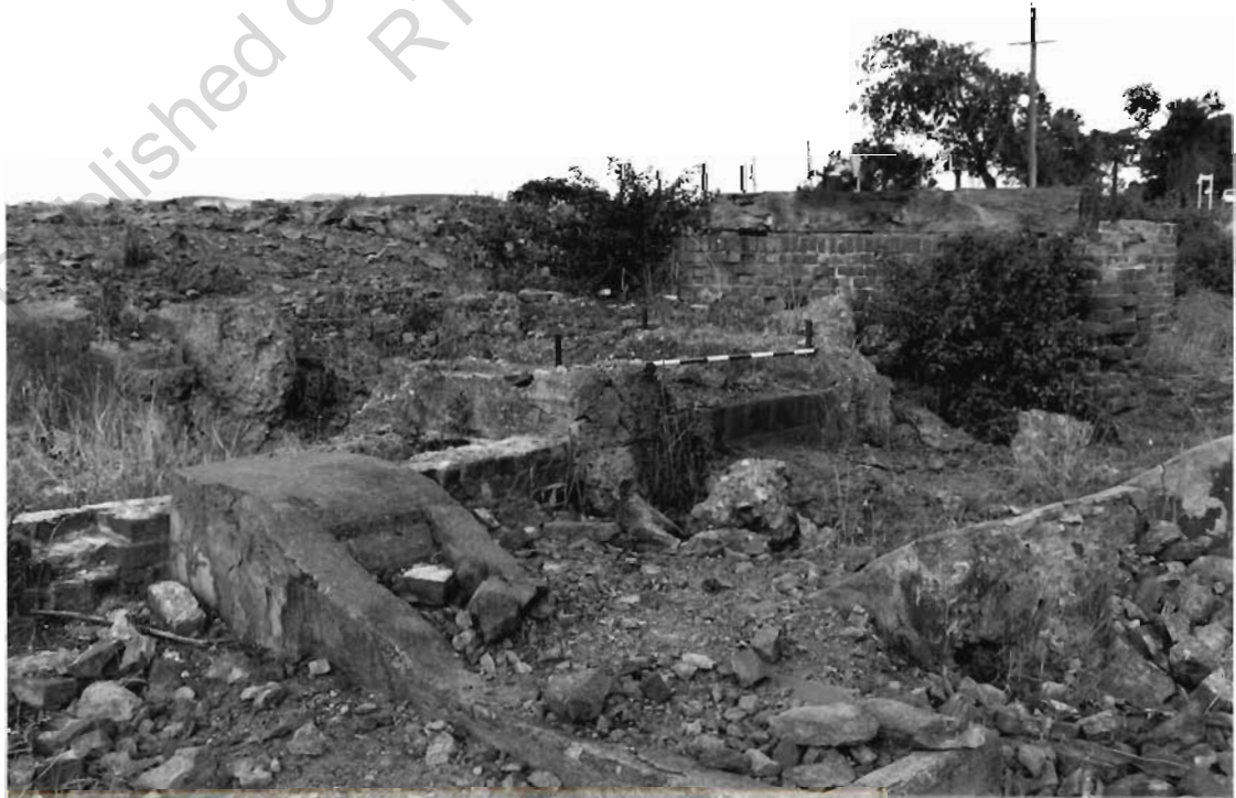
Stamp battery foundations, looking E.
