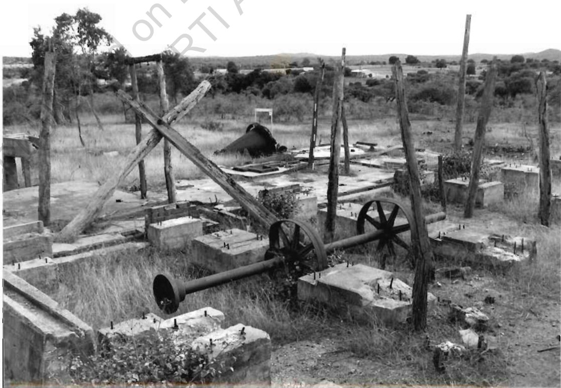
Concentrating mill foundations and timber uprights, looking N.
