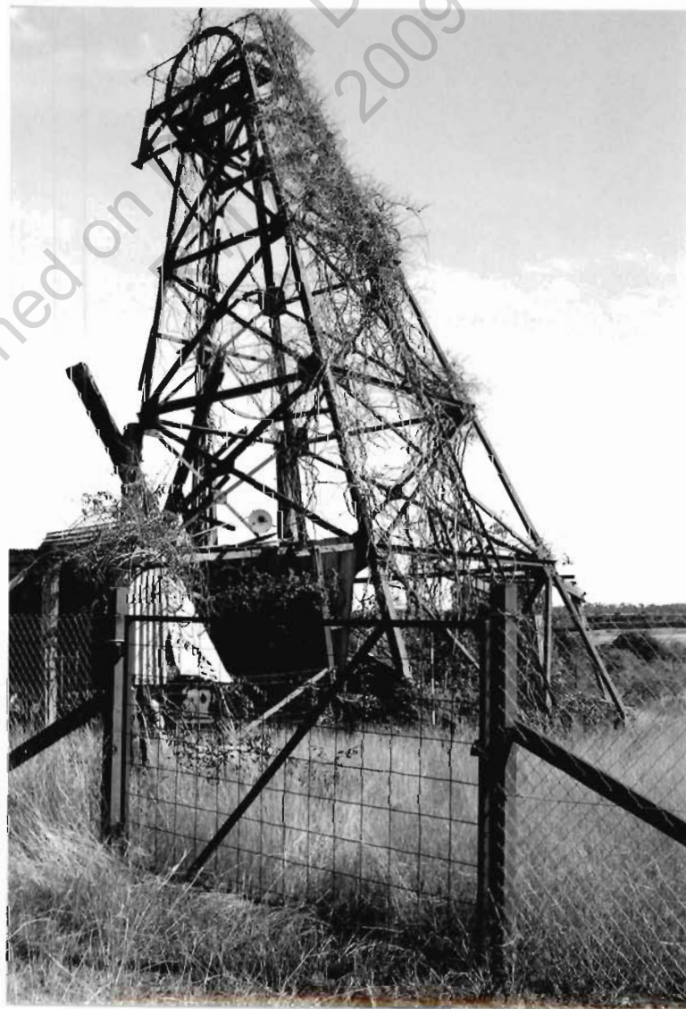
Headframe, looking NW.
