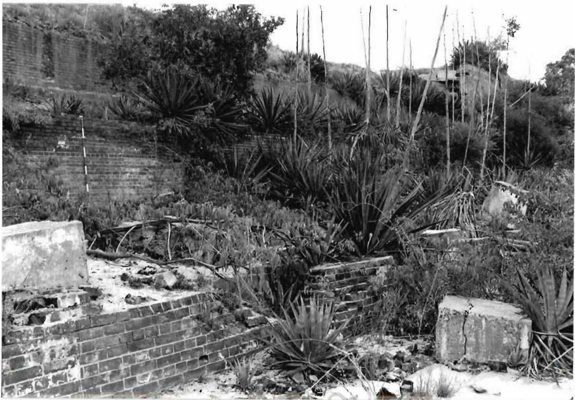
Stamp battery concrete mounts looking SE.
