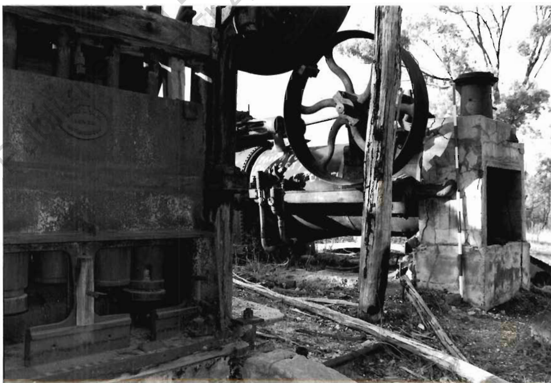
Burns & Twigg five head mortar box (left), with the portable engine in the background. Looking N.
