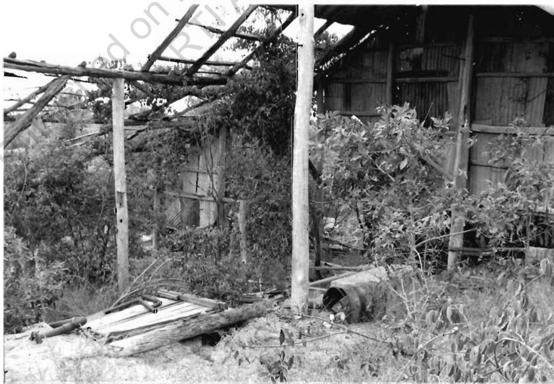
Bed log and concrete mounts for 10 head of stamps, looking N.
