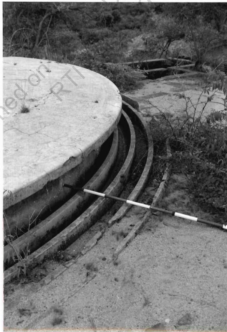
Close up of baffle bases, looking N.
