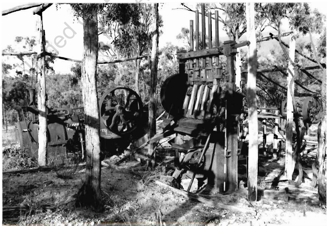
Portable engine and five head stamp battery, looking E.
