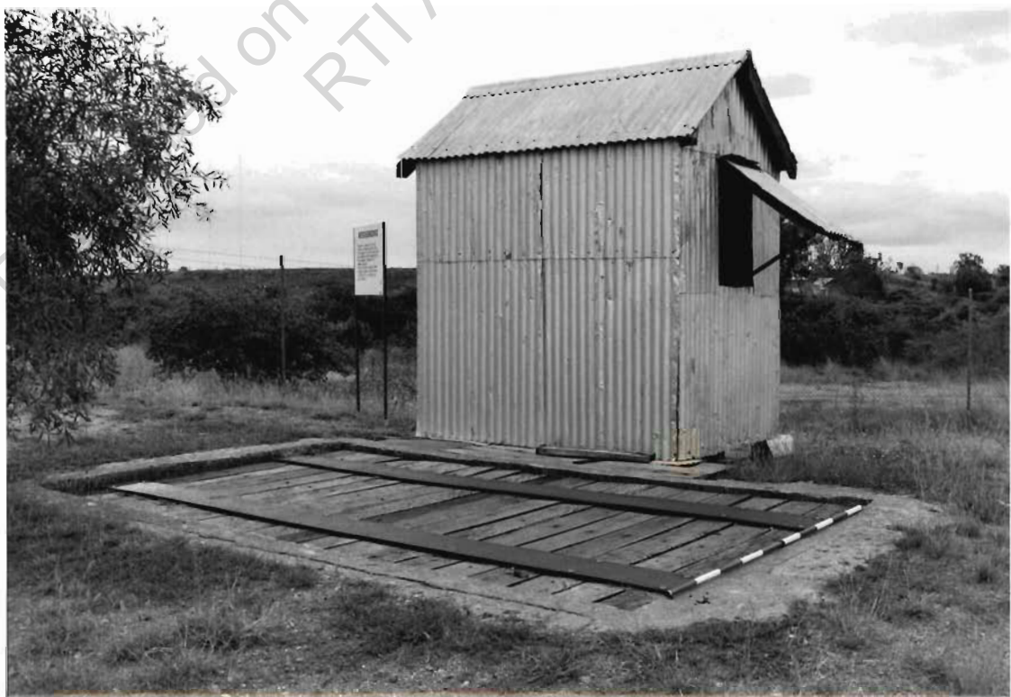
Weighbridge and office, looking NW.
