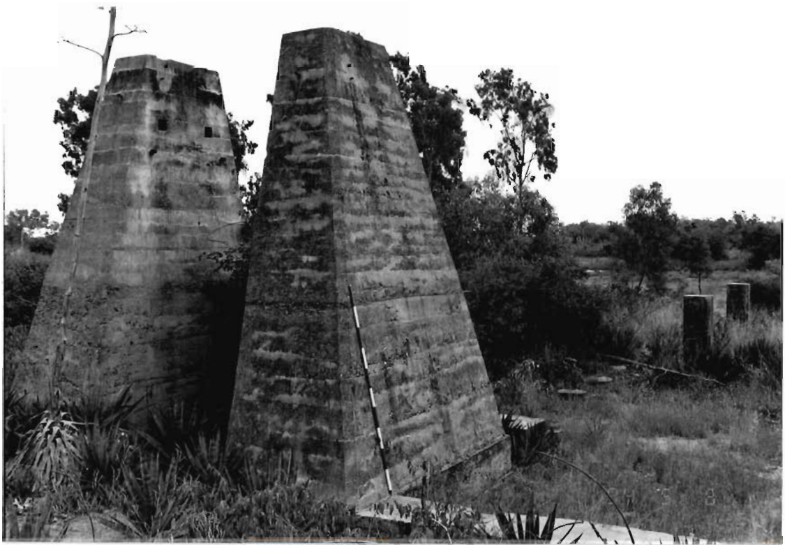
Raff wheel concrete mounts looking W.
