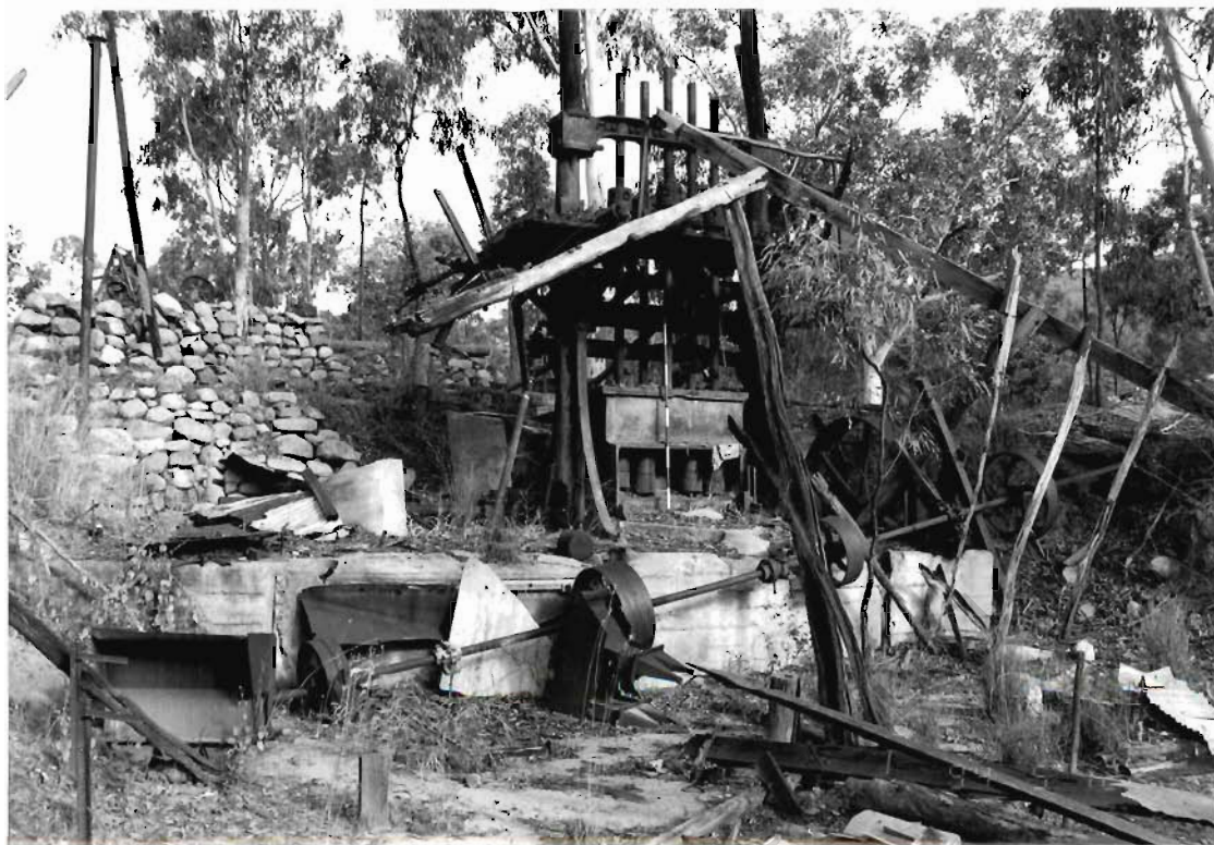
Battery and shed foundations, looking SE.
