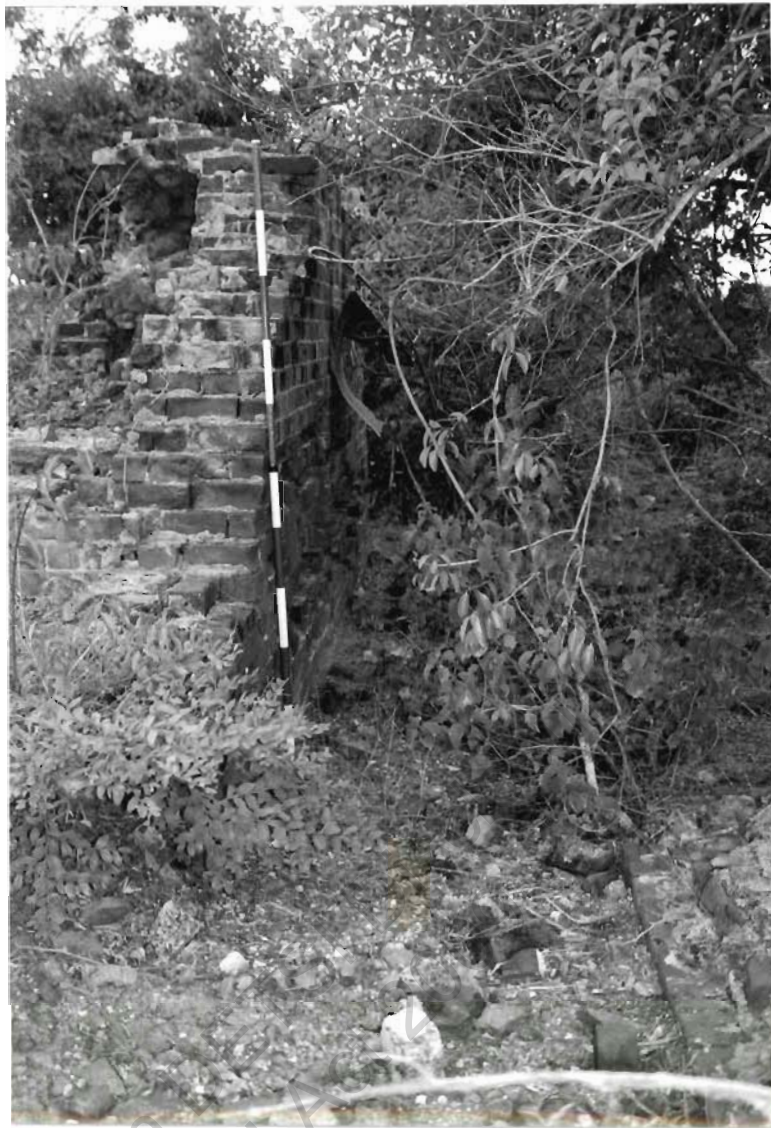
Brick mount associated with the terminus of the endless chain tramway. Looking E.
