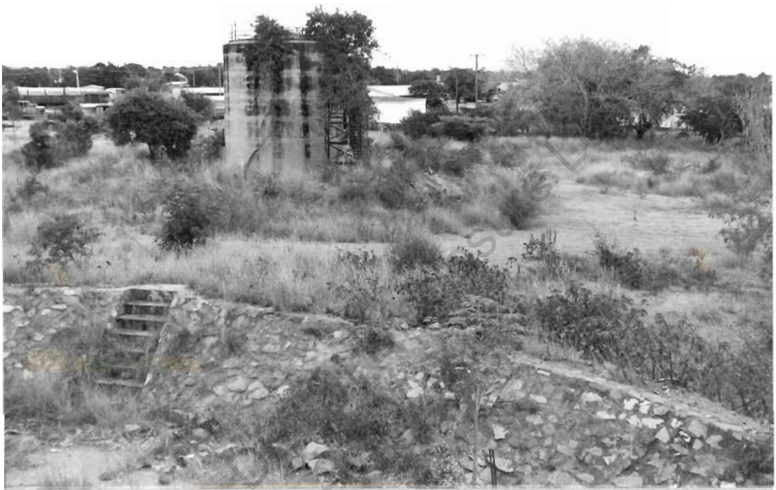
Looking over the mine site from a fuel tank. Charters Towers railway yards in the background.
