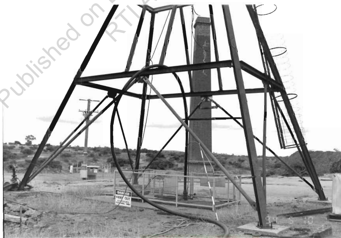
New escape shaft headframe over original shaft. Chimney in background, looking N.
