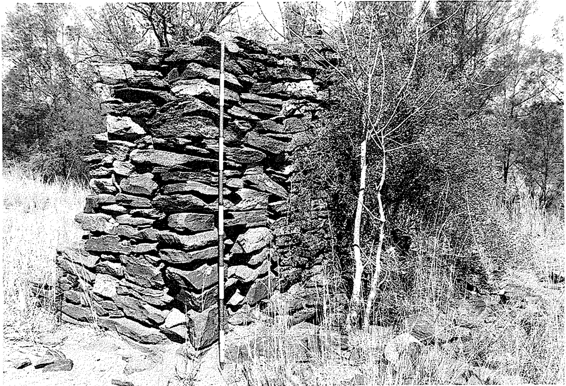
Cornish boiler flue and chimney base, looking SE.
