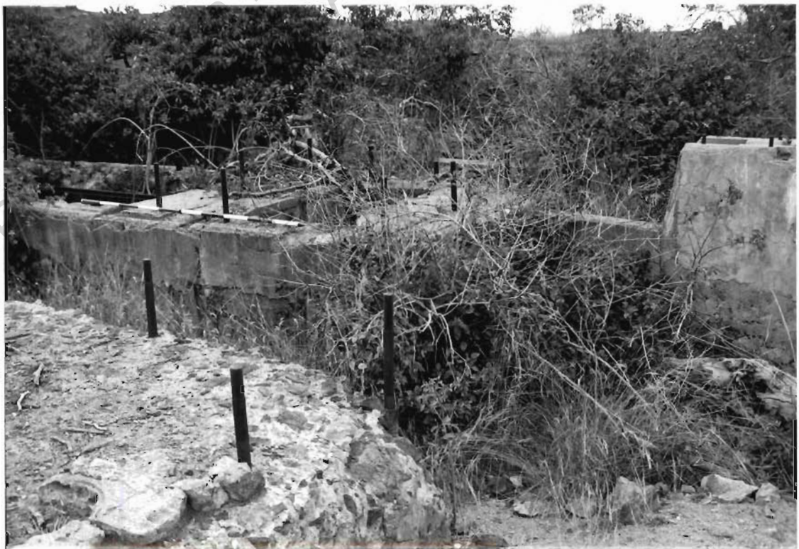
Engine mount, looking SE.
