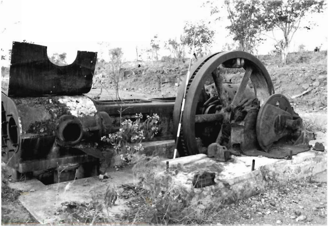
Engine house site with Ingersoll compressor, looking E.
