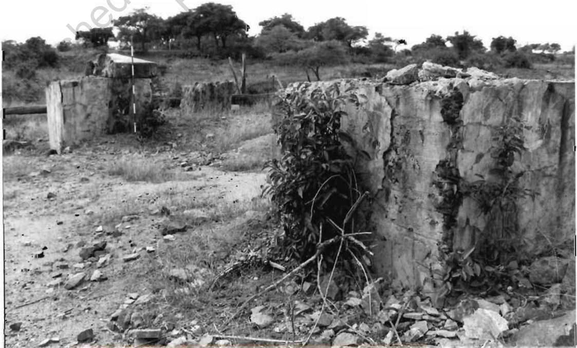
Headframe concrete foundations, looking N.
