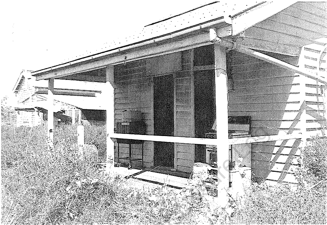
Watchhouse at rear of police station. Police cottage in the background. Looking E.
