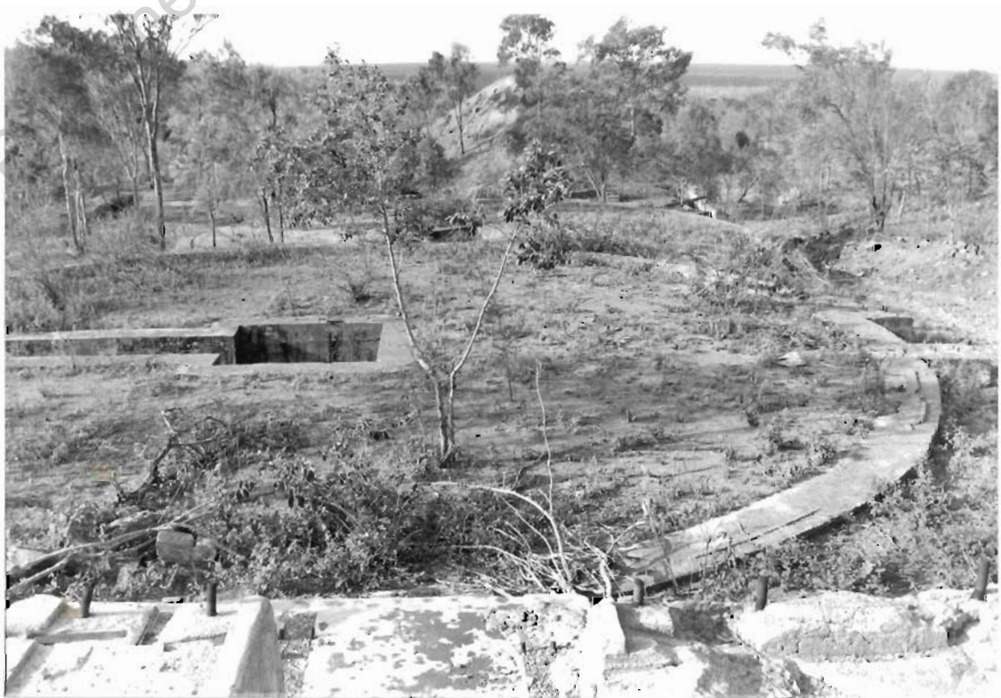
Concentrator vat concrete mounts, looking NE to main shaft and mullock dump.
