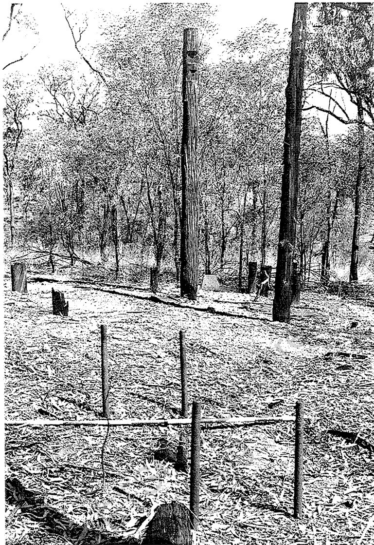
Battery east of township showing stamper frame or engine mounting rods and shed timber uprights.
