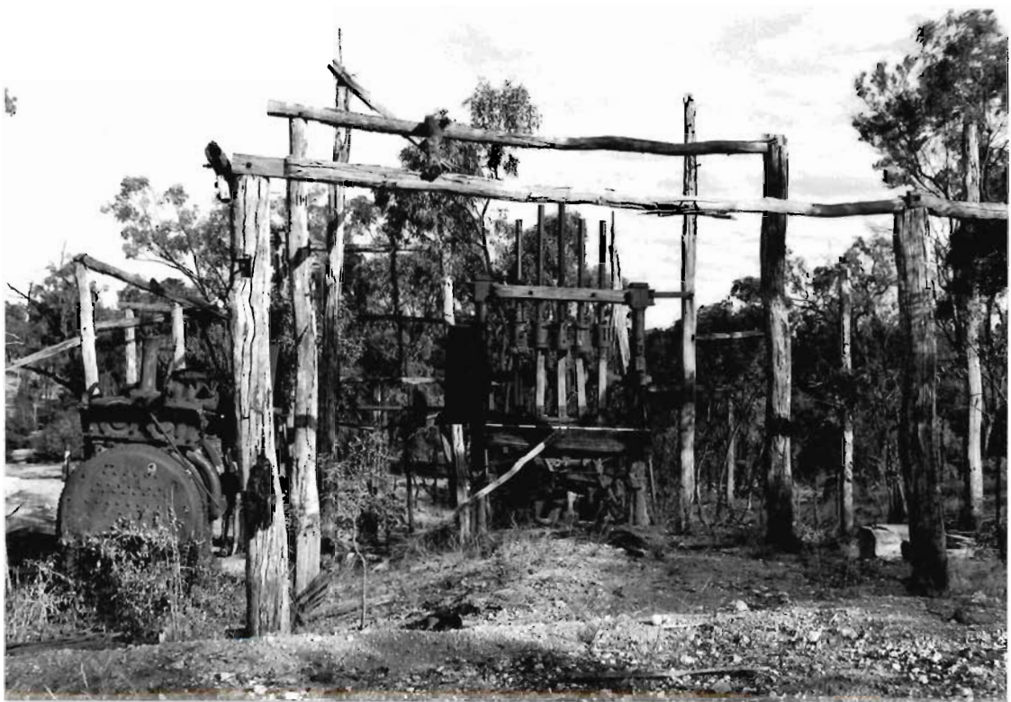
Battery shed looking SE, showing engine and stamp battery
