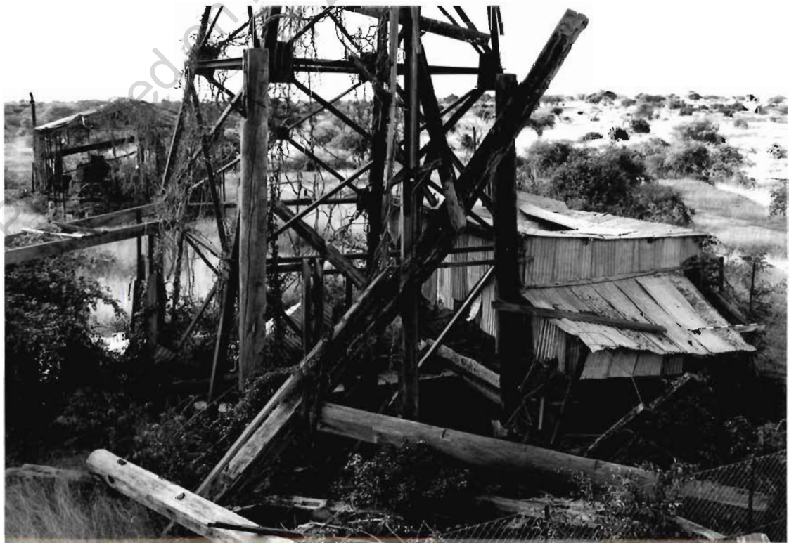
Base of headframe showing brace uprights and workshop. Winding engine shed in background. Looking E.
