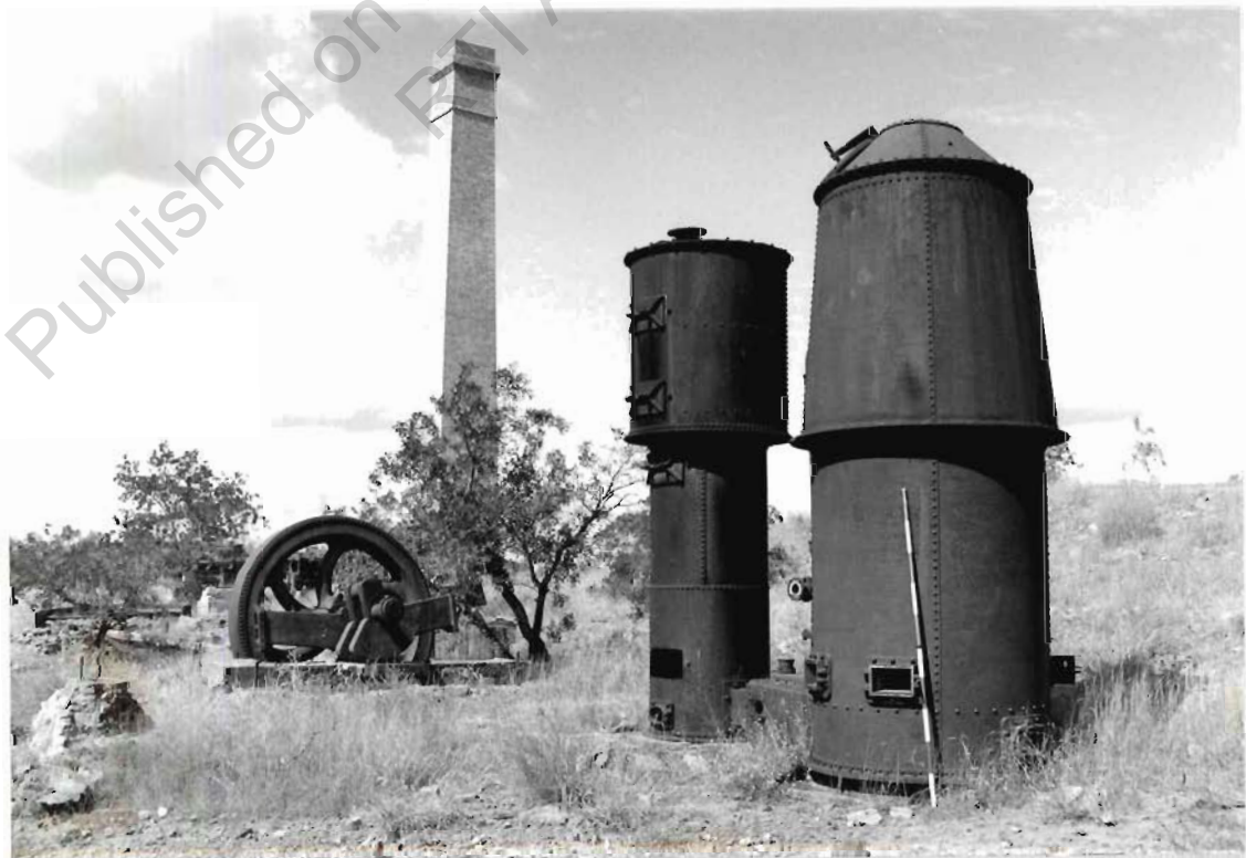
Suction gas plant looking E.
