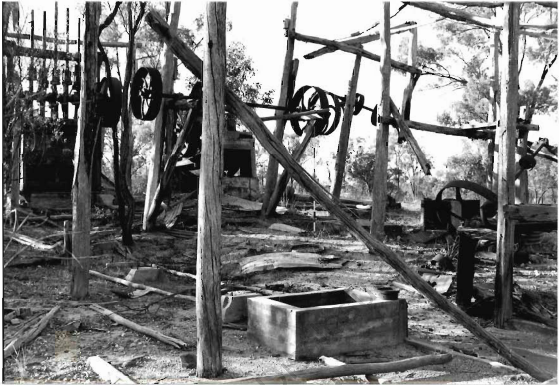
Battery shed timber uprights with the concentration plant site in the foreground. Looking N.
