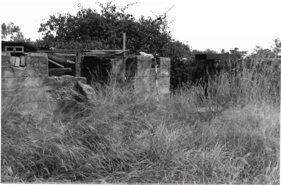
Concrete engine mounts.
