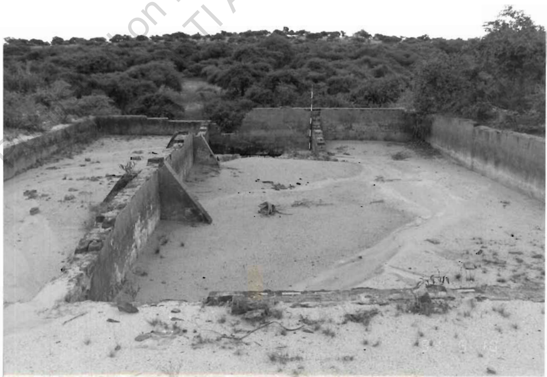
Rendered brick settling tanks, looking W.
