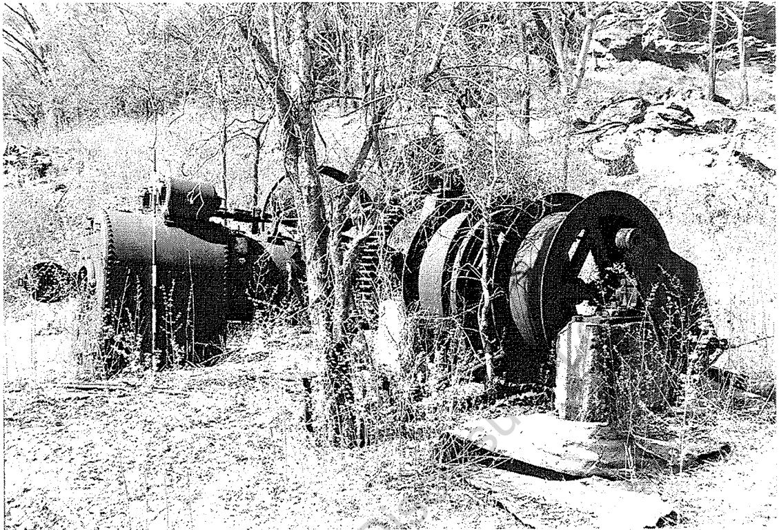
Robey 2 cyl. portable engine (left background) with a two drum winding winch (right). Looking N.
