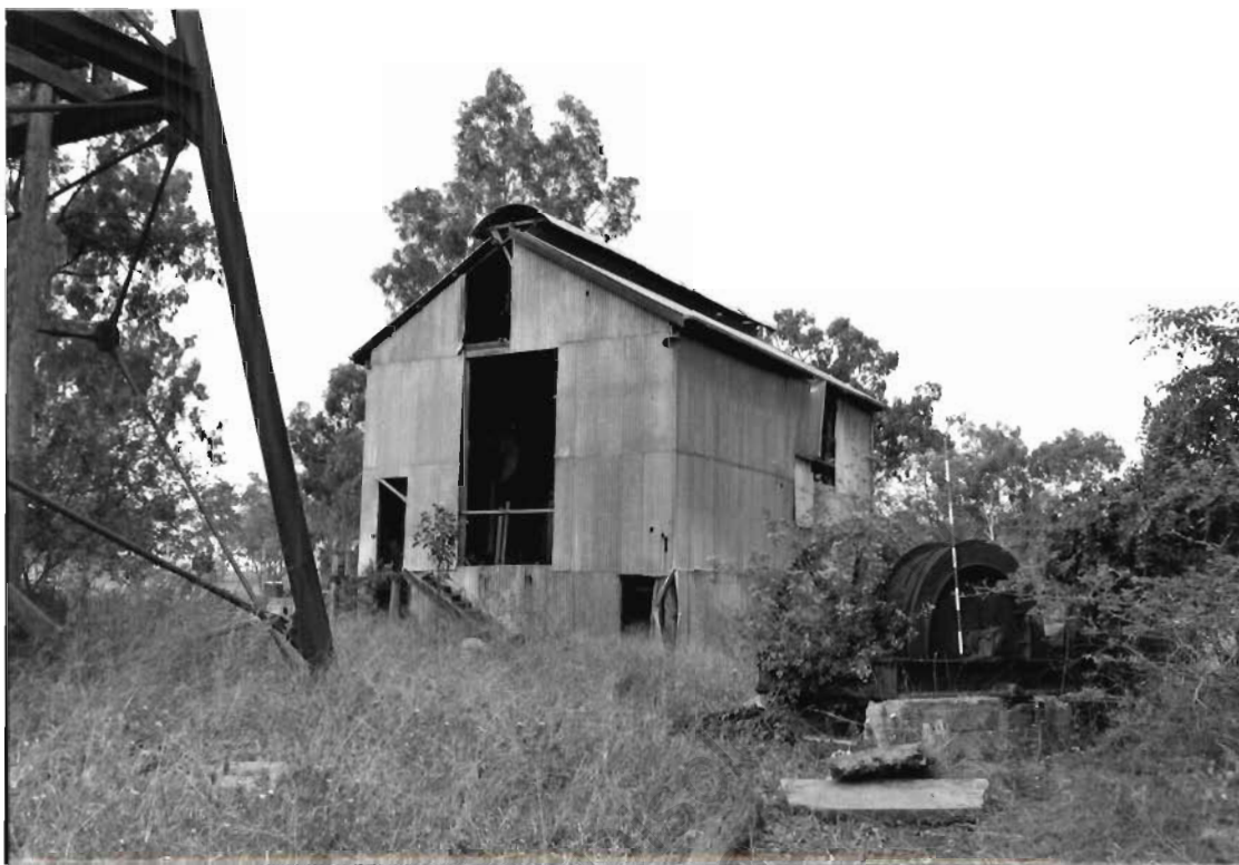
Walkers main haulage winding engine shed with headframe (right) and Hornsby winding engine (left). Looking S.
