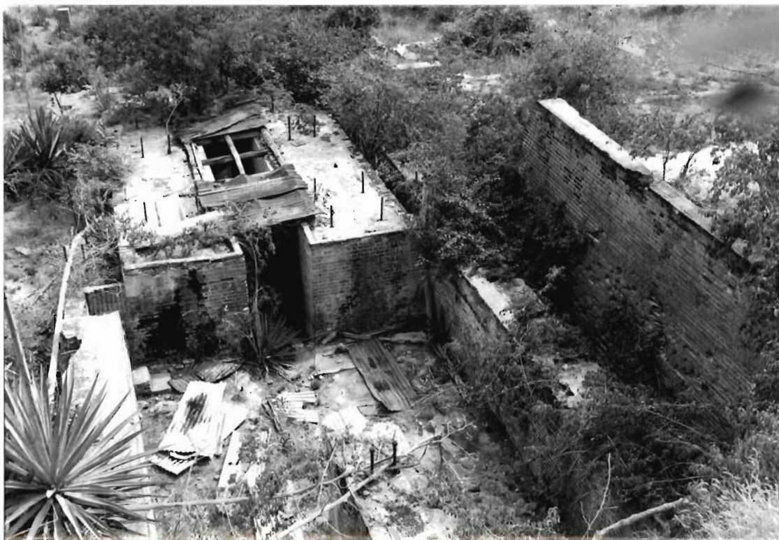
Boiler house looking W.
