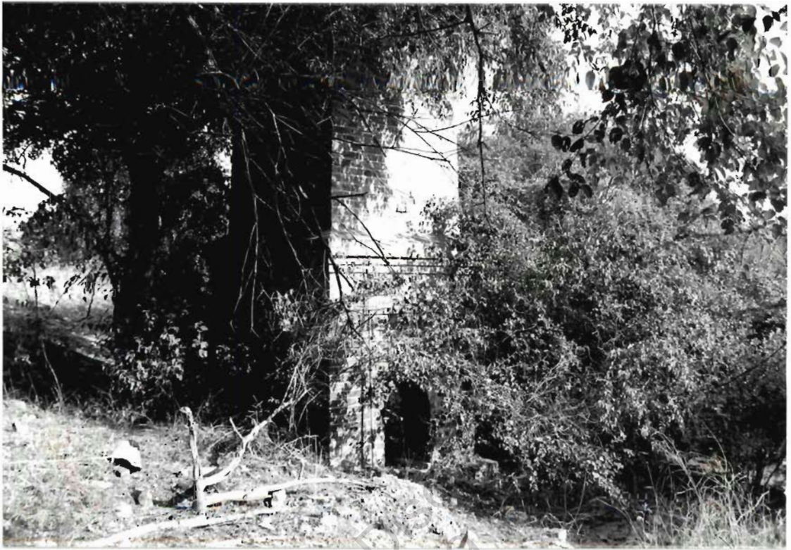
Brick chimney, looking S.
