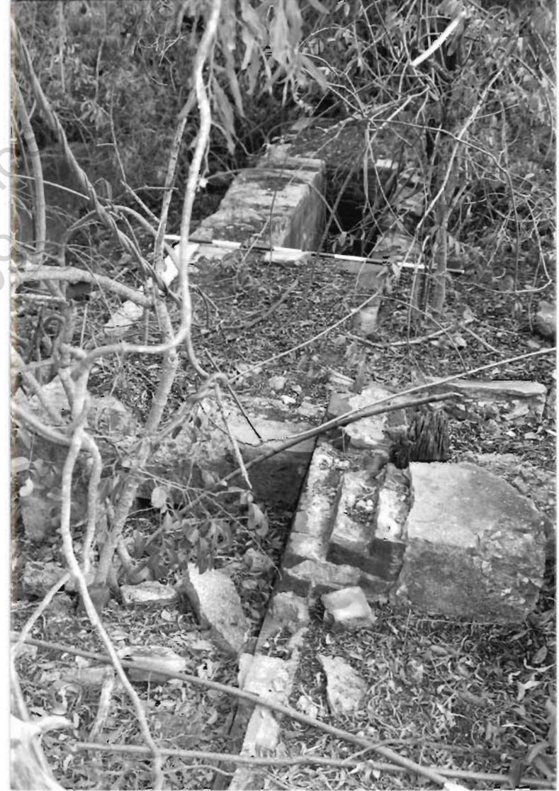
Rendered brick mill foundations.
