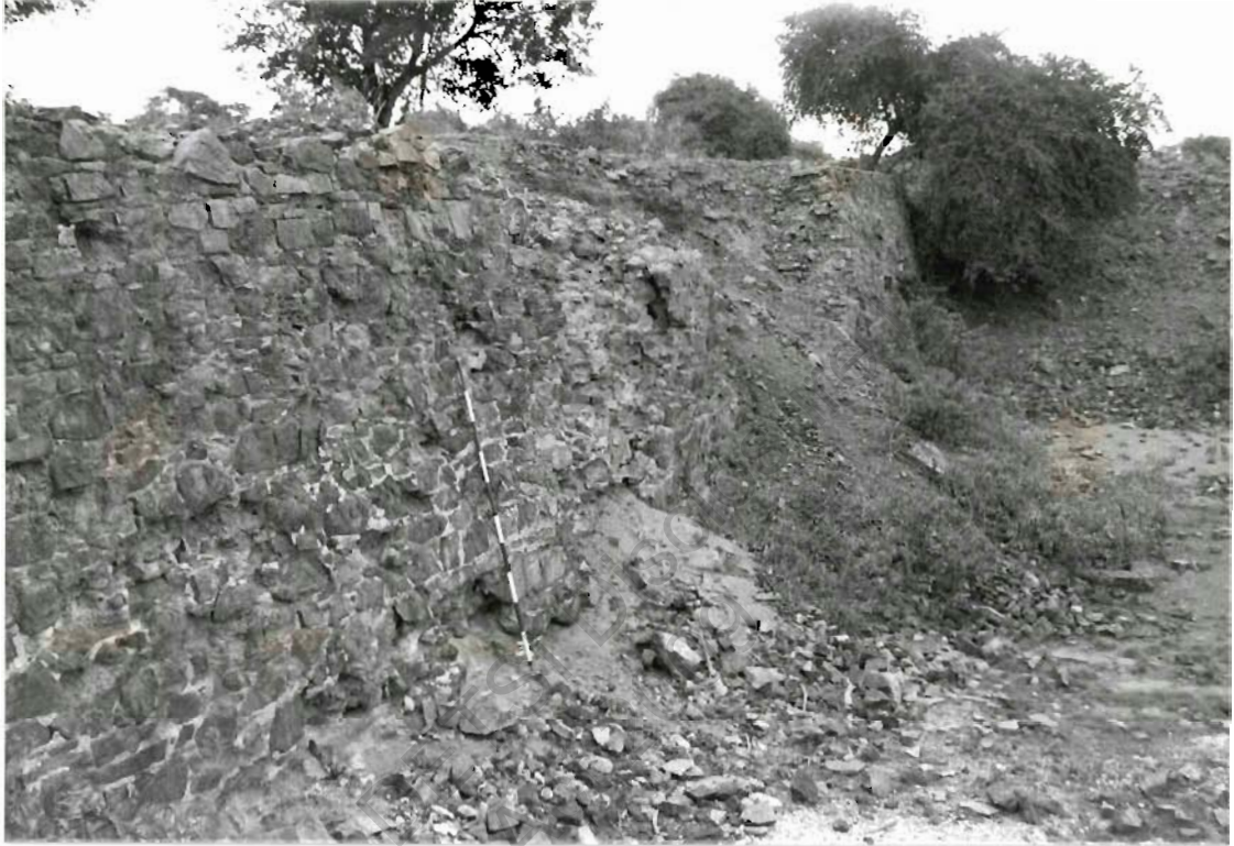
Stone retaining wall, looking S.
