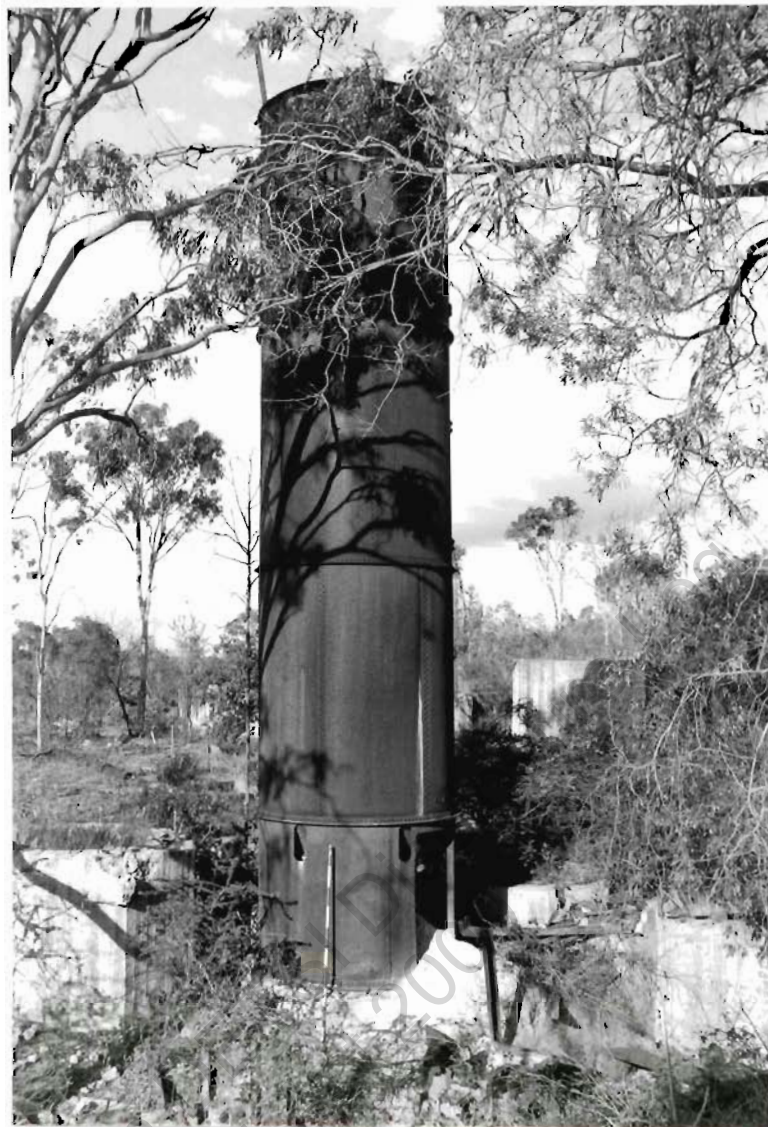
Surviving calciner tower, looking NE.
