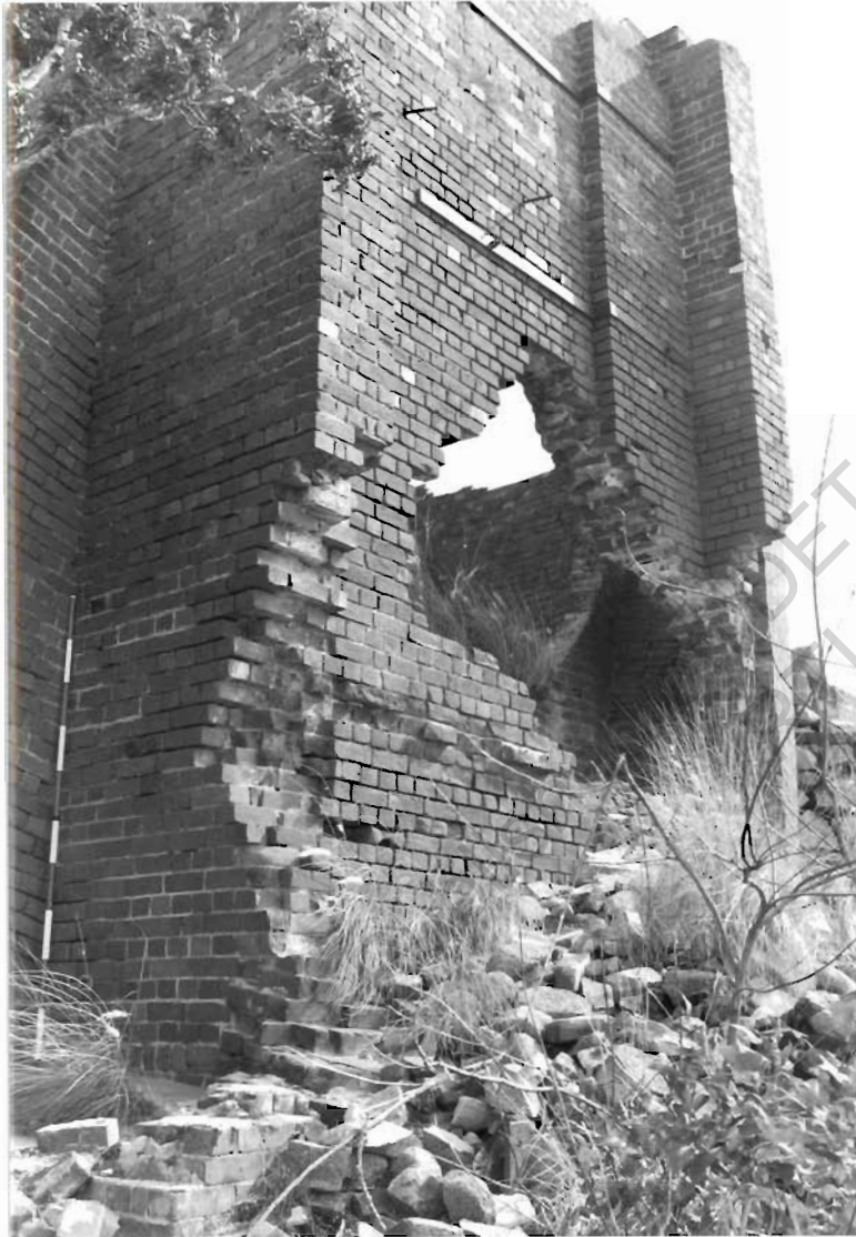
High brick bin ? Looking ]
