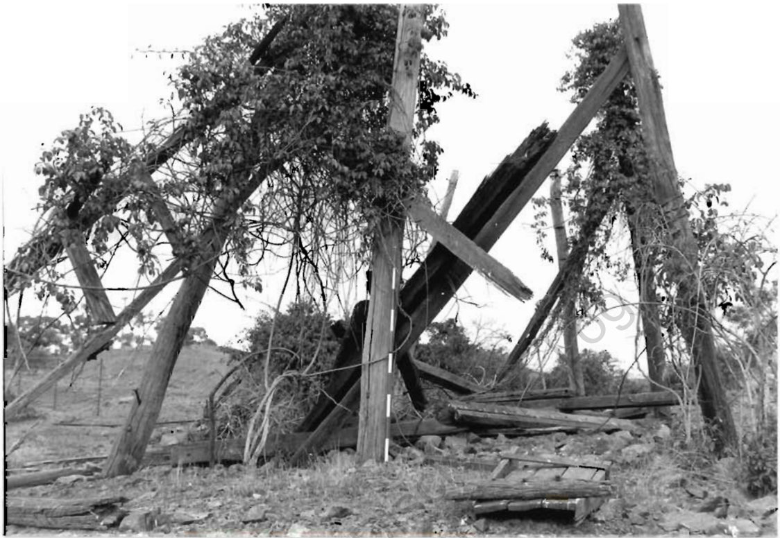
Headframe round timber uprights, looking E.
