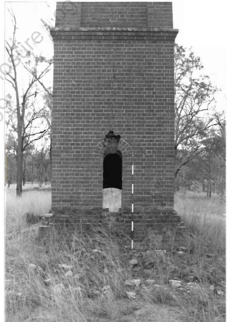
Chimney base and flue looking SW.
