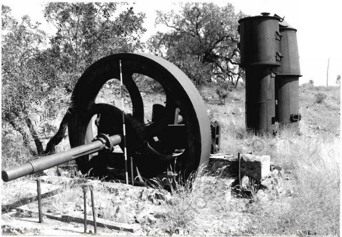
Crossley gas engine (foreground) and gas producer looking SW.
