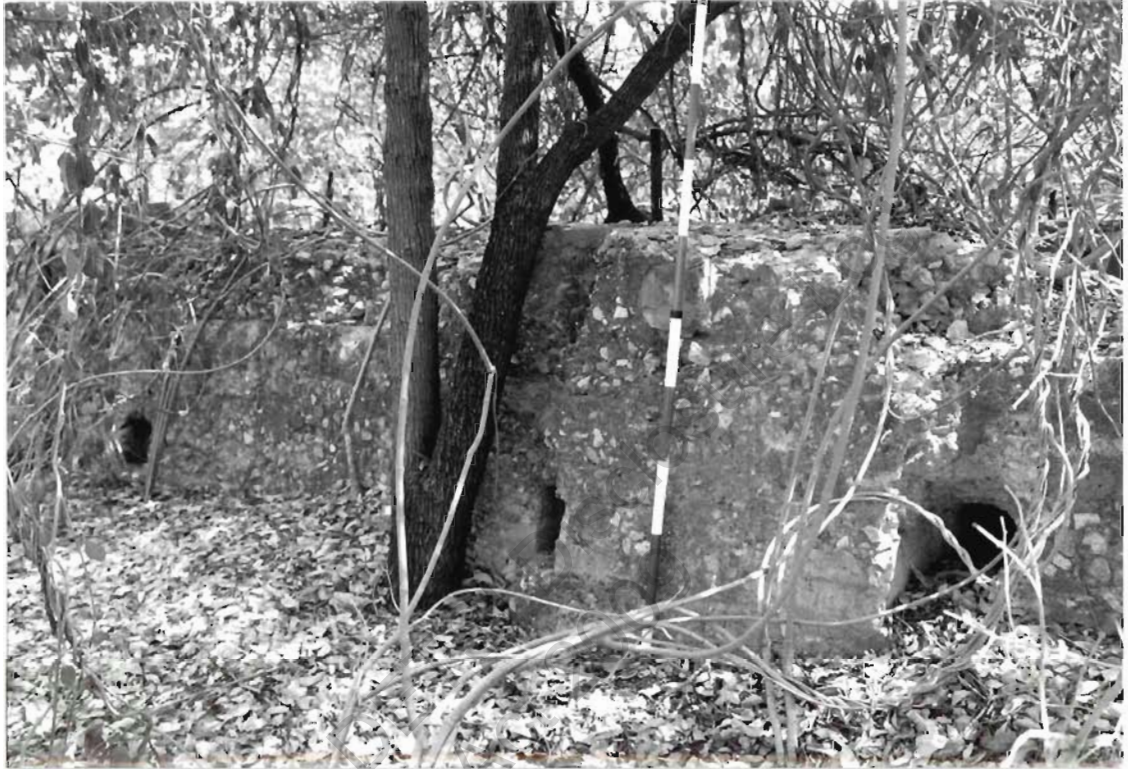
Dam stone retaining wall, looking NE.
