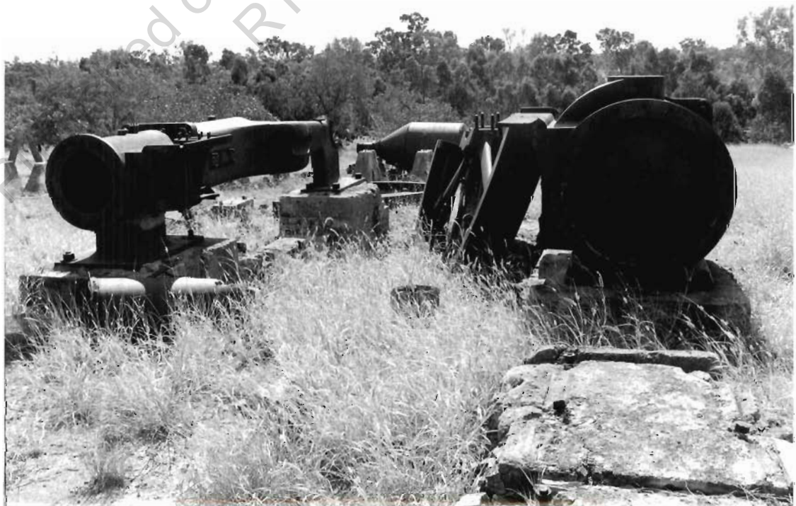
Cross compound gas engine sections looking N.
