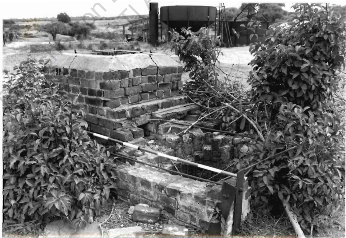
Mabel Mill: Assay office foundations near the Partridge and Ralston mill. Looking W.
