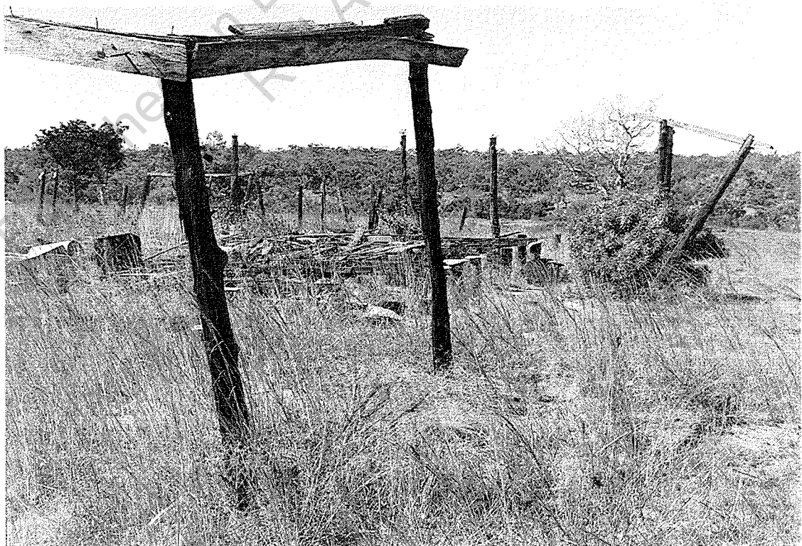
Timber stumps and uprights at the southern end of Parallel Street. Thought to be a former hotel site.
