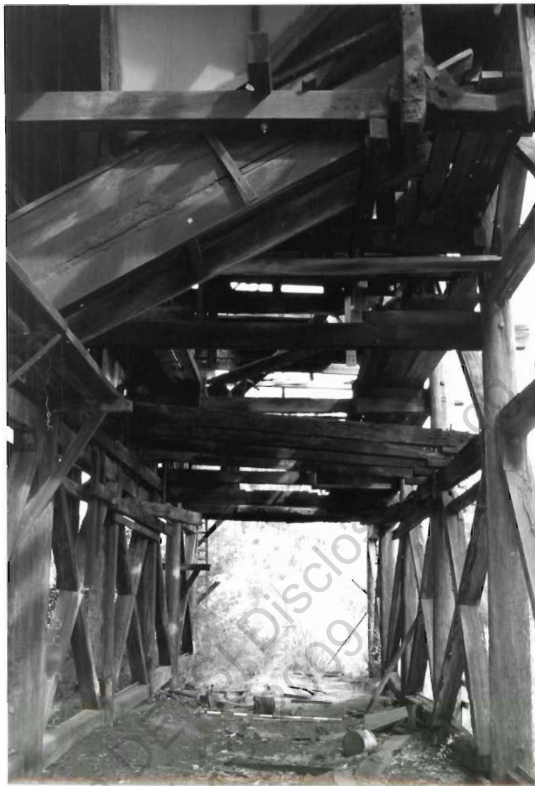
Gantry over the coal loading siding with bins and chutes above. Looking W.
