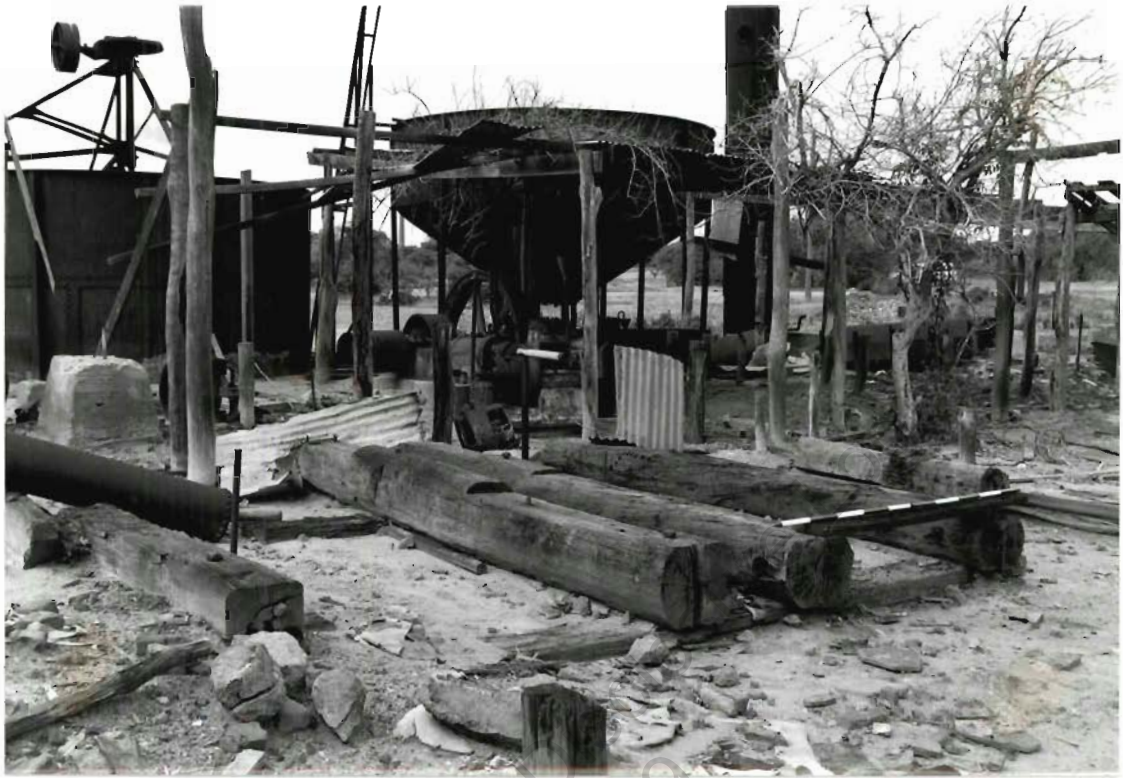
Partridge mill: Engine mount bed logs in foreground, looking SE.
