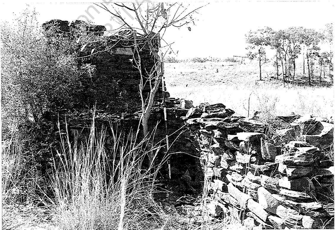
Cornish boiler stone mount and flue, looking N. to the township site.
