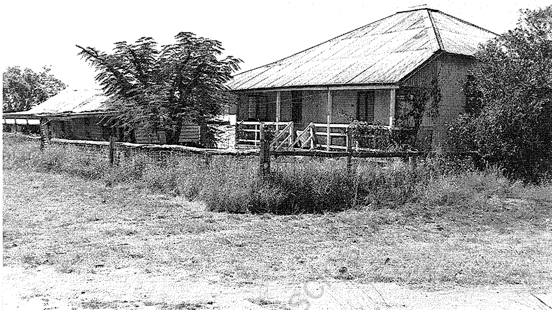
Police house (foreground), with Kidston police station alongside (left). Looking NE.
