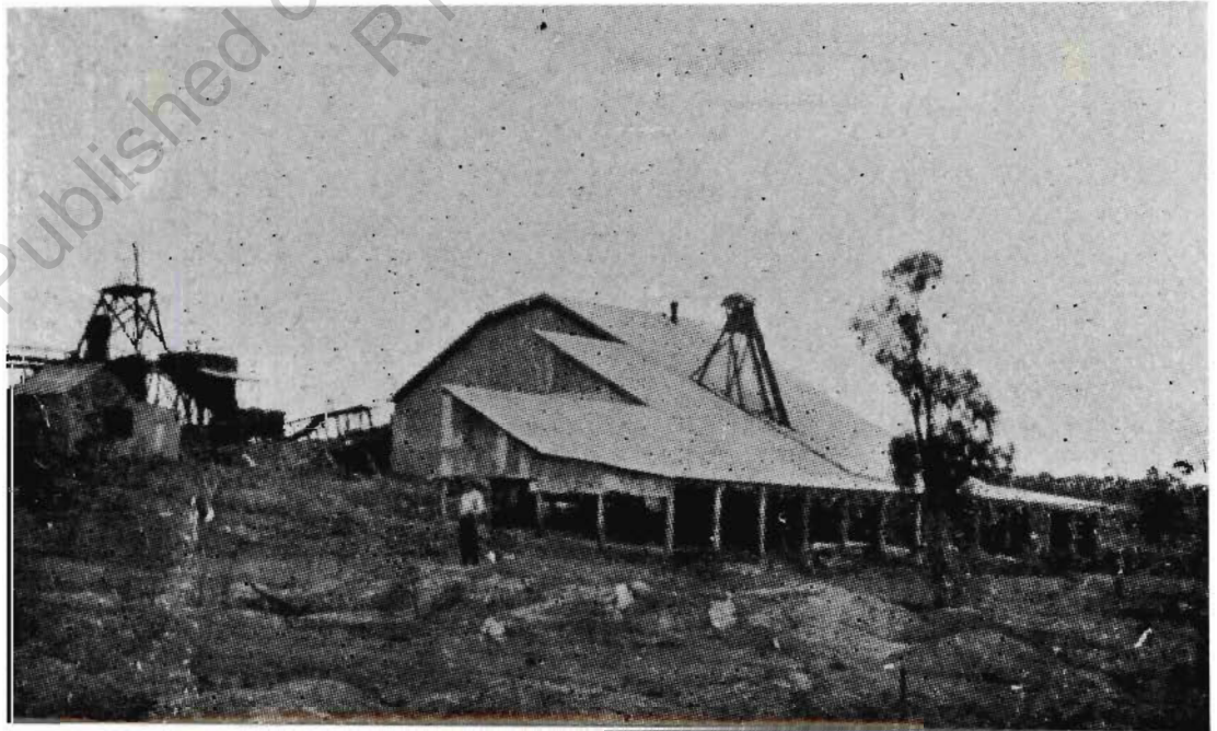
Carrington Lion P.C. showing main shaft (left) and battery (foreground). Q.G.M.J. 14 June 1919, p.238.
