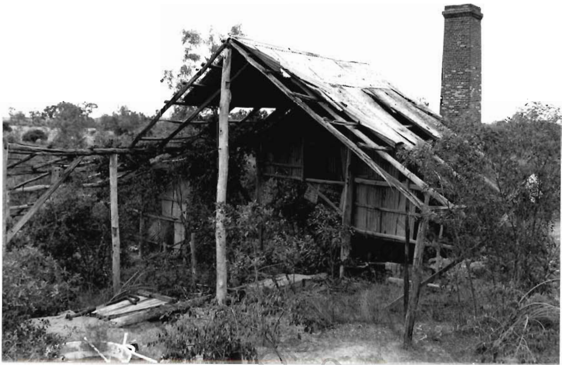
Battery shed and chimney, looking N.
