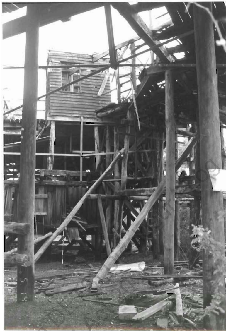
Fire damaged gantry showing the weighbridge office. Looking N.
