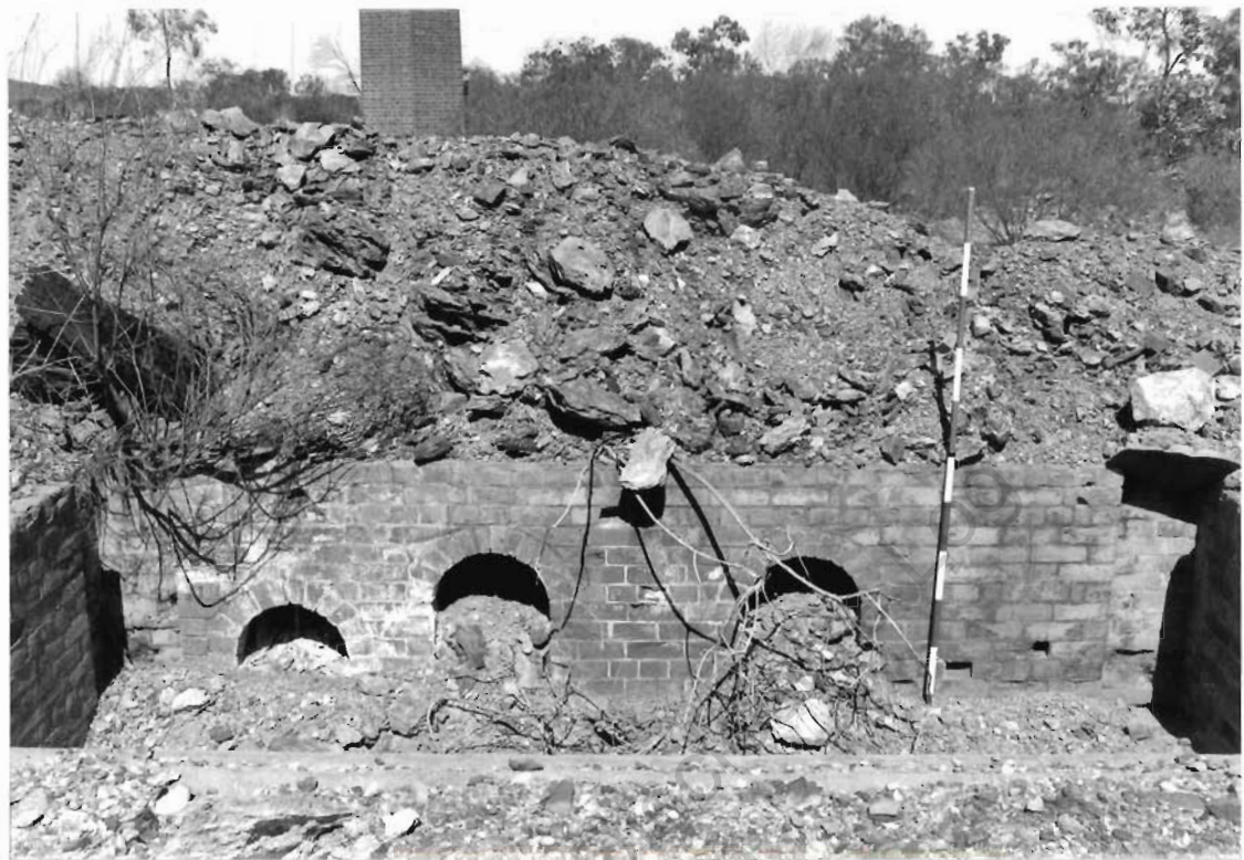
Brick lined pit and tunnels looking SW.
