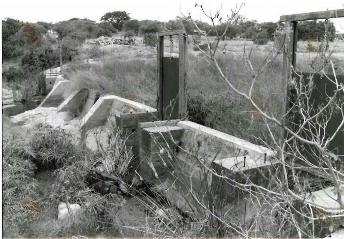
Gladstone Creek weir, looking SE.
