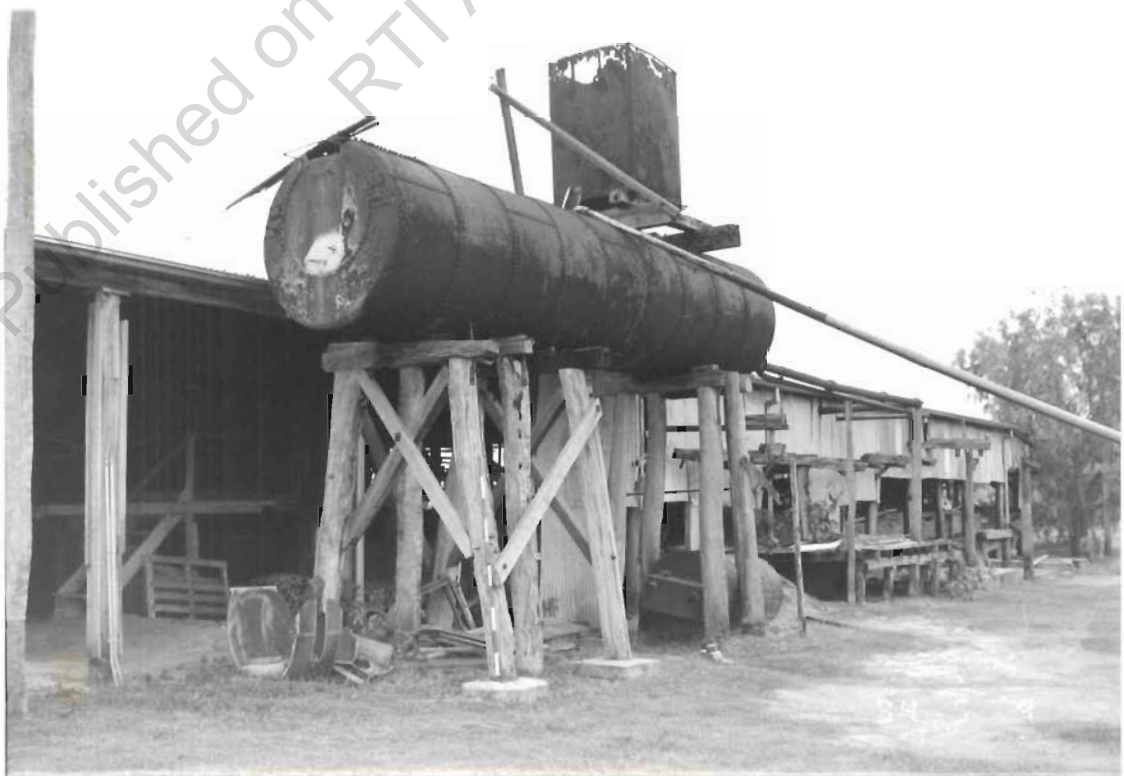
Cornish boiler adapted as a water tank, looking S.
