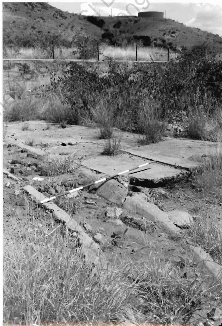
Concrete surfaces and laundry, looking W to Towers Hill.
