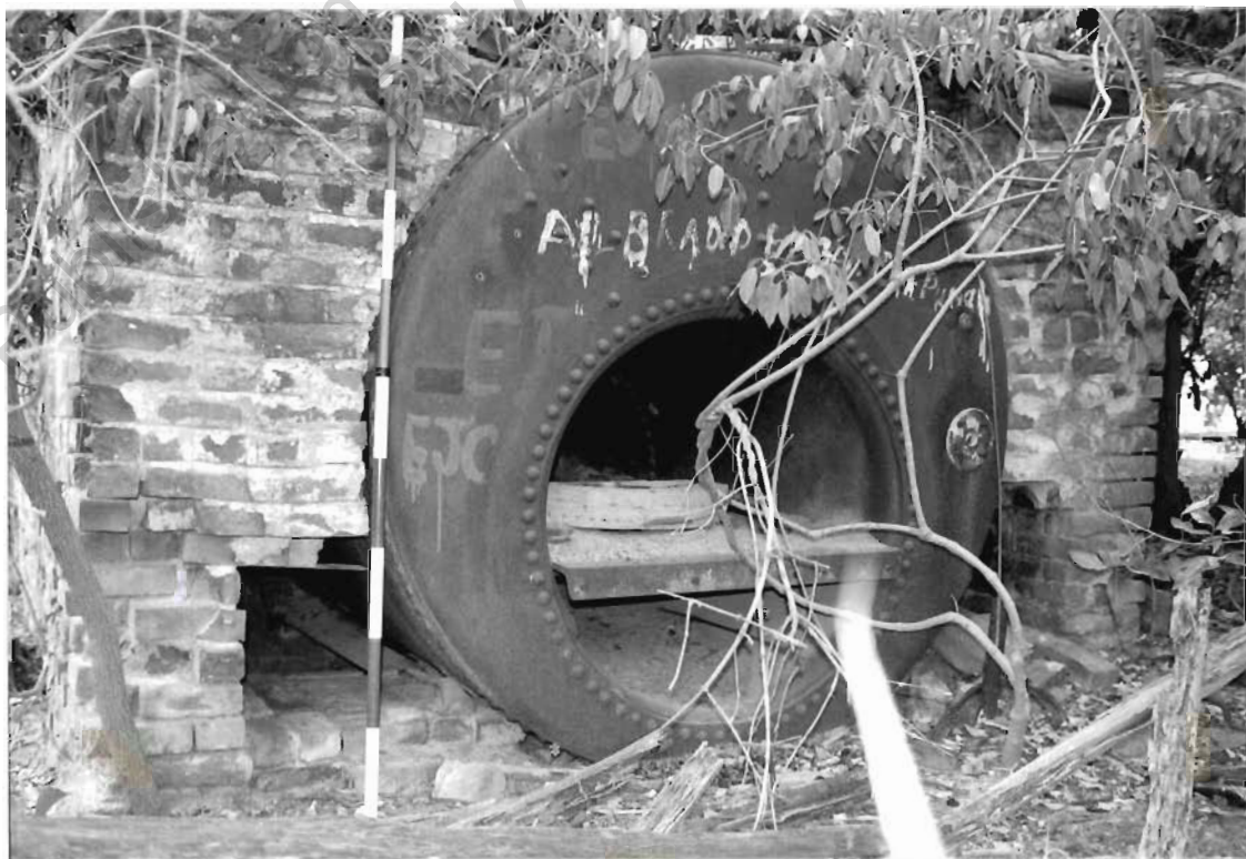
Cornish boiler and brick mount, looking NE.
