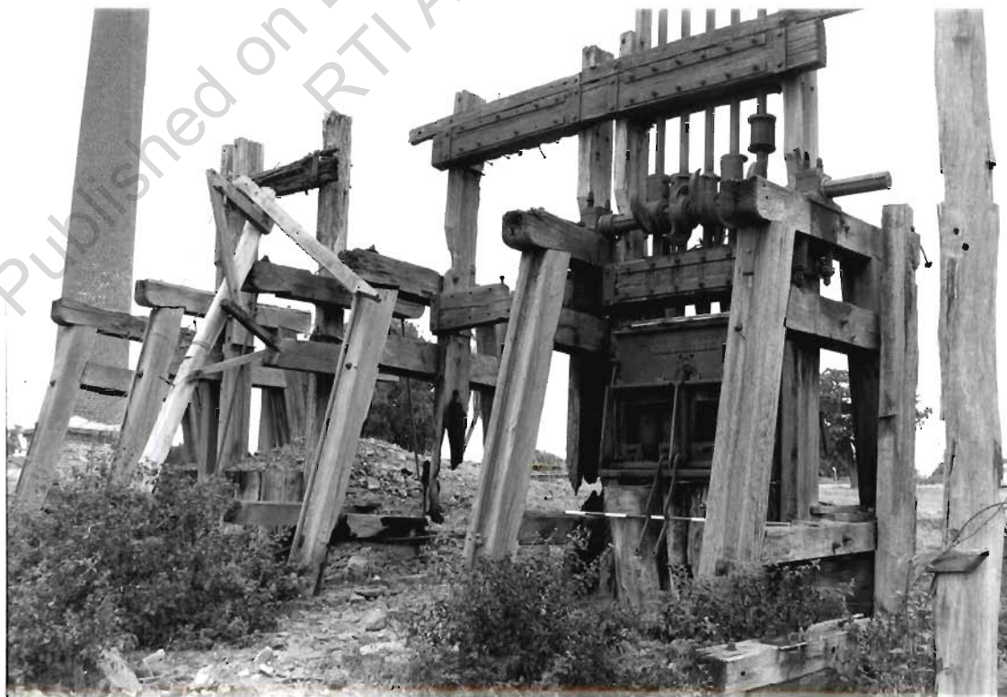
Mabel Mill: Stamp battery timber frames showing surviving five head of stamps (right). Looking NW.
