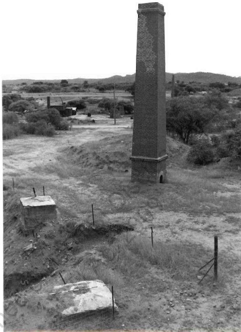
Grand Junction Consols chimney with headframe concrete mounts in foreground. Looking NW towards Partridge's mill.
