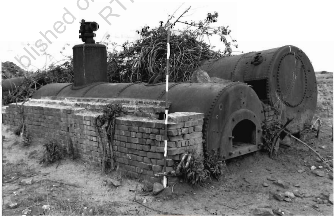
Cornish boiler with Cornish boiler adapted as a water tank on right. Looking SE.
