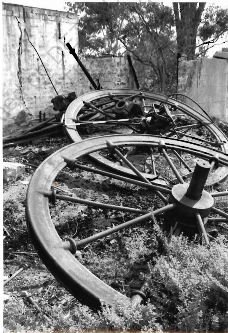
Headframe sheave wheels from the fire damaged No.2 (Horse) shaft. Looking N.
