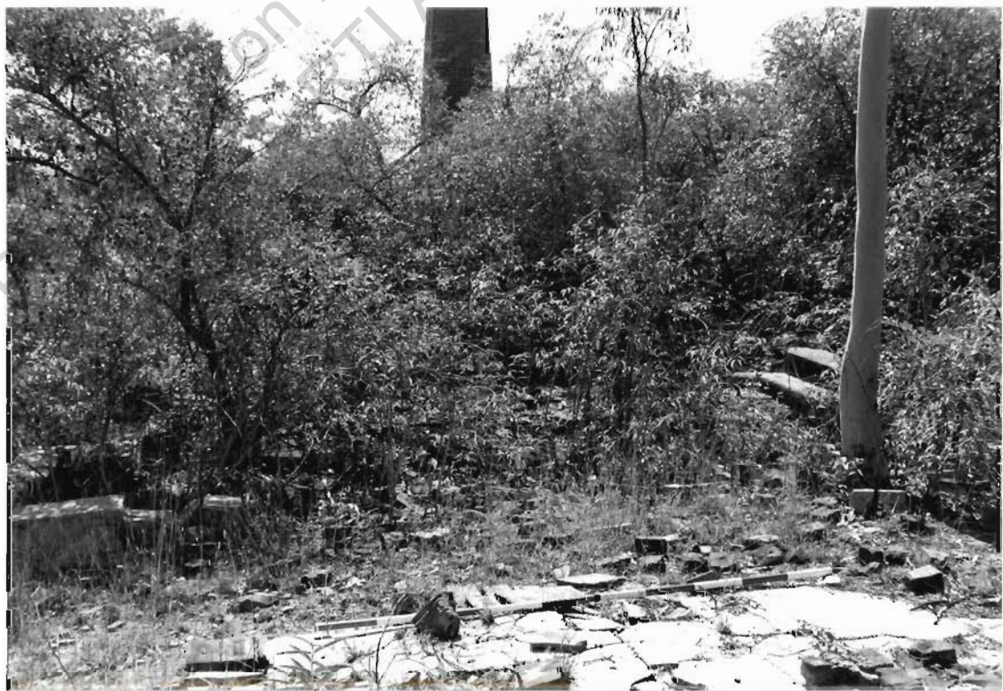
Mill foundations, looking N.
