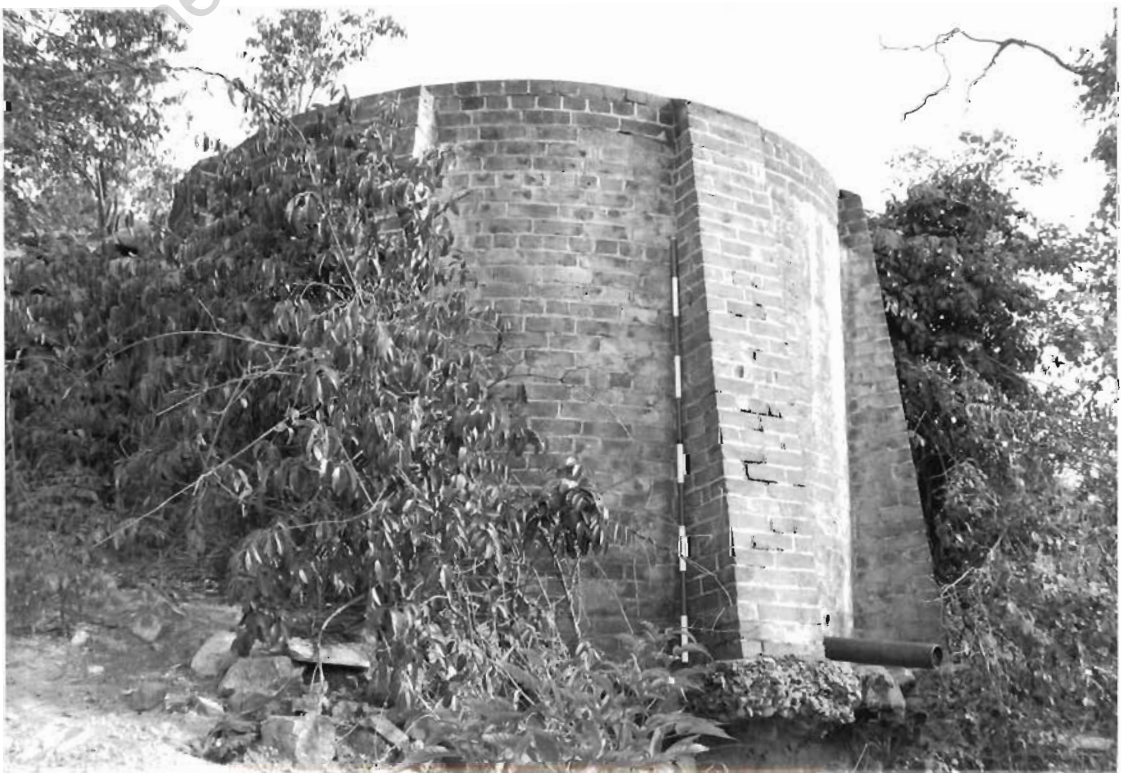
Chlorine tank ? Looking NW.
