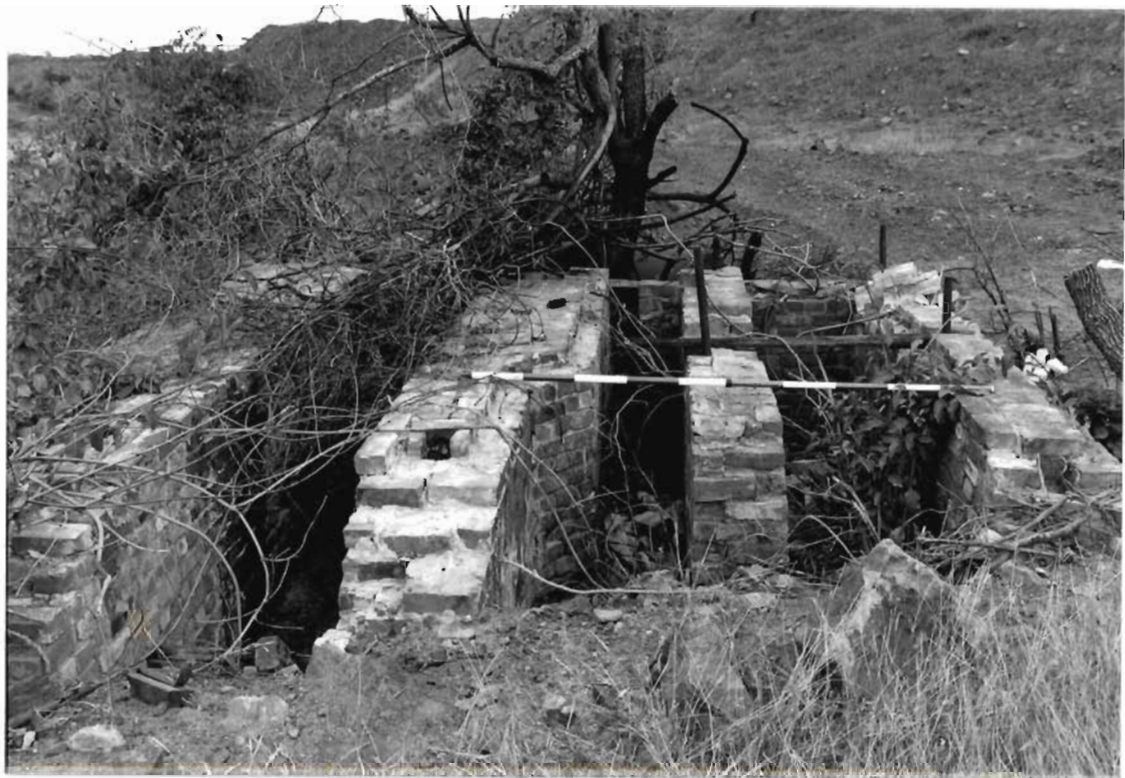
Winding engine brick mounts, looking NE.
