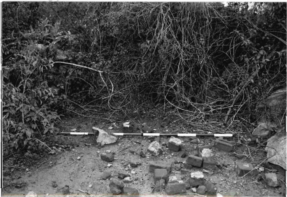
Formation of endless chain tramway under Birkby Street, Totley. Stone abutments on each side. Looking E.
