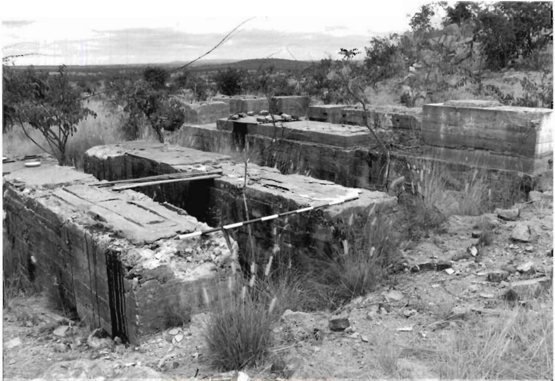
Engine house, concrete machinery mounts looking SW.
