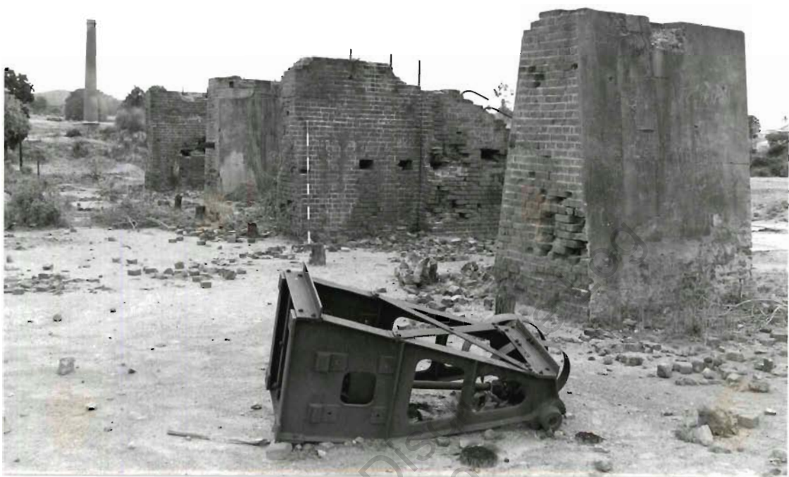
Mabel Mill cyanide plant site - high brick mounts. Looking NE.
