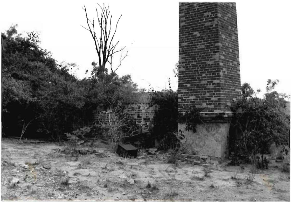
Cornish boiler brick mount and chimney, looking SW.
