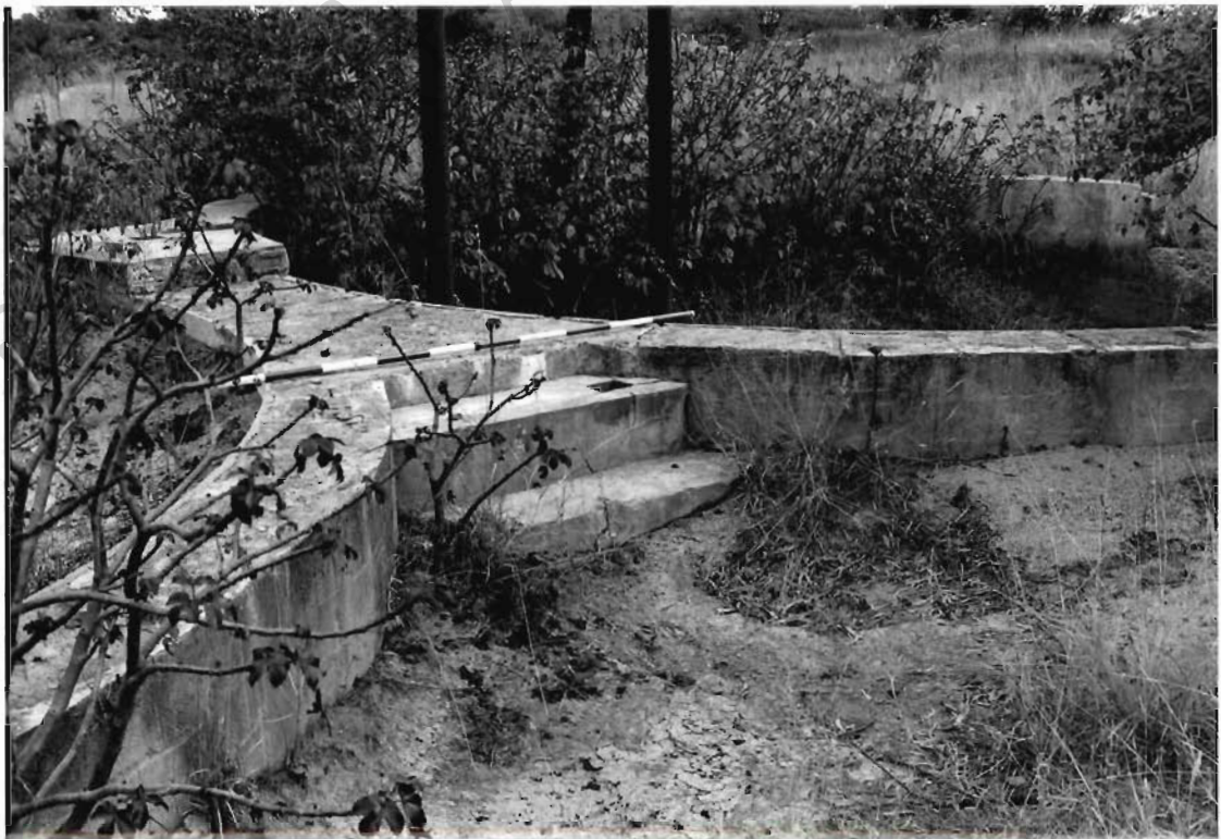
Cyanide vat concrete bases looking S.
