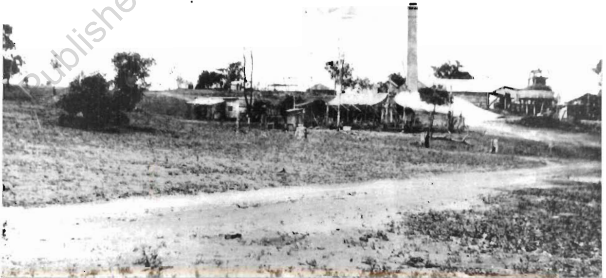
Barclay's battery: Mount Coolon Gold Mines. Queenslander. 2 June 1932. (John Oxley Library No.109691)
