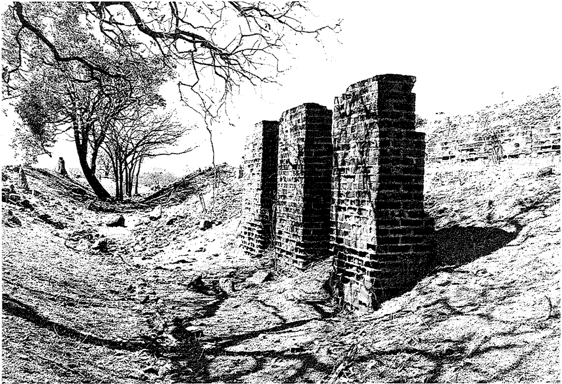
Tramway formation showing brick piers and retaining wall alongside Nil Desperandum mine.
