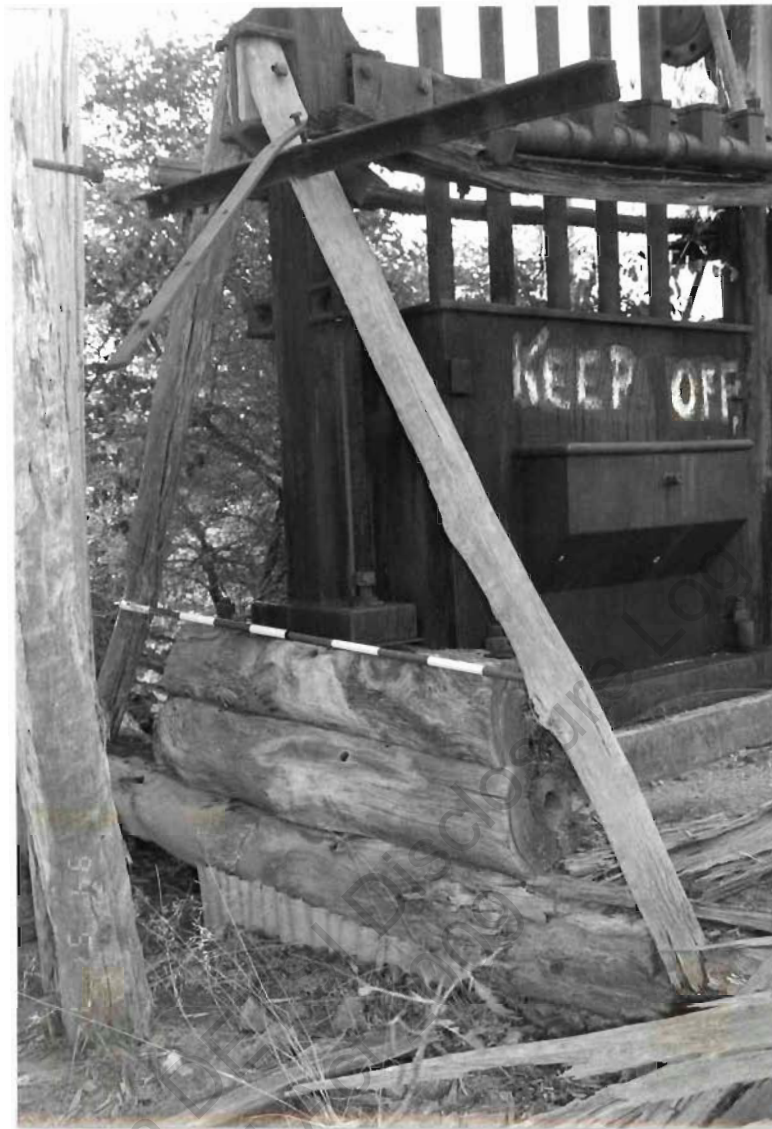
Stacked bed log battery mount with Walkers mortar box. Looking NW.
