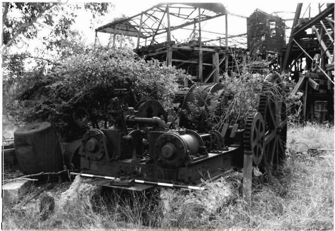
Hornsby winding engine. Looking NE with headframe, gantry and weighbridge office in background.
