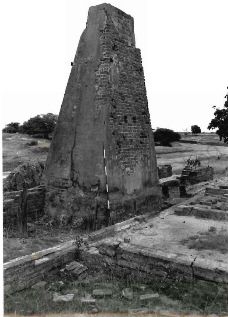
Rendered brick raff wheel mount, looking SW.
