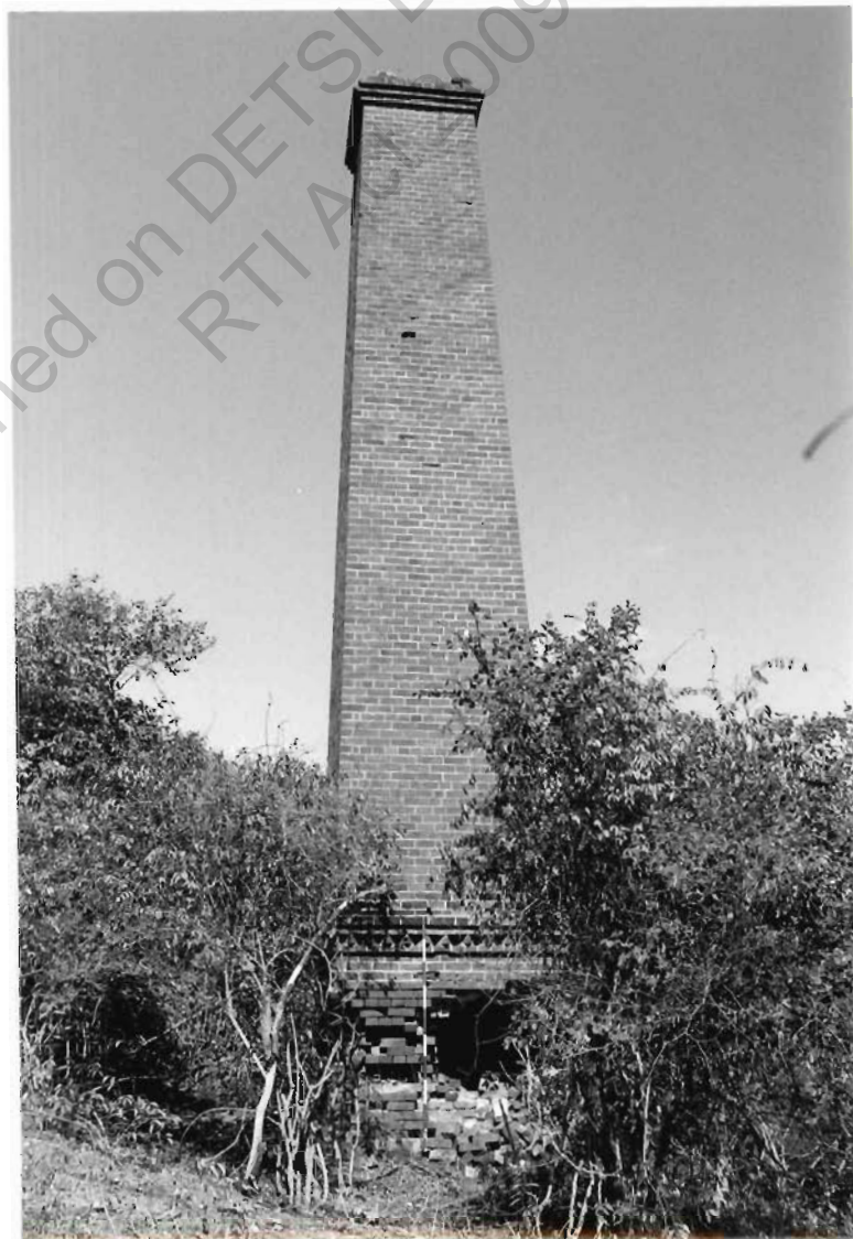
Brick chimney, looking S.
