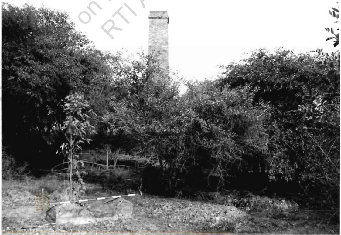
Winding plant foundations, looking SE.
