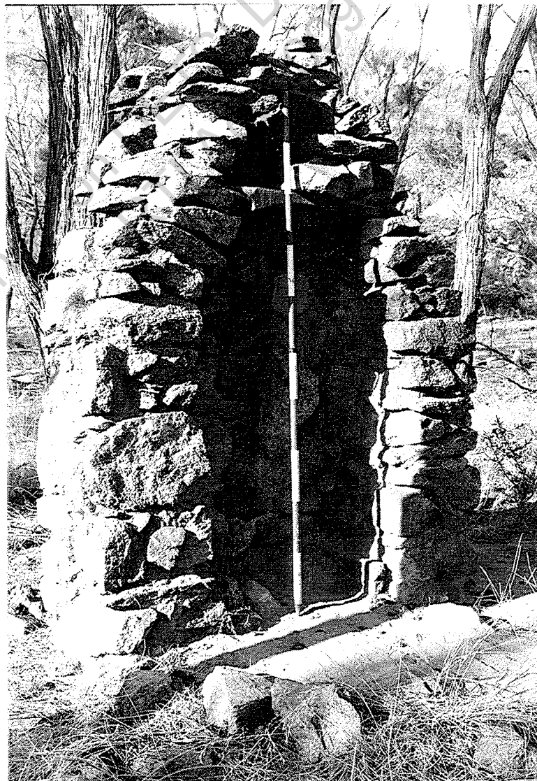
Stone chimney of hut, looking NE.
