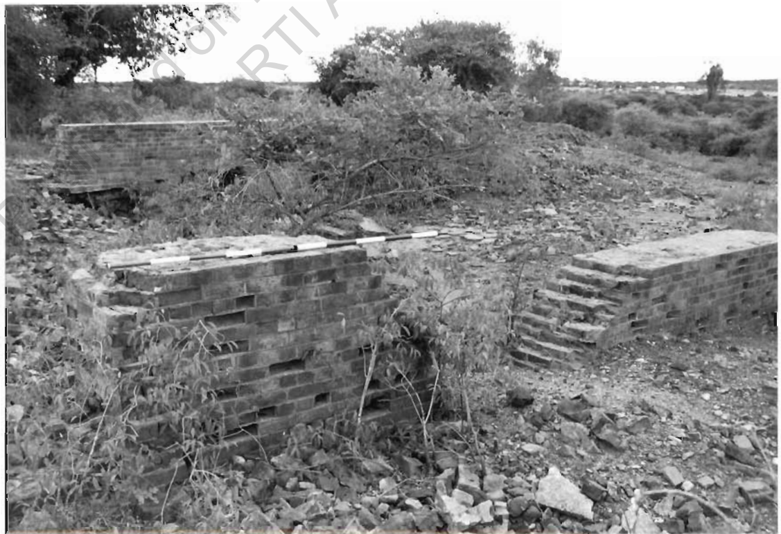
Battery shed foundations, looking E.
