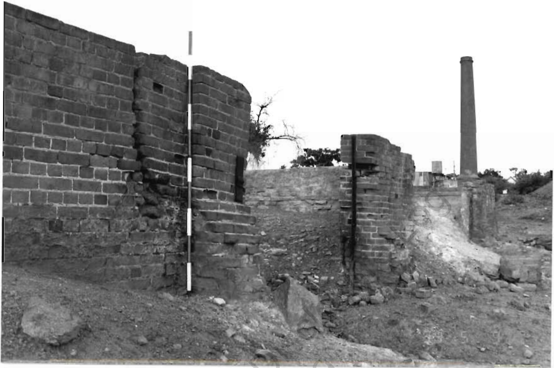
Brick retaining walls of settling tanks, looking SE.
