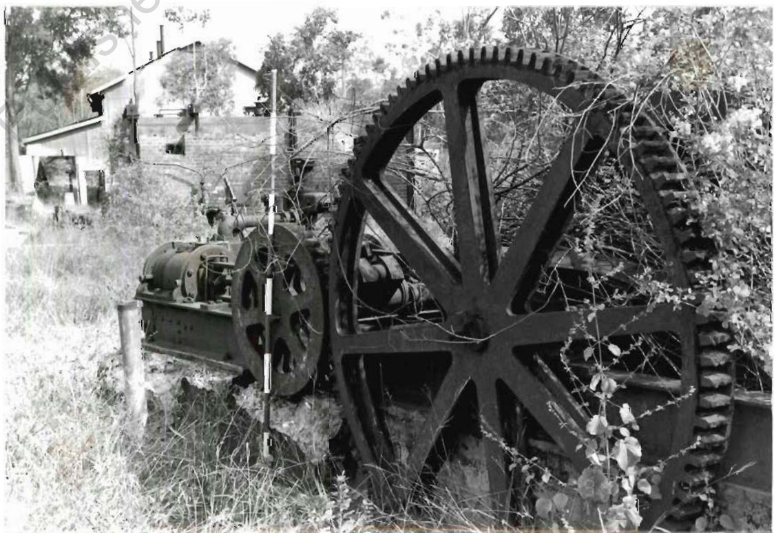
Hornsby winding engine, looking W towards the boiler house and power house.
