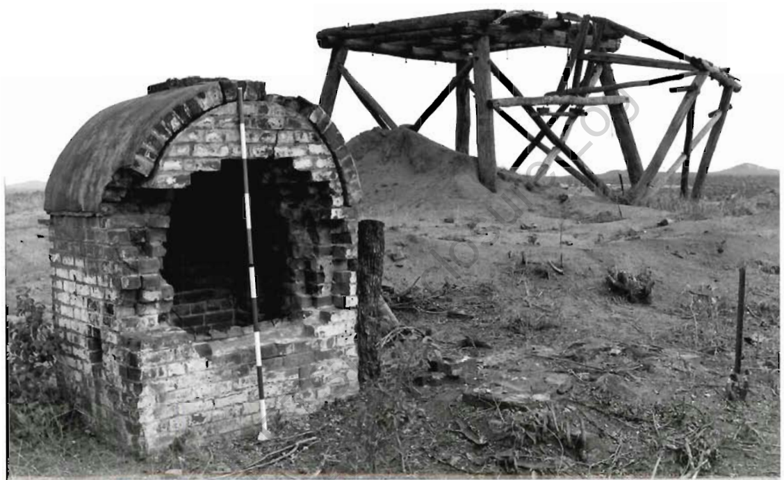
Detonator magazine and underlie shaft headframe, looking NW.
