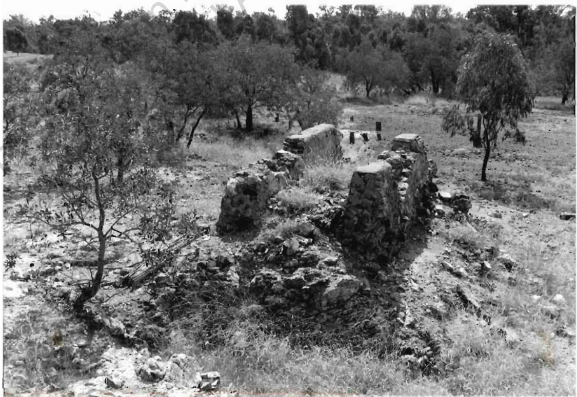
Cyanide plant - stone footings of hopper looking N.
