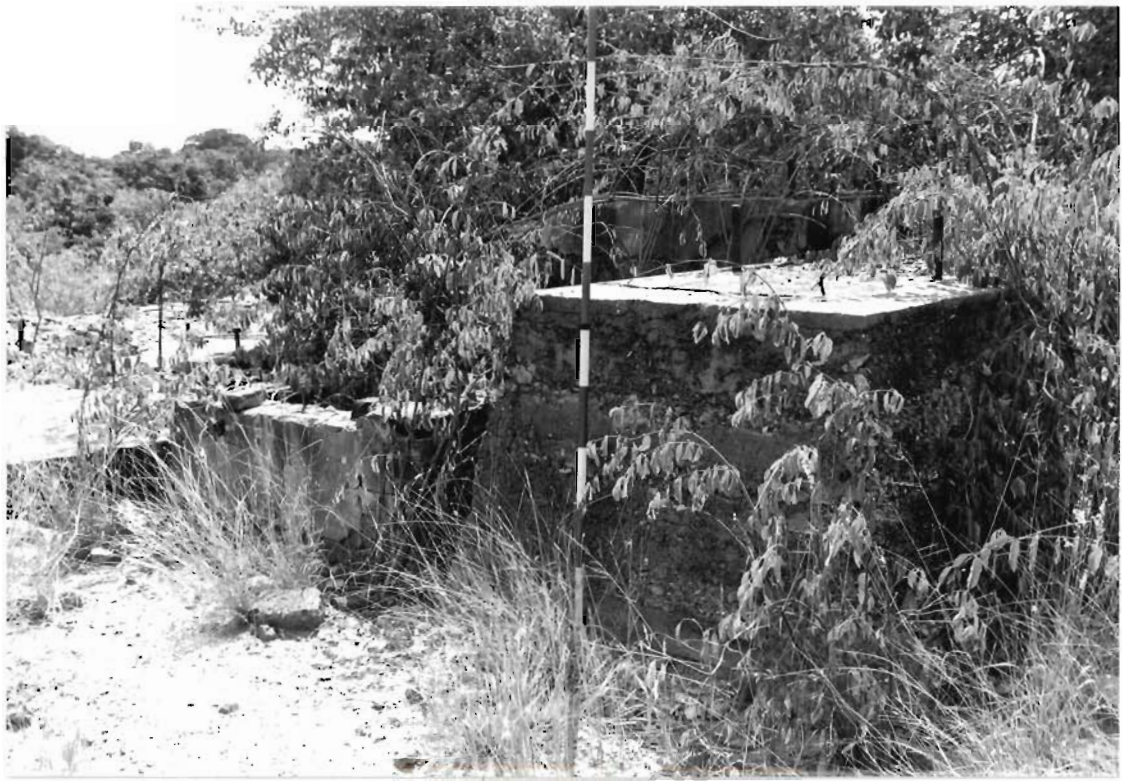
Engine concrete mounts, looking N.
