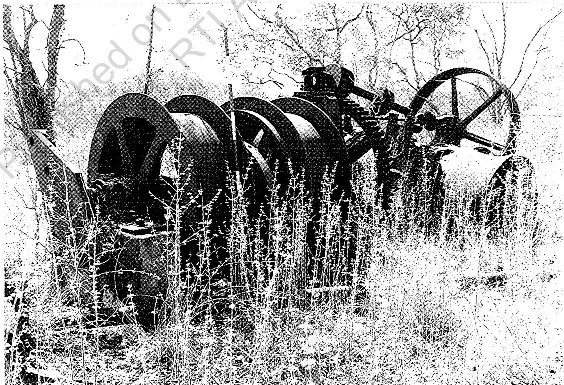
Winding winch (left) and Robey portable engine (right). Looking NW.
