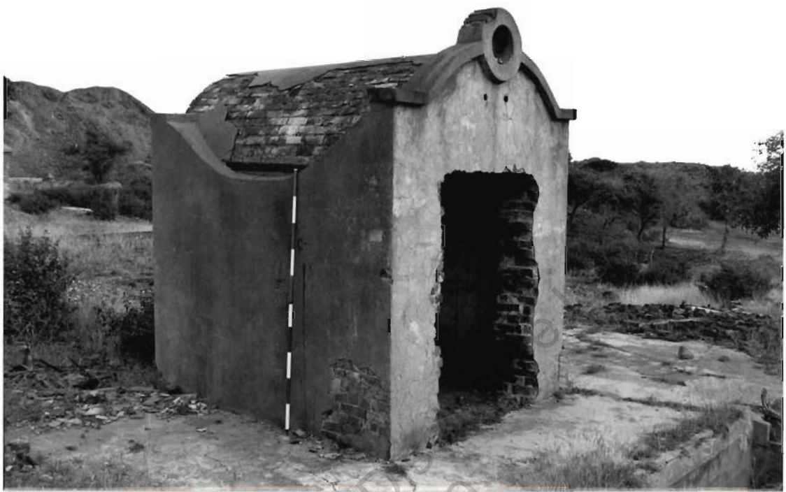
Rendered brick strongroom adjacent to the battery site. Looking SW.
