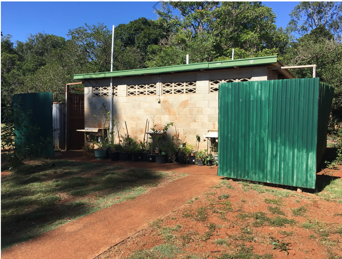
Garden shed adjoining ablutions block (store and shed in background)
