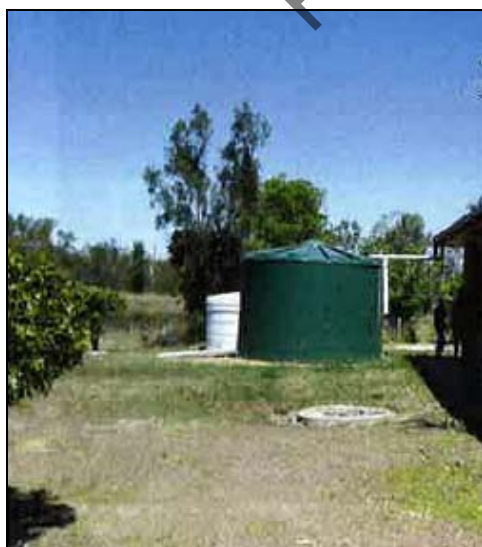
Figure 2. Polyethylene Tank, with White Tank behind.
