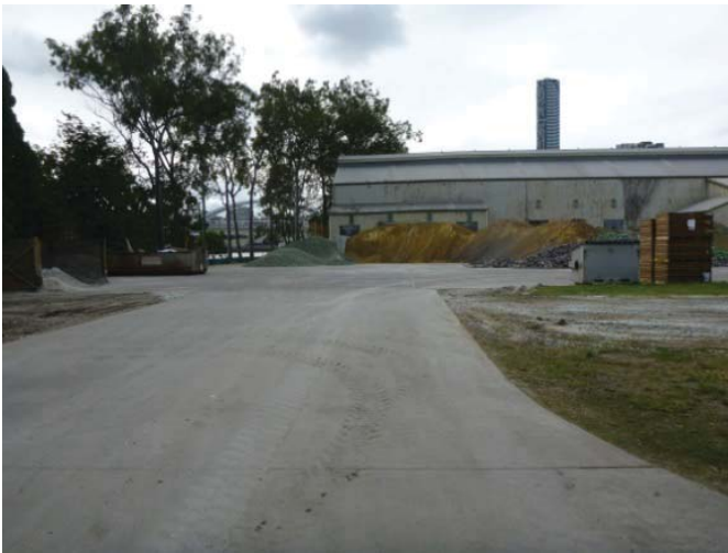
Photo 13 – Hardstand where glass shards were stored during previous inspection.
