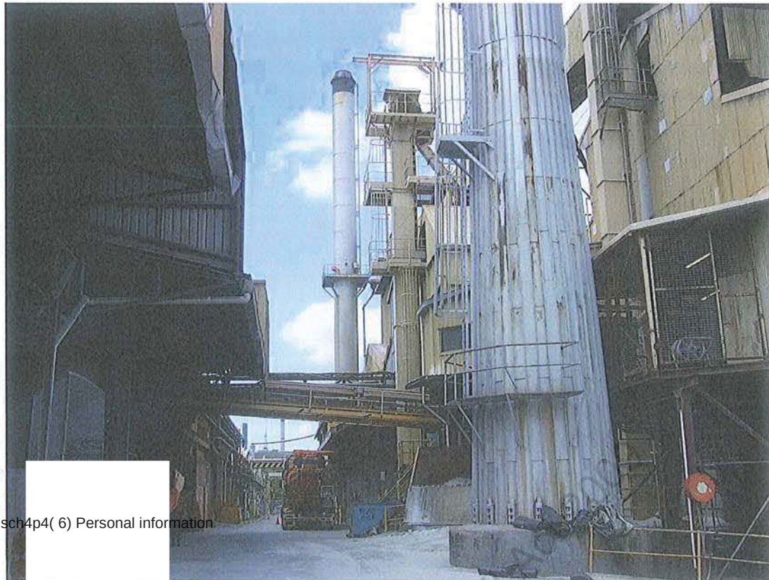
View of Release Point 2 – the QG2 furnace stack at centre-rear of the photograph.
