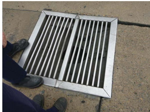
Photo 5 – Stormwater drain with drain warden (filter sock)
