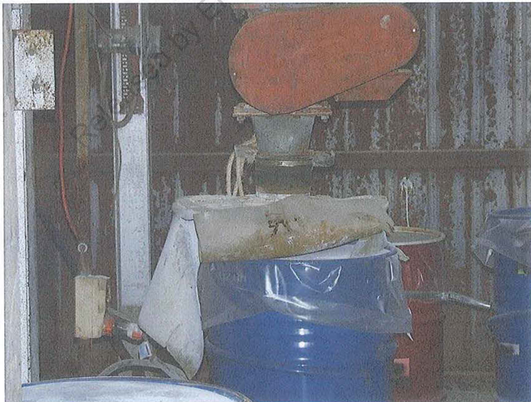
View of the 200 litre drum used to collect the stannic chloride and ammonia chloride particulate matter for disposal in accordance with condition B15.
