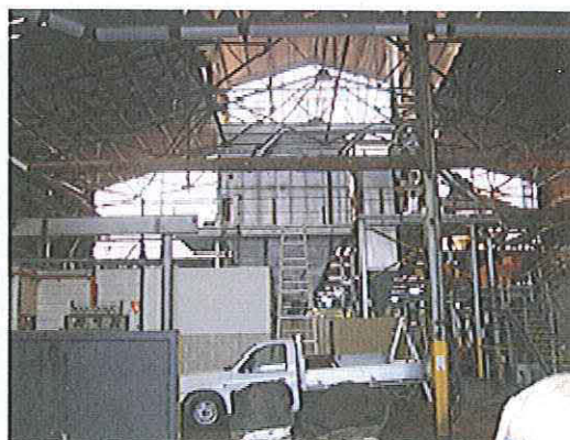
Photo: 1020610 – Batch house.
