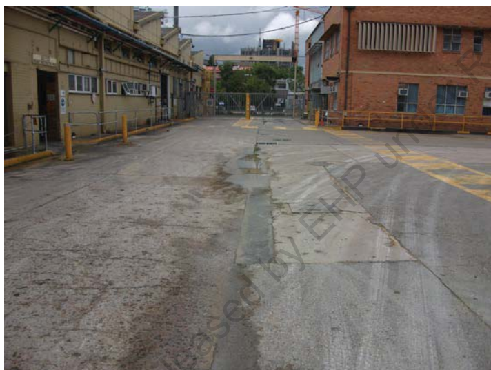
Photo 2. Stormwater drain with 'drain warden', photo captured looking at the entry driveway near Montague Road/Brereton Street.
