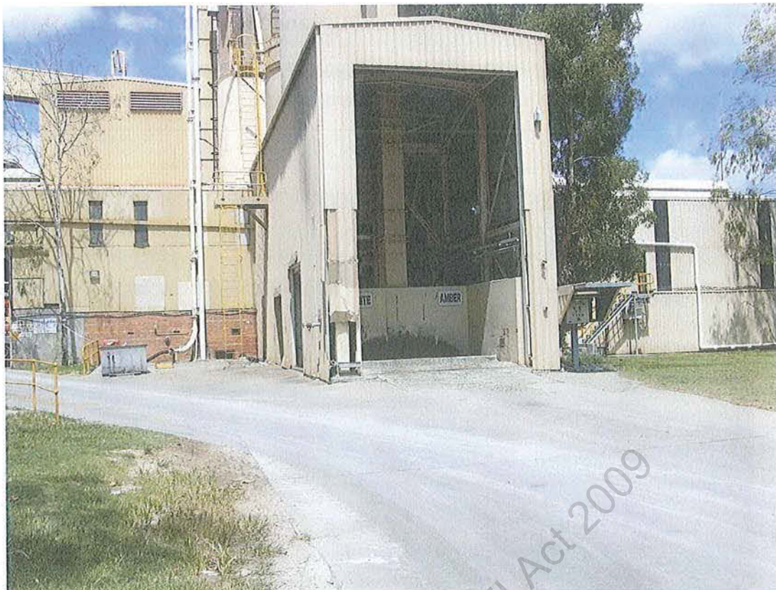
General view of the materials handling area where raw materials including silica, soda ash and recycled glass are delivered prior to batching for glass bottle manufacture. Flint (clear), amber, and green glass bottles form the majority of products manufactured at the site.
