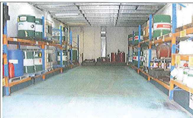
Photo: 1020631 – Chemical storage – rollover bund at entrance
