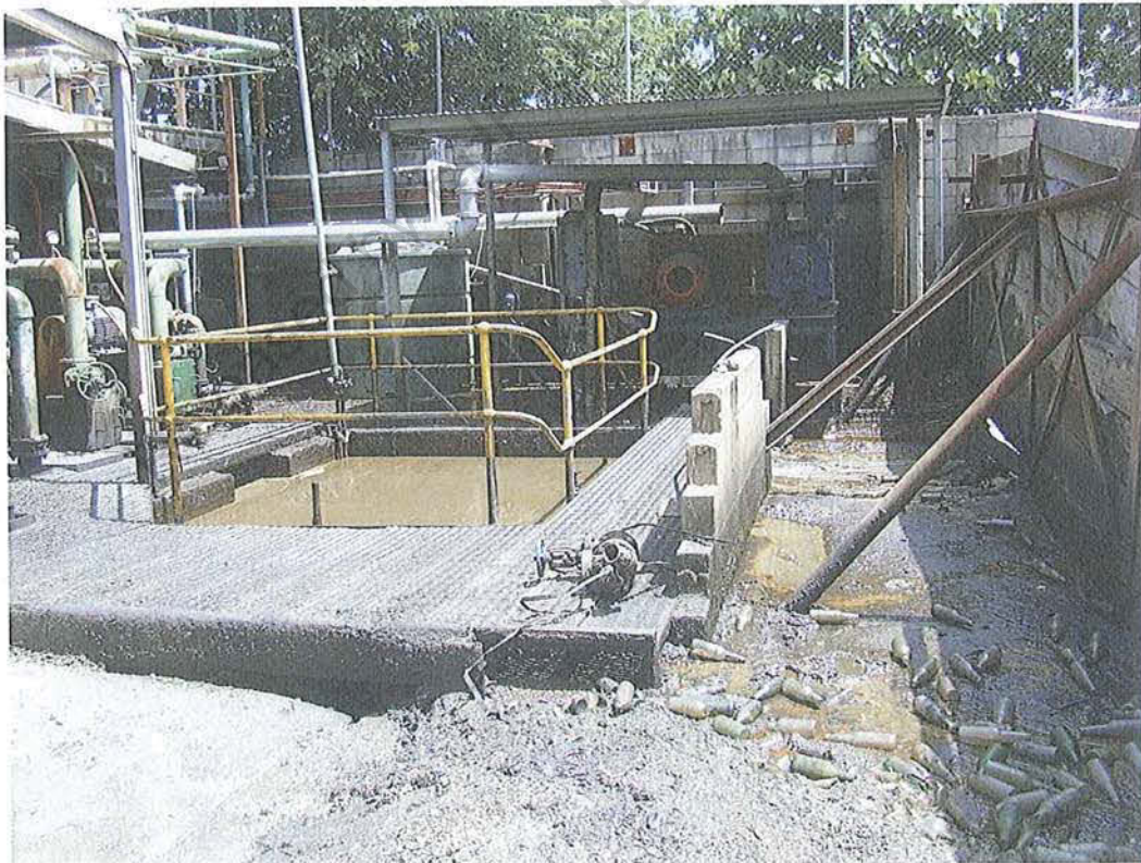
View if the site "sump". Localised odours of an unpleasant nature were readily detectable in the vicinity of the sump.
