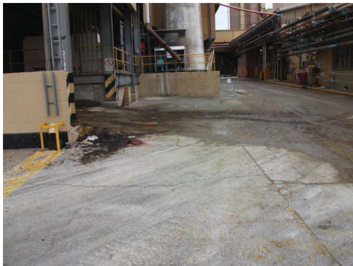
Photo 1. Loading bay diagonal to mould shed/spray booth.
