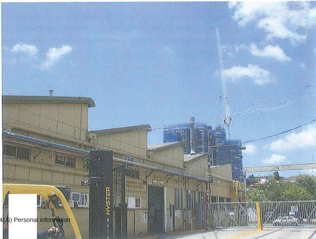
View of Release Point 3 – Machine shop fume extraction (larger stack framed by the high-rise construction).
