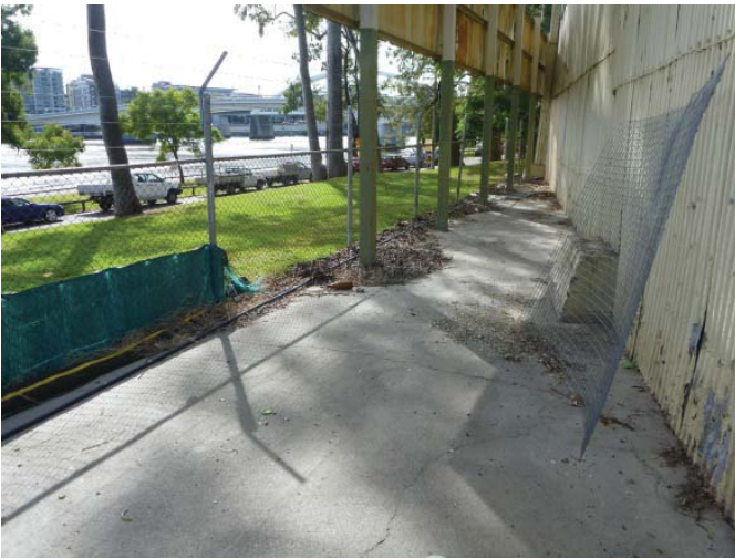
Photo 16 – Dust/particulate fence finishes before the end of the site boundary.
