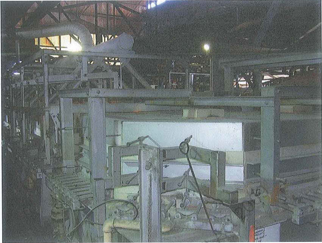
Two views of the QG1 refiner, immediately downstream of the furnace. Specialty chemicals used to modify glass viscosity and other properties are added at the refining stage.
