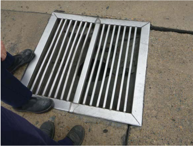
Photo 5 – Stormwater drain with drain warden (filter sock)
