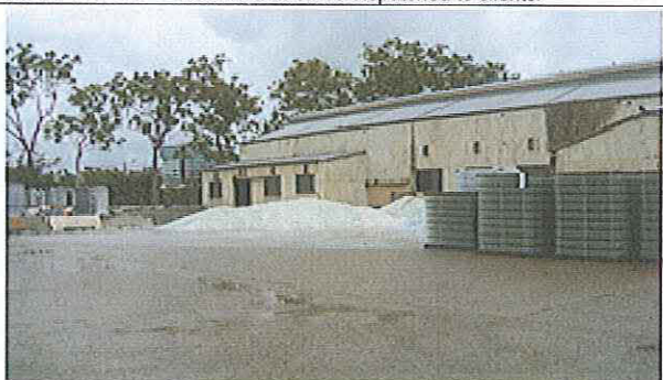
Photo: 1020594 – Hardstand area – crushed glass is banded – the product is recycled.
