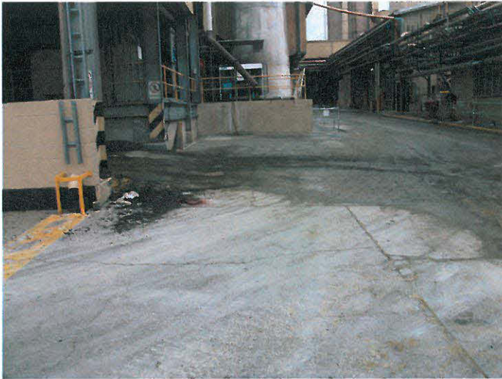
Photo 1. Loading bay diagonal to mould shed/spray booth.
