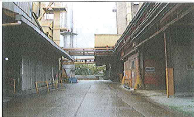
Photo: 1020635 – Housekeeping has improved since the last inspection in 2009.
