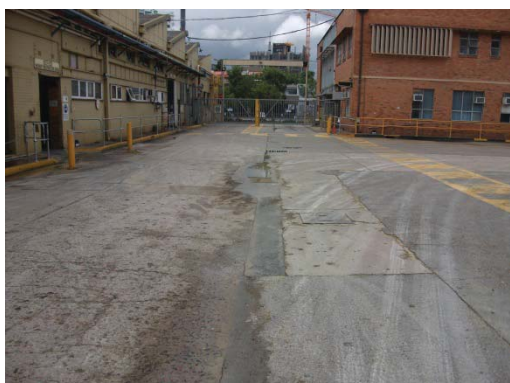
Photo 2 – Photo captured looking at the entry driveway near Montague Road/Brereton Street. Note sediment laden water in channel flowing to stormwater drain.
