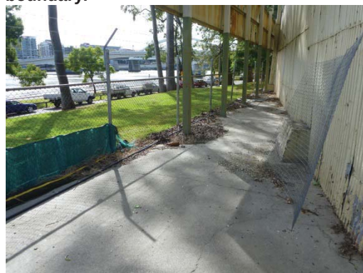
Photo 16 – Dust/particulate fence finishes before the end of the site boundary.
