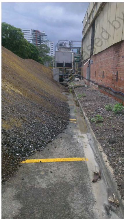
Photo 6 – Surplus stockpiling of crushed glass, banded by cement bollards.
