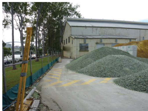
Photo 15 – Glass stockpiles the hardstand. Dust/glass particulate fence along site boundary.
