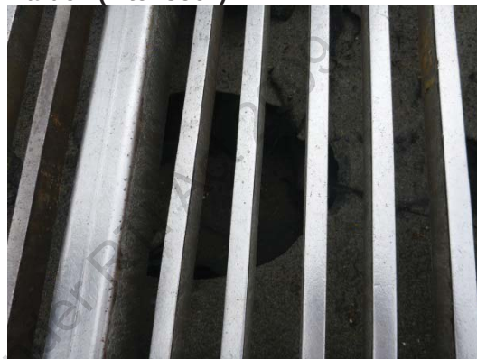
Photo 6 – Close up of stormwater drain
