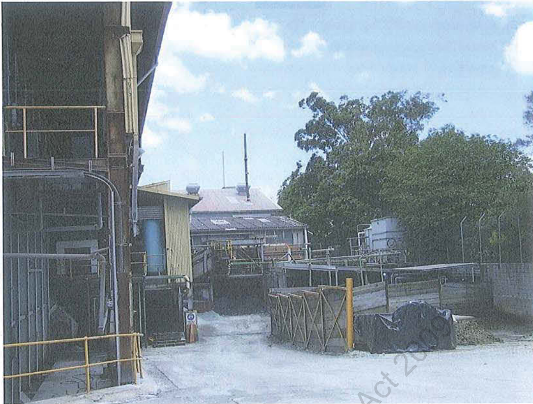
View of Release Point 6 – delivery cleaning oven.
