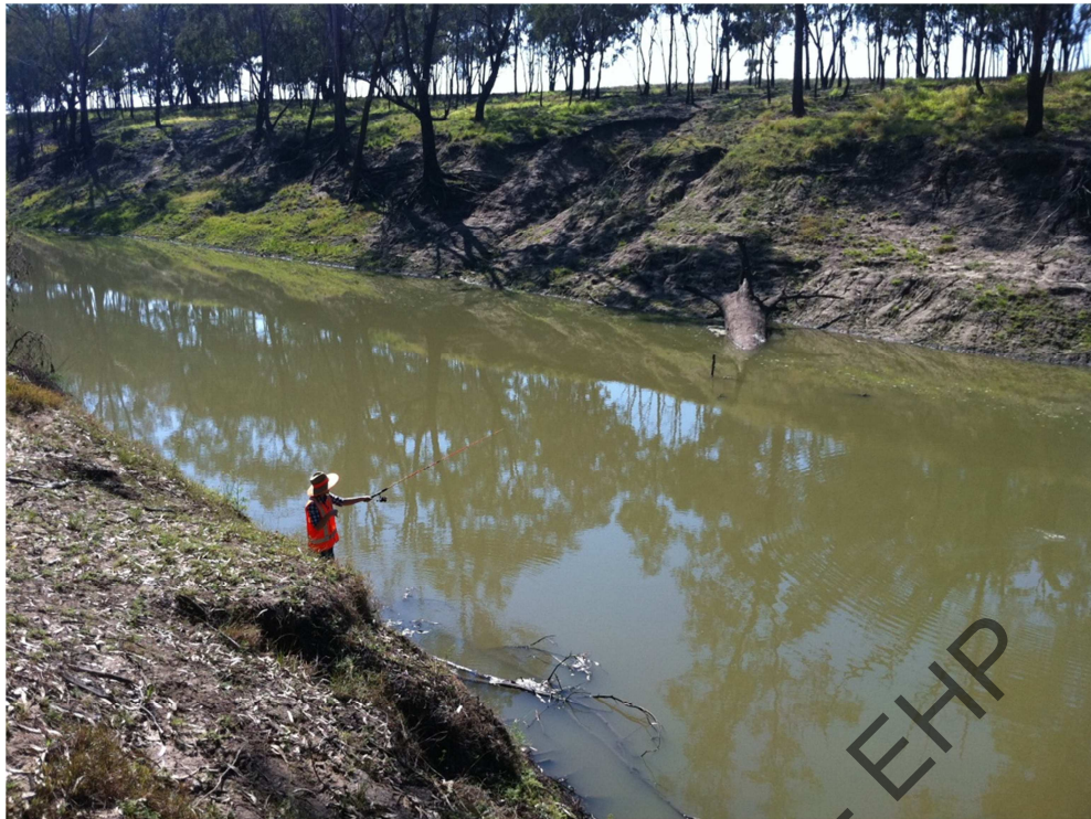
Figure 3. Condamine River crossing at KP 68.6
