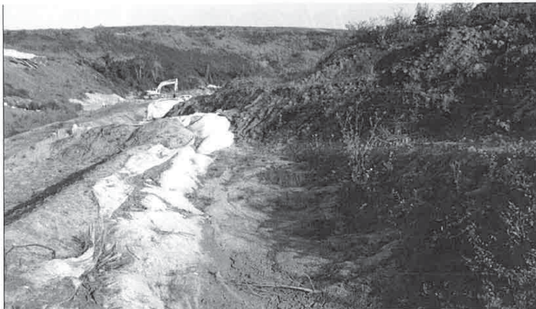
Photo 1: Southern part of contaminated stockpile retention basin
