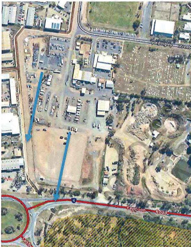
Figure 1 – Blue arrows indicates concrete drainage channel and new culvert under Yeppoon Rd.
