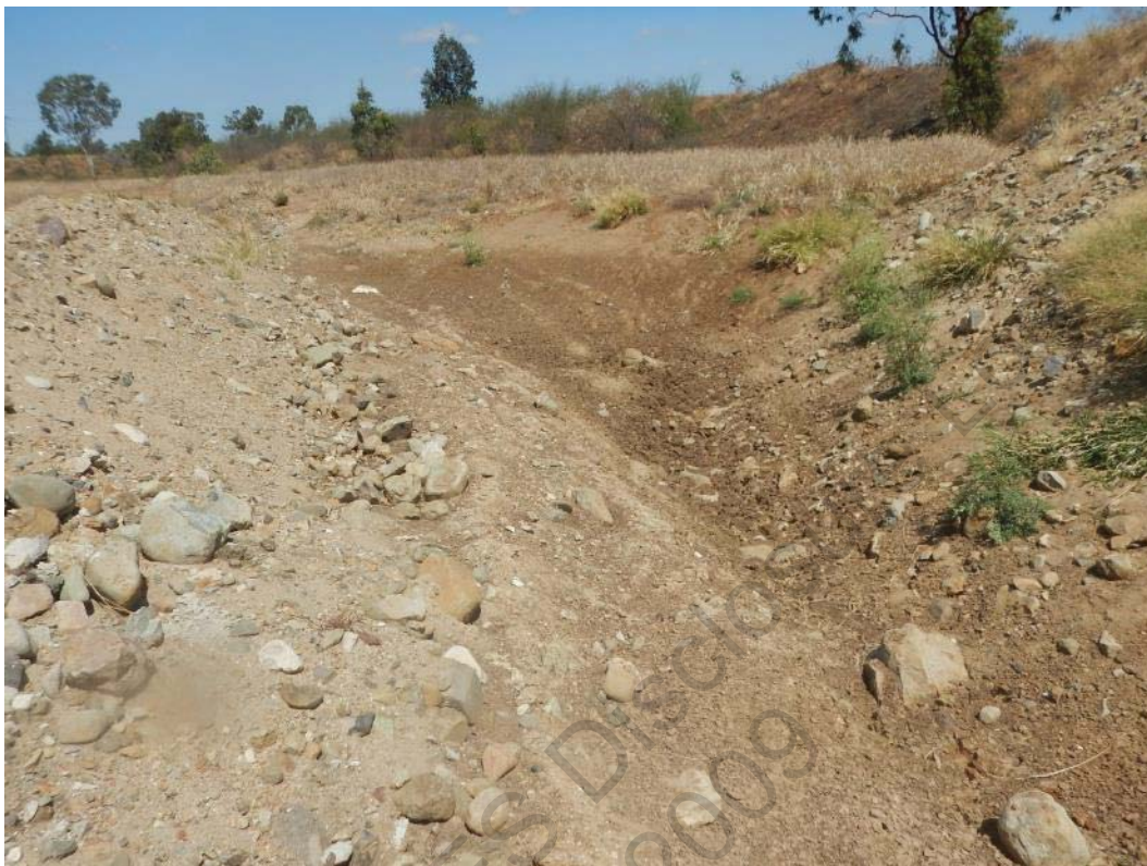
Photo 5 Settling Area on Downstream Side of Plug Formed by North Pit Dump
