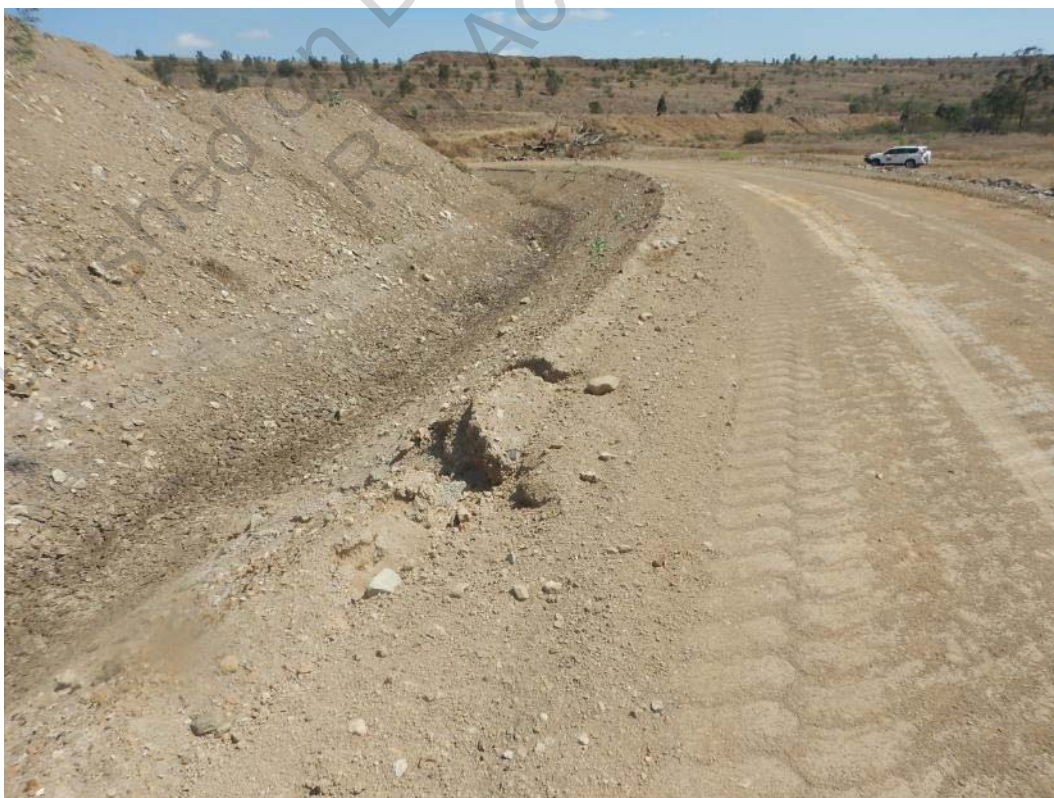
Photo 10 Crest and Downstream Side of Plug (Approximate Chainage 100m)
