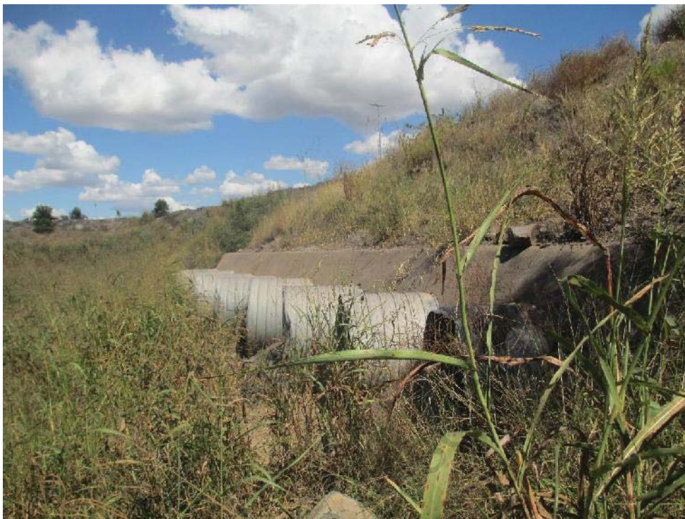
Figure 6.9 High Level Culverts At Upstream Side Of Haul Road
