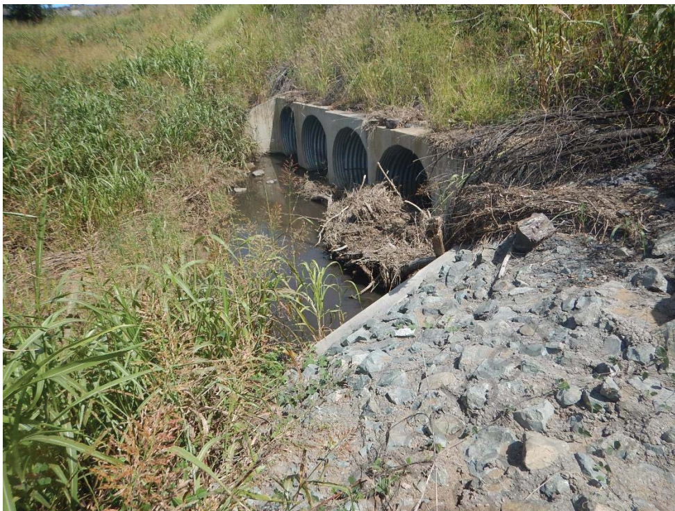
Figure 6.11 Low Flow Culverts at Upstream Side of Haul Road
