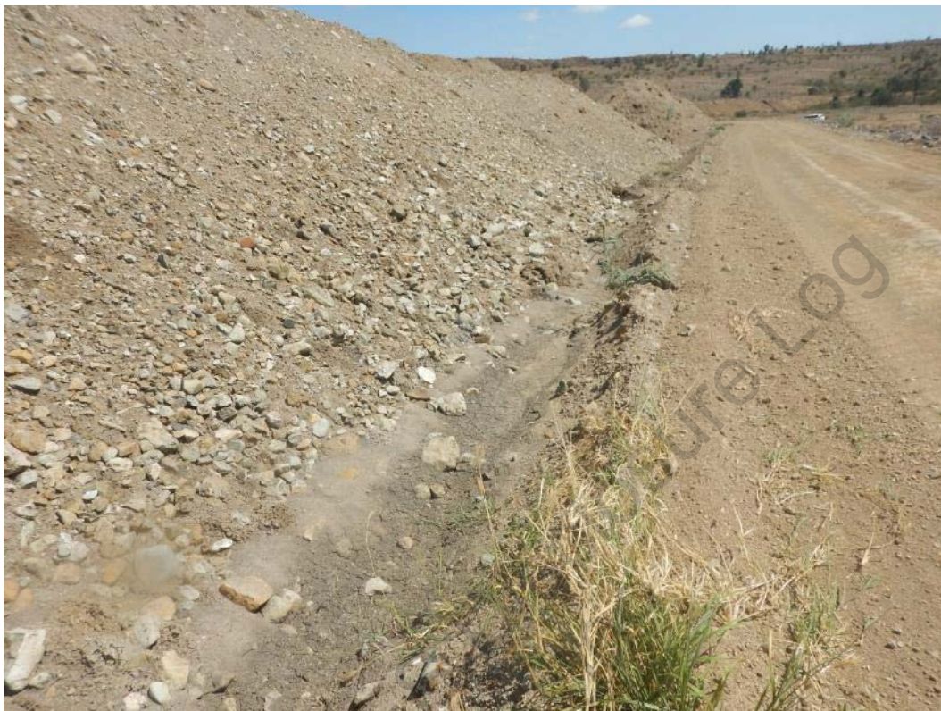
Photo 9 Crest and Downstream Side of Plug (View from North-East End)
