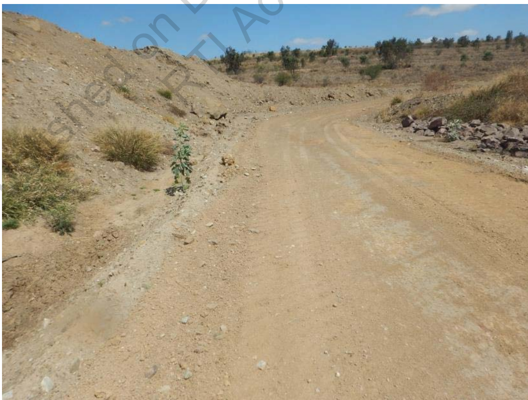
Photo 12 Crest and Downstream Side of Plug (Approximate Chainage 170m)
