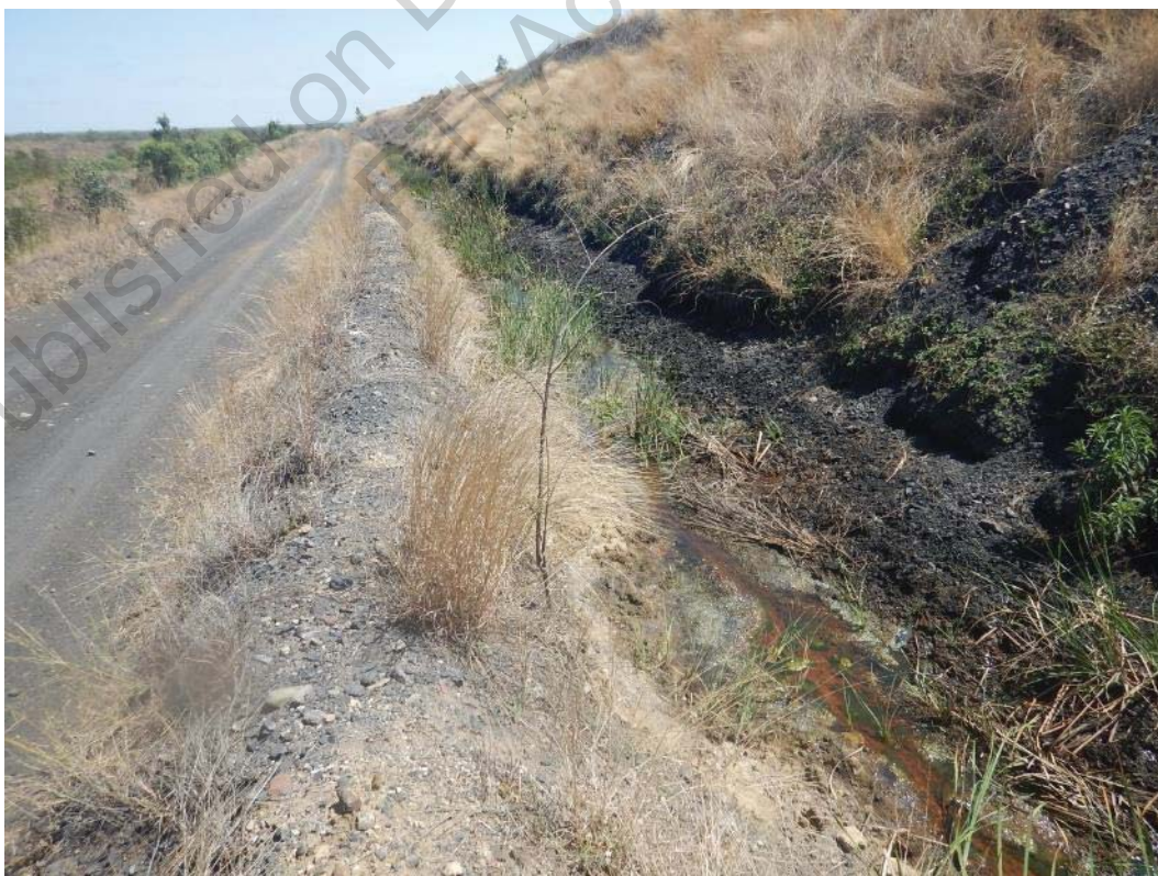
Photo 8 Western Wall of Cell 2 and Seepage Flows in Drain above Starter Bund (View to north)
