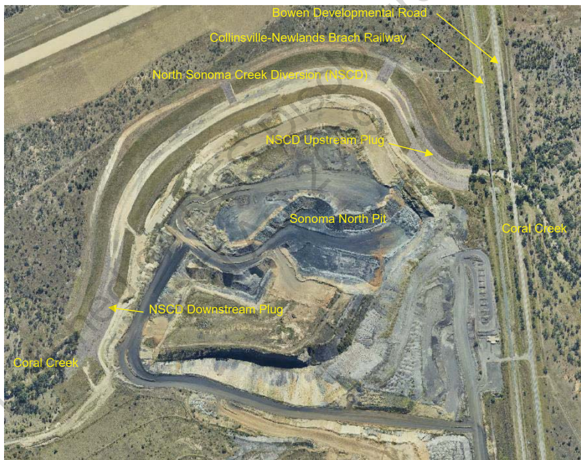
Figure 4.1 Aerial image of NSCD including Upstream and Downstream Plugs (aerial photo taken June 2019)
