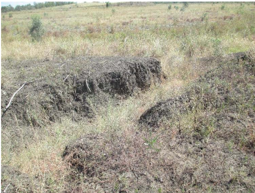
Figure 6.17 Gully Erosion Of Right Bank Upstream Of TMC-Div3
