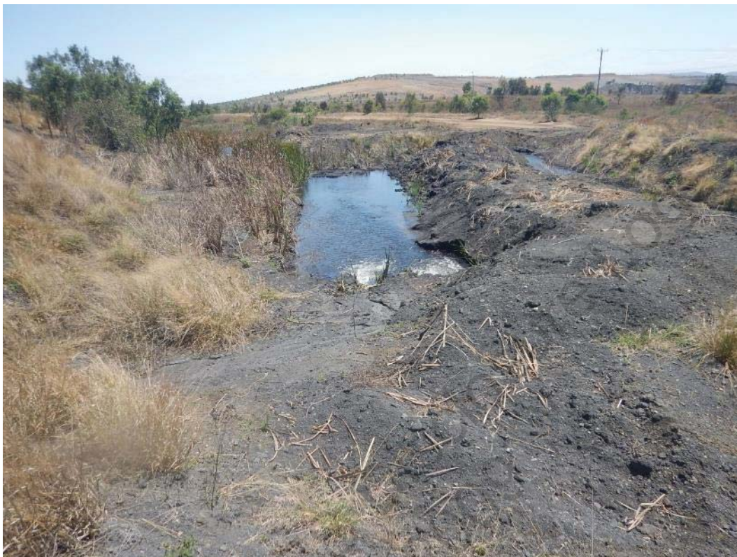
Photo 21 View Downstream Along Eastern Solution Trench and Clean Water Drain from Road Crossing at North-Eastern Corner of Cell 3
