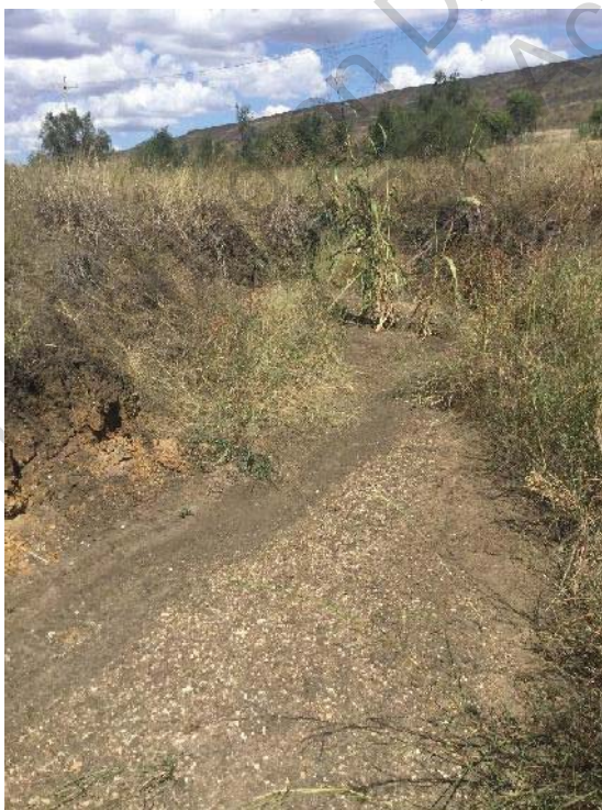
Figure 6.20 View Along Erosion Gully On Left Bank Of Diversion Downstream Of TMC-Div2
