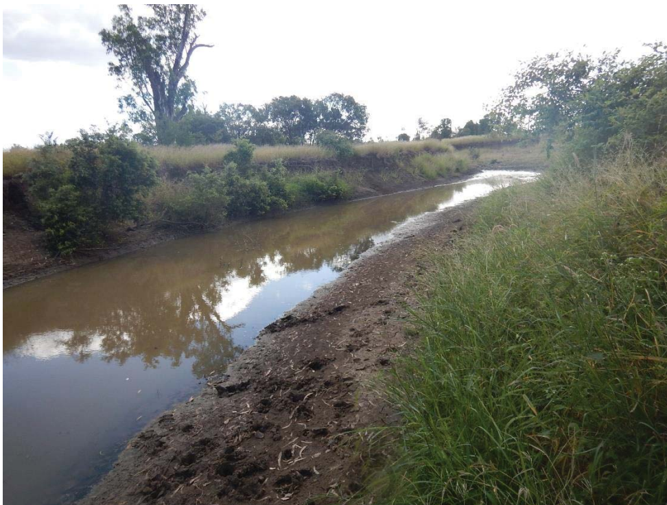
Figure 6.30 Ponding and Bank Steepening At TMC-DS4
