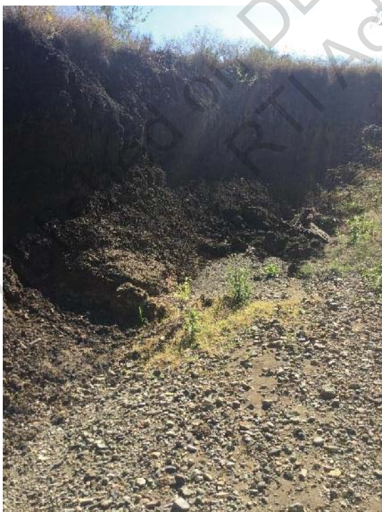
Figure 6.4 Bank Erosion Upstream Of TMC-US4
