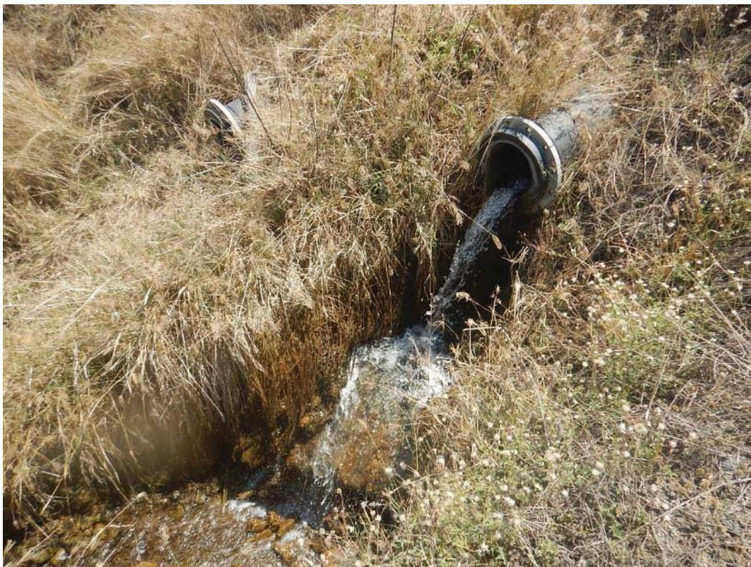
Photo 11 Discharge from Drainage Pipe Outlet into Western Solution Trench
