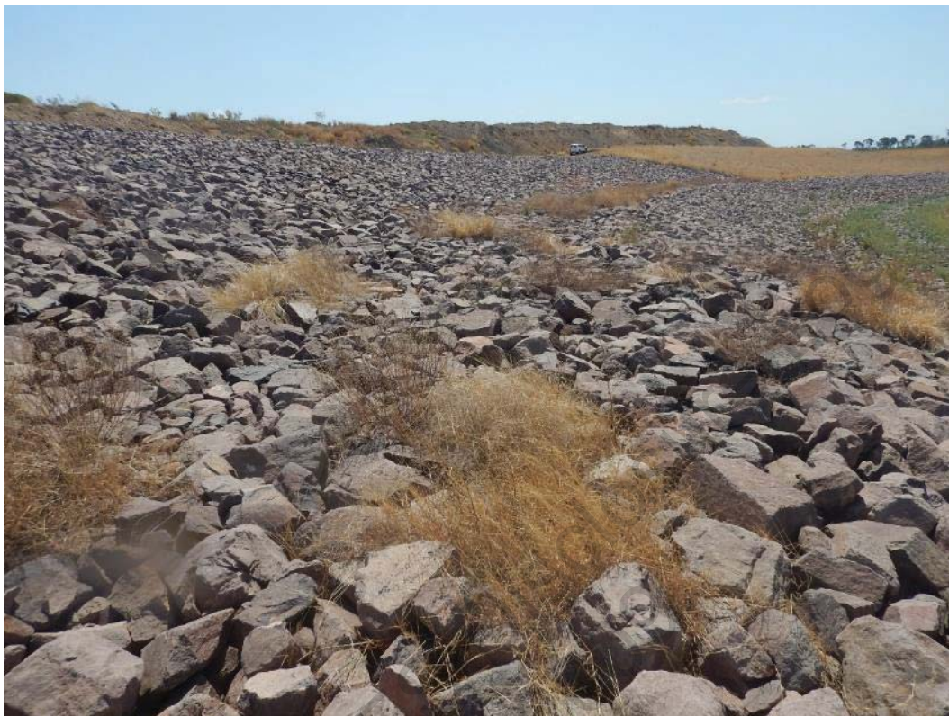
Photo 7 Upstream Side of Plug Viewed from Bench at Upstream End of Plug
