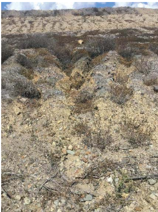
Figure 6.15 Rilling In The Vicinity Of TMC-Div2
