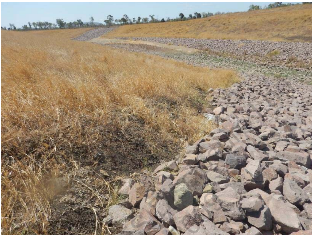
Photo 9 Interface Between Dumped Rock and Vegetation at Upstream End of Plug
