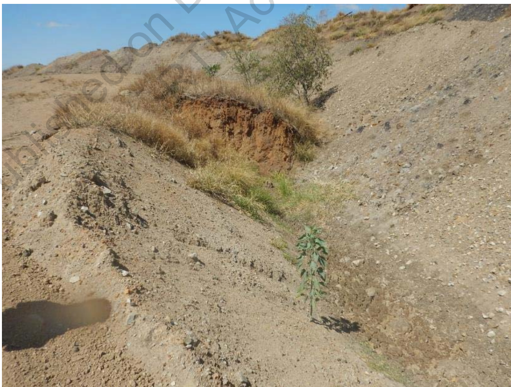
Photo 8 Insitu Creek Bank and North Pit Dump at Upstream End of Plug
