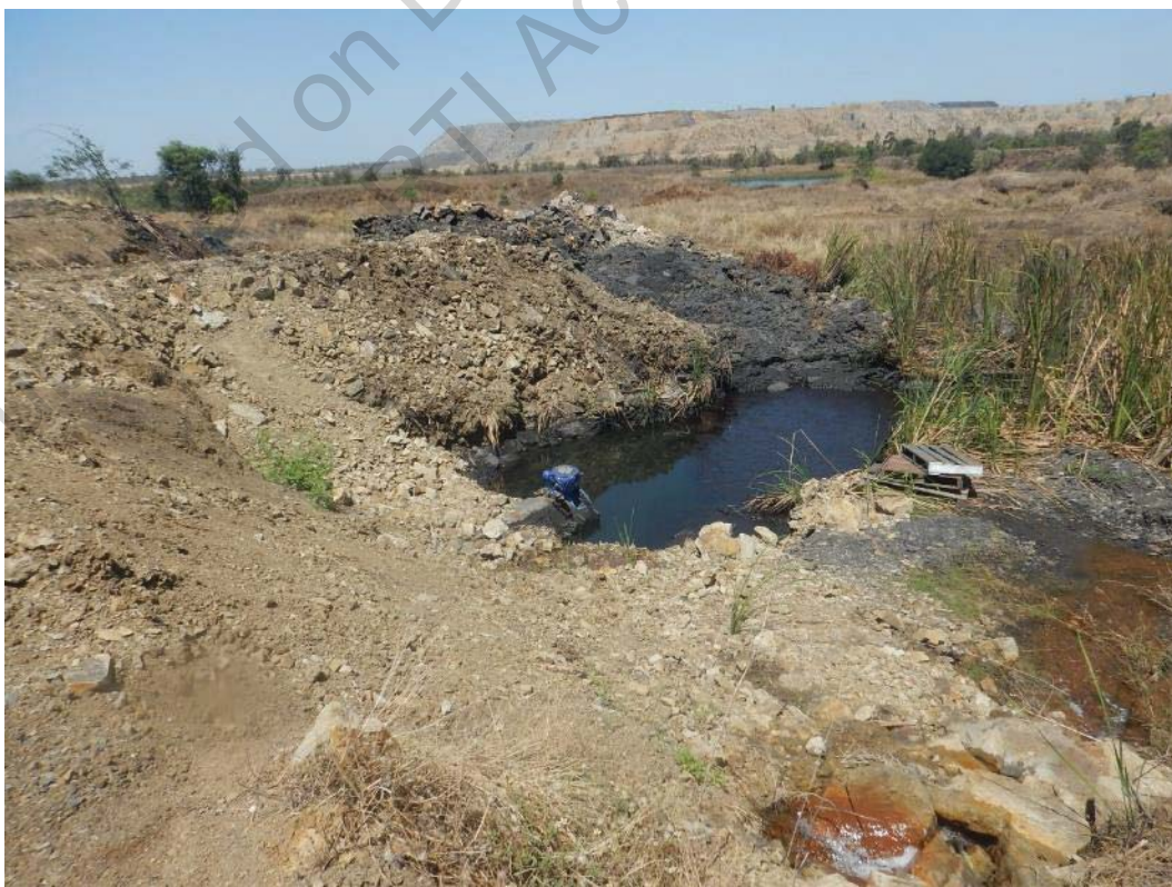
Photo 6 Decant Pipe Outlet into Western Solution Trench Adjacent to Cell 3 with Valve Closed
