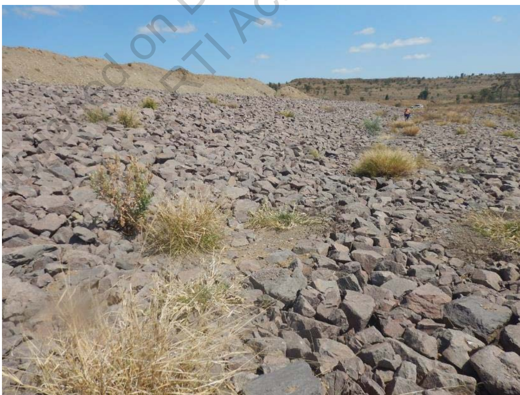
Photo 4 Upstream Side of Plug Viewed from Bench at Upstream End of Plug
