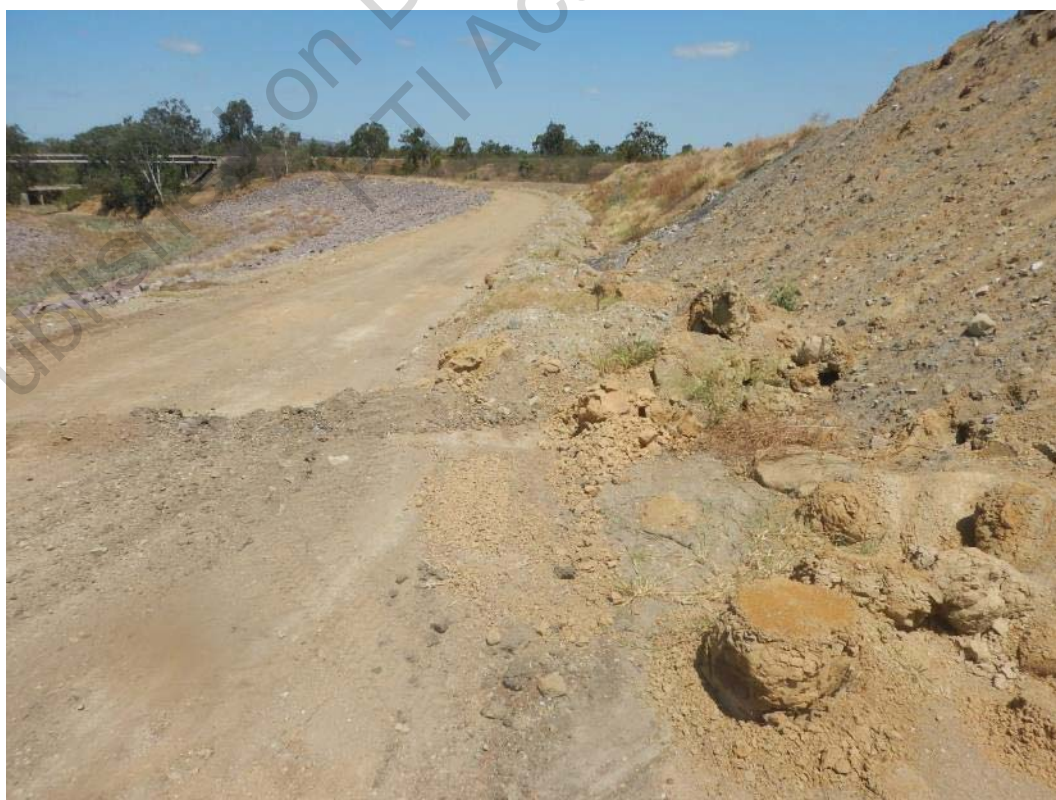
Photo 2 Crest and Downstream Side of Plug (View from North-West End)
