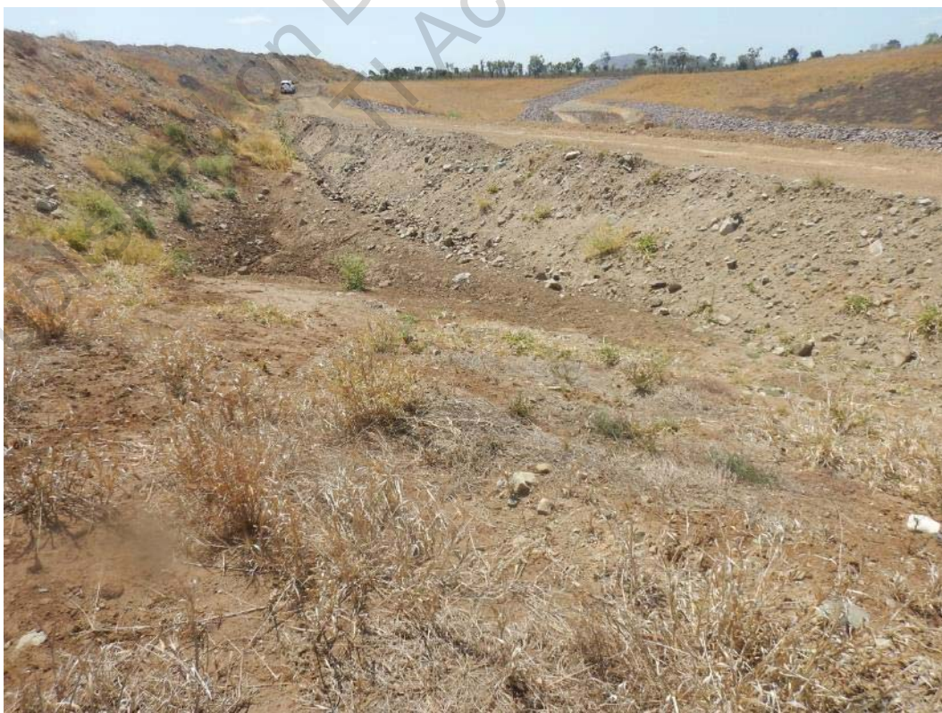
Photo 4 Downstream Side of Plug with Buttrressing by North Pit Spoil Dump
