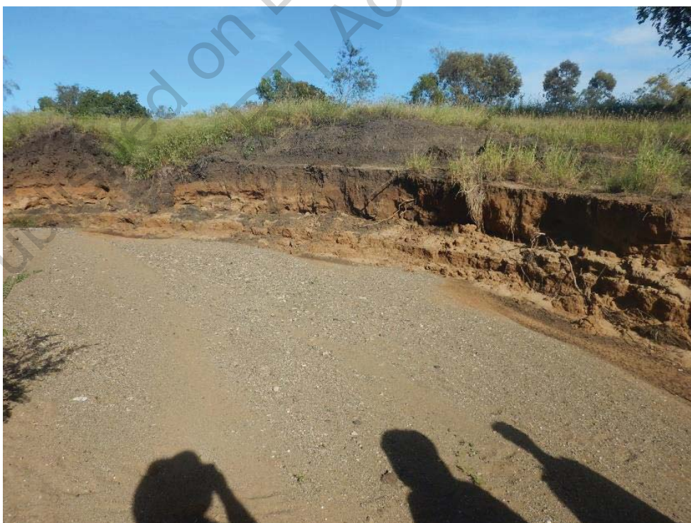
Figure 6.3 Bank Erosion Upstream Of TMC-US4
