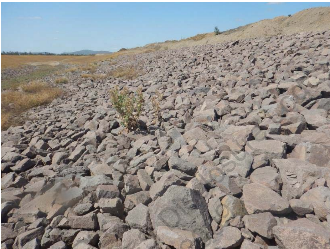
Photo 3 Upstream Side of Plug Viewed from Bench at Downstream End of Plug
