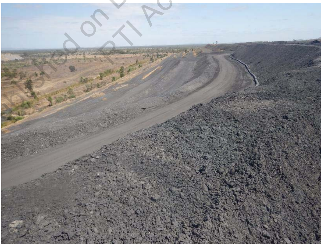
Photo 16 Western wall of Cell 2 Viewed from Top of Cell 3/4
