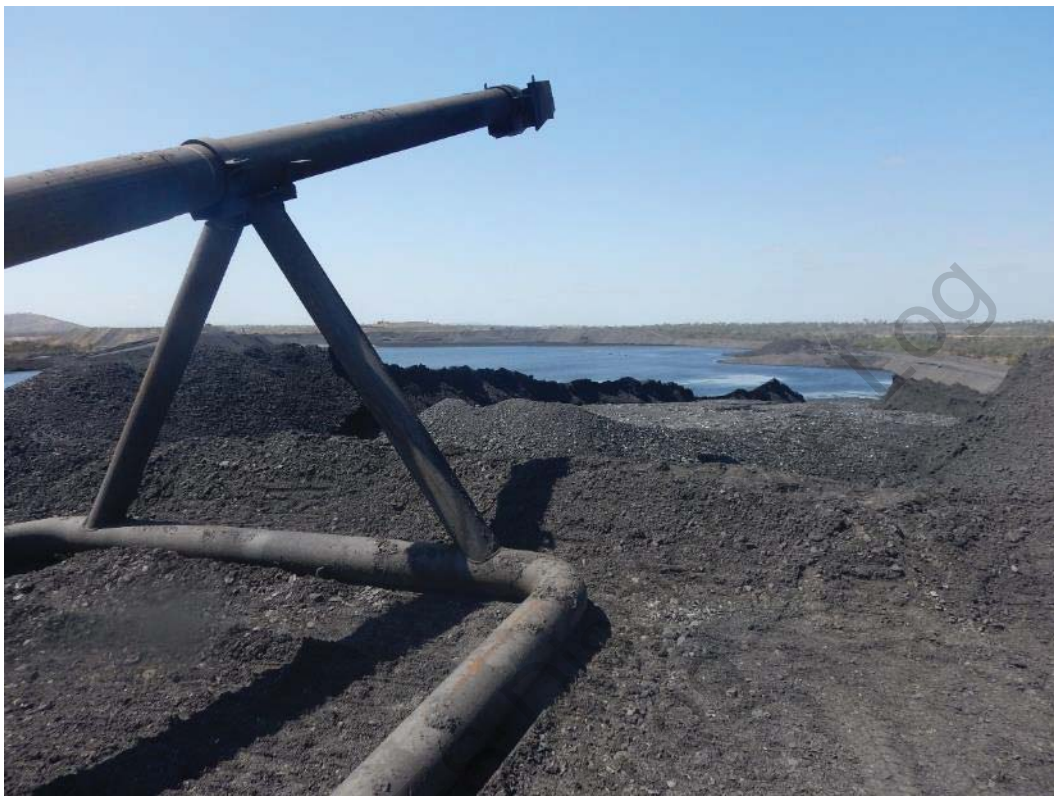
Photo 7 Western Side of Cell 3/4 Viewed from the Top of Partially Constructed Fifth Wall Raise
