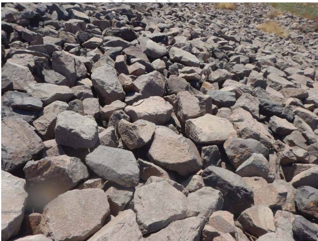
Photo 6 Rock Surface Treatment on Upstream Side of Plug
