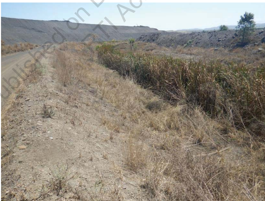
Photo 18 Eastern Solution Trench Adjacent to Cell 3
