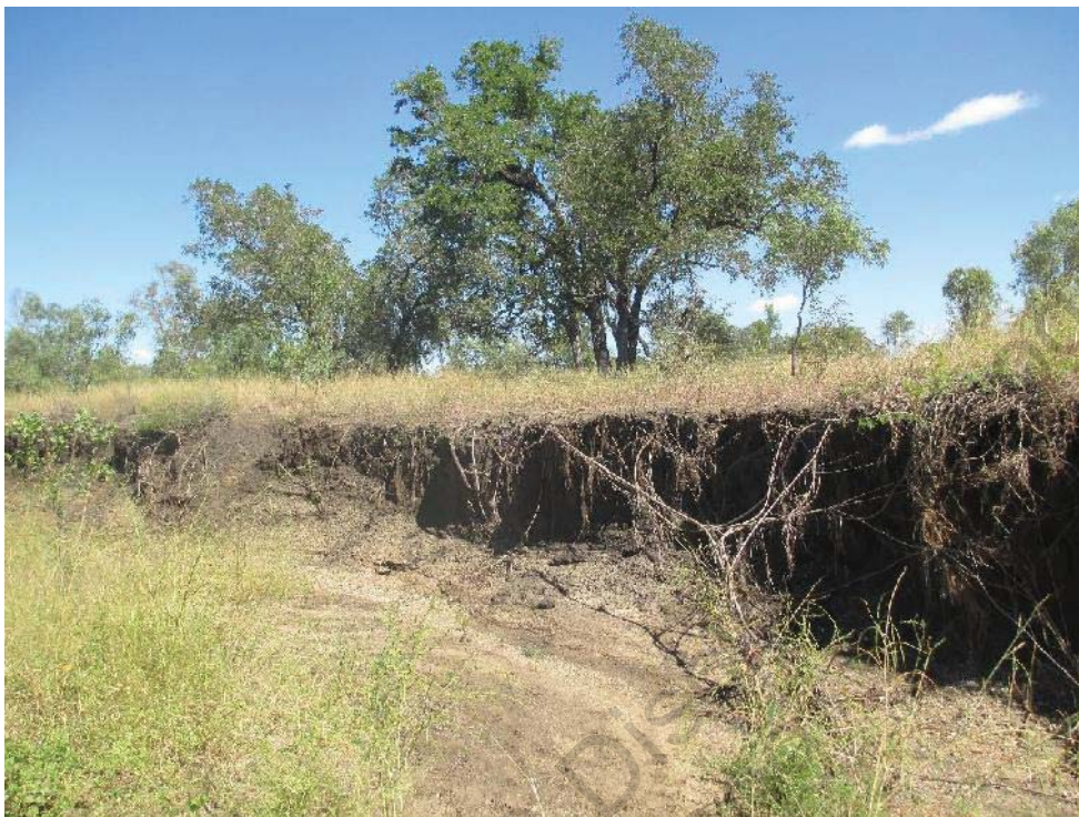
Figure 6.1 Bank Erosion And Undercutting Downstream Of TMC-US1
