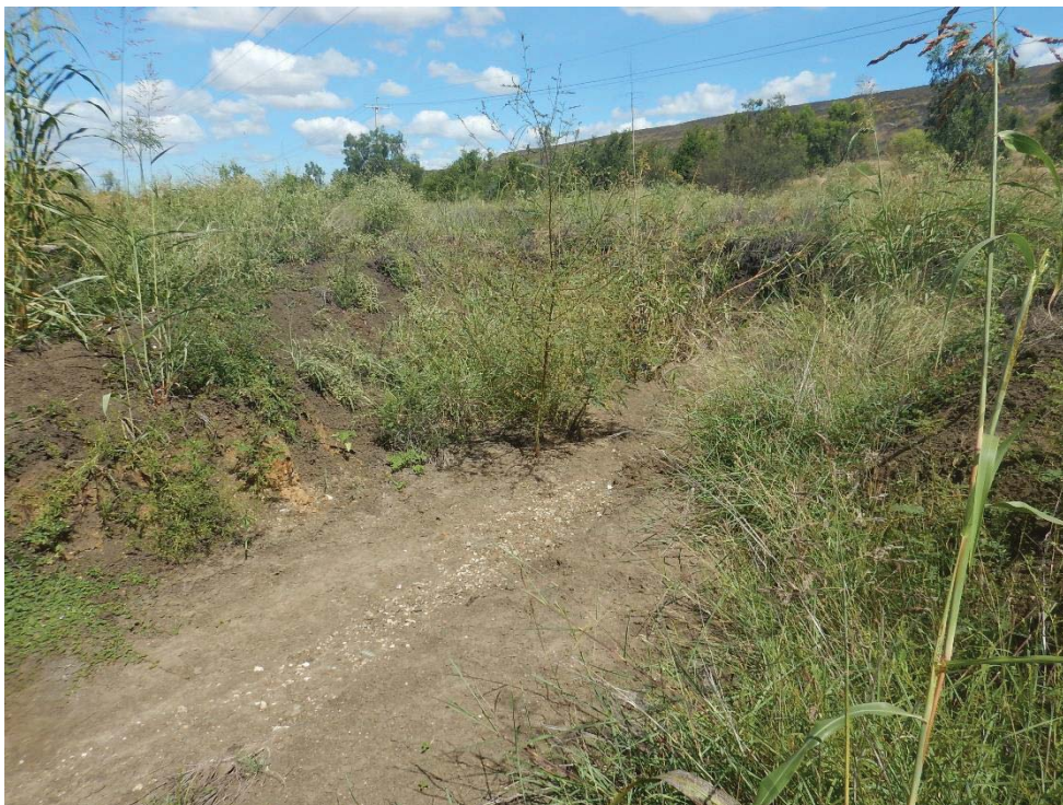
Figure 6.19 Upstream Limit of Erosion Gully (View Towards SD5 and MIA)
