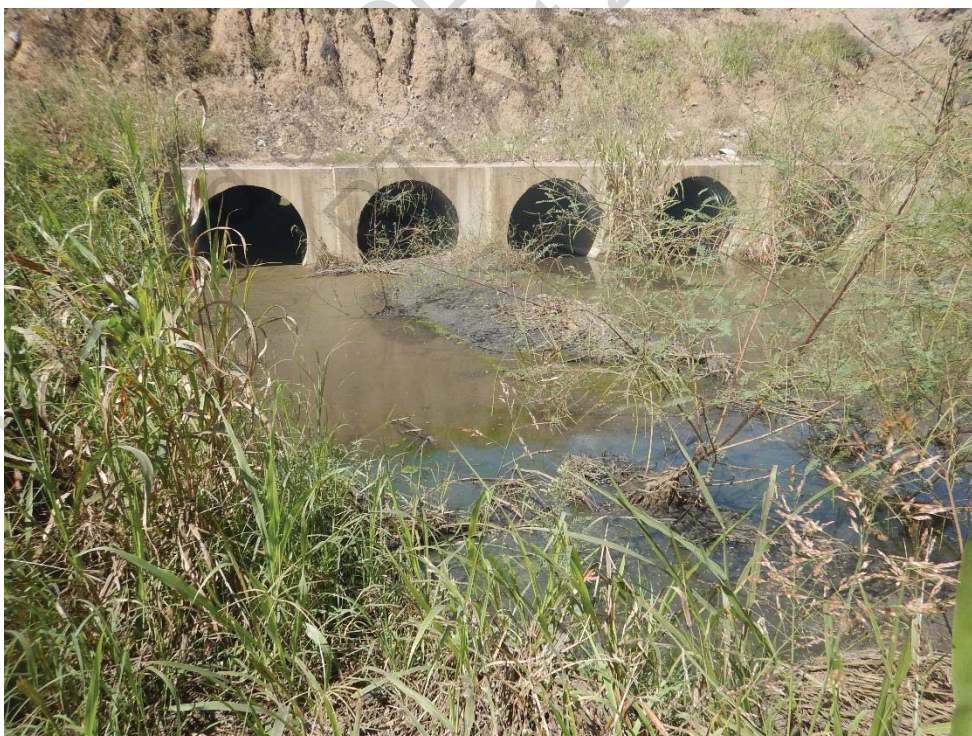
Figure 6.14 Downstream Headwall of Low Level Haul Road Culverts
