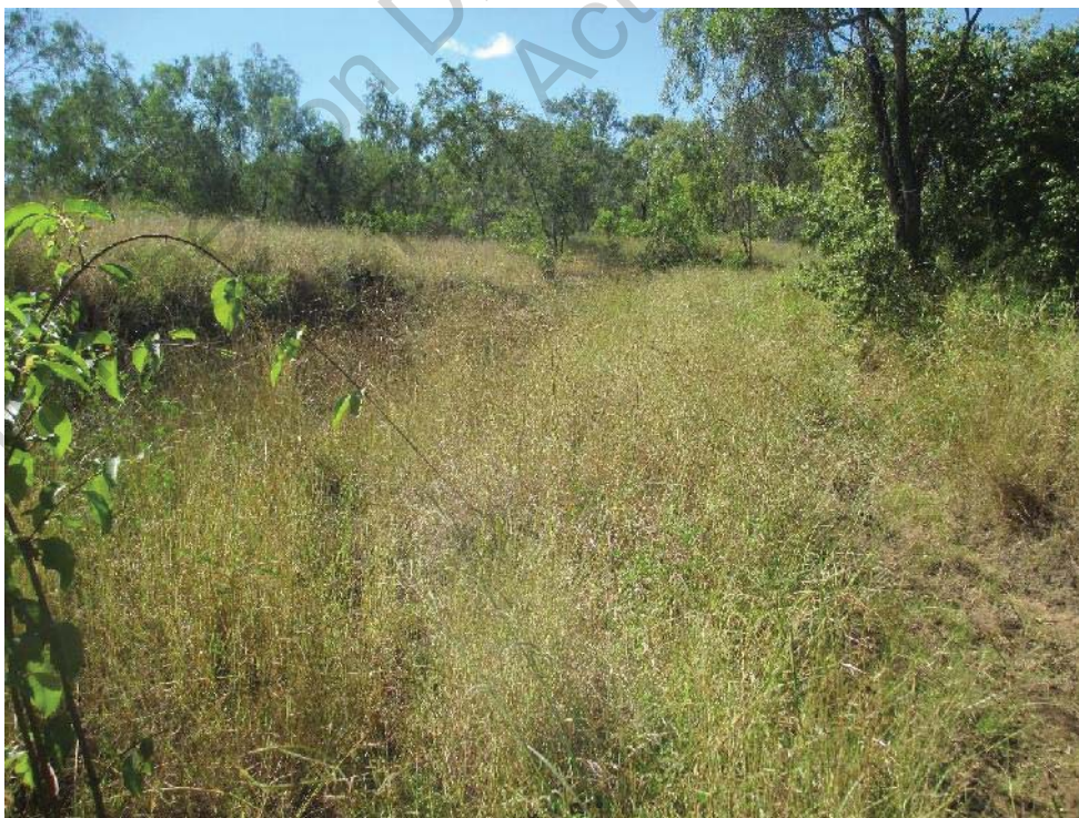
Figure 6.2 Grass Establishment In Channel At TMC-US2
