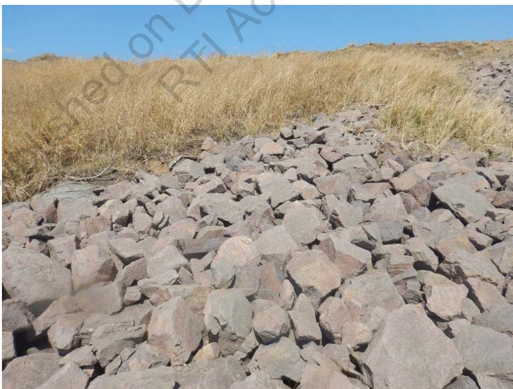
Photo 6 Interface Between Dumped Rock and Vegetation at Upstream End of Plug
