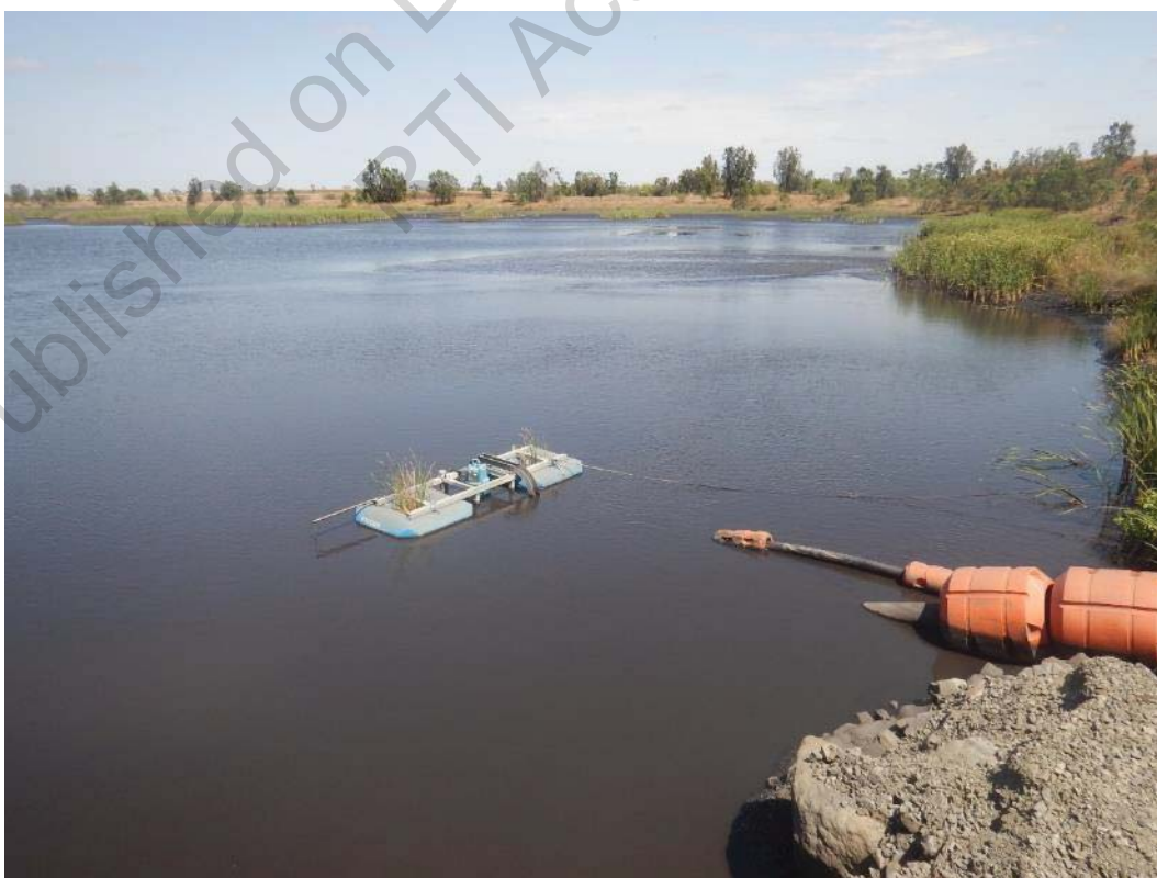
Photo 6 Return Water Dam Pump Suction Line
