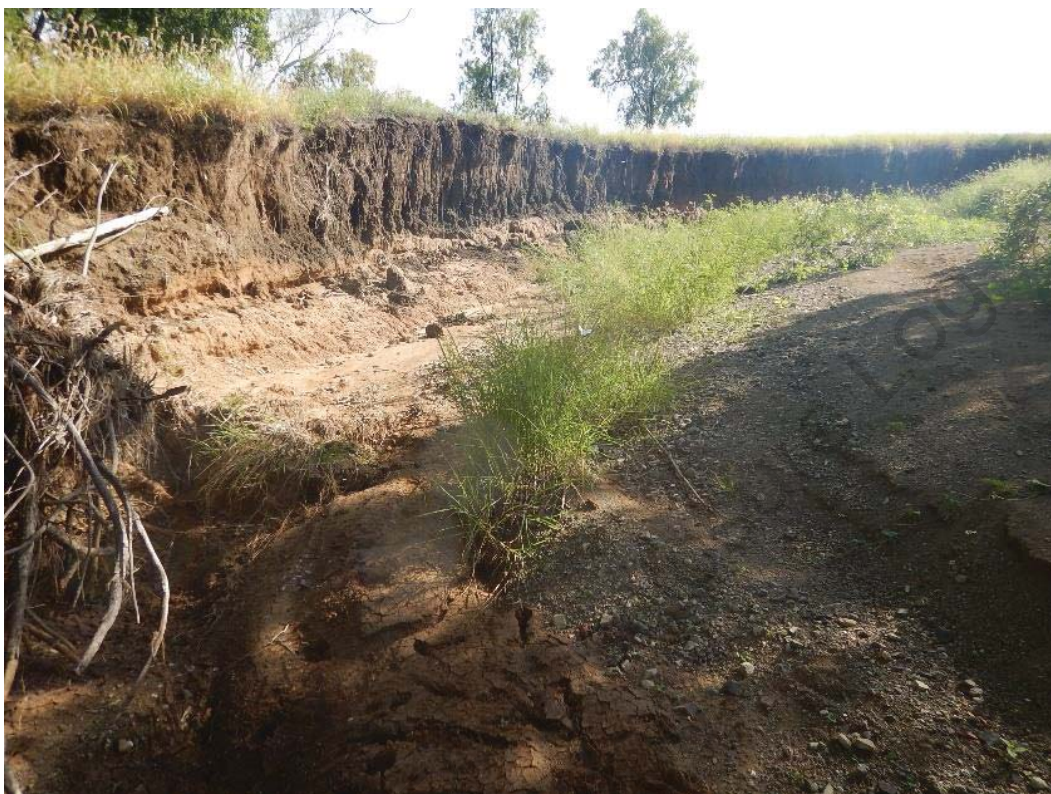
Figure 6.4 Bank Erosion Upstream Of TMC-US4
