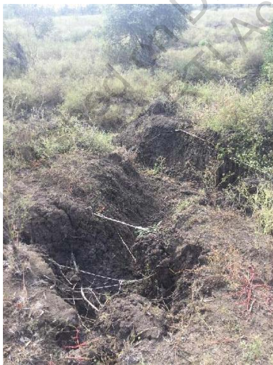
Figure 6.31 Gully Erosion On Right Bank Downstream Of TMC-DS3
