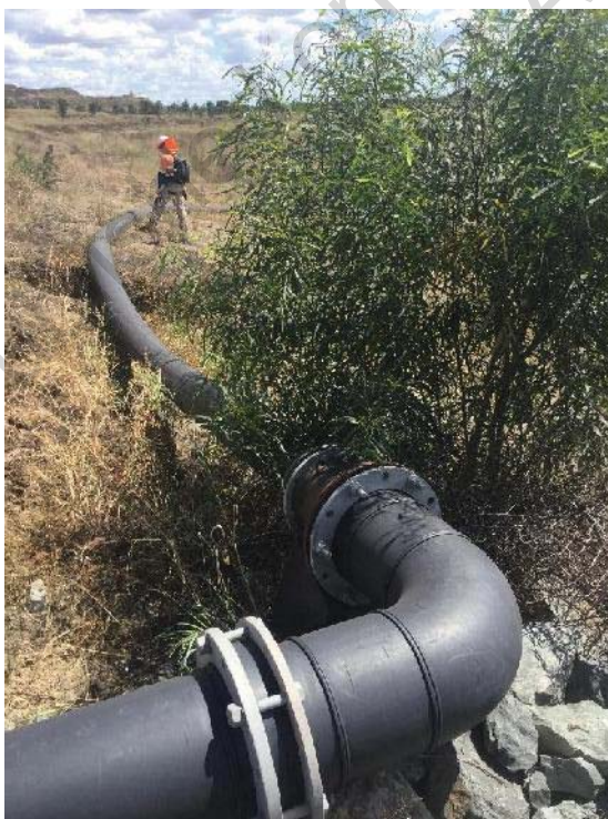
Figure 6.18 Vegetation Establishment At Location Of Previous Scour At Outlet Of Sd5 Gravity Discharge Pipe
