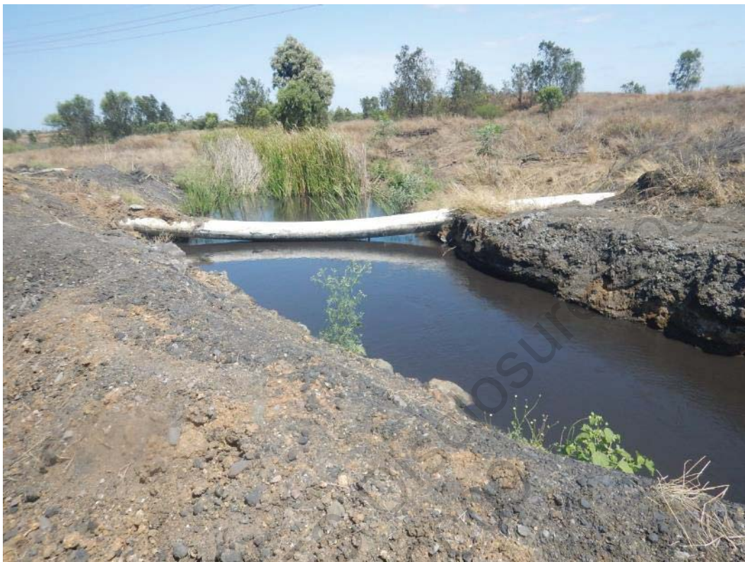
Photo 15 Eastern Solution Trench Upstream of Outlet into Return Water Dam
