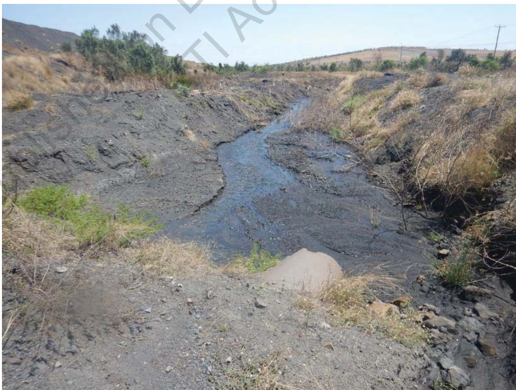
Photo 12 Eastern Solution Trench and Eastern Wall of Cell 1
