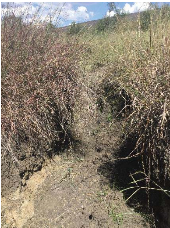
Figure 6.21 Upstream Limit Of Erosion Gully (View Towards SD5 And MIA)
