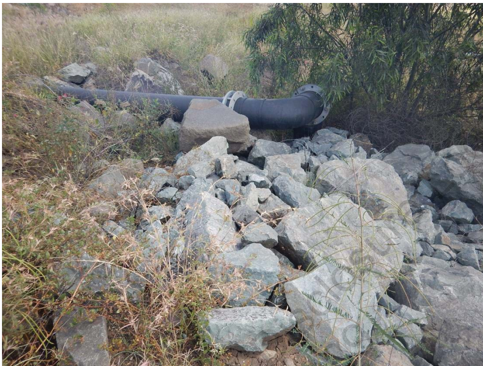
Figure 6.17 Vegetation Establishment at Location of Previous Scour at Outlet of SD5 Gravity Discharge Pipe
