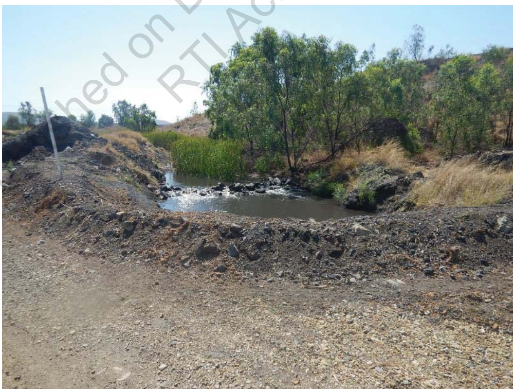
Photo 14 De-silted Channel at Downstream End of Eastern Solution Trench
