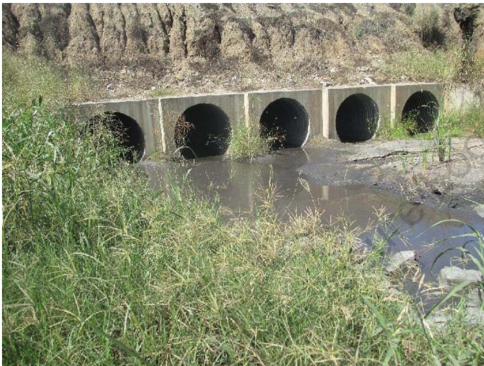
Figure 6.13 Downstream Headwall Of Low Level Haul Road Culverts
