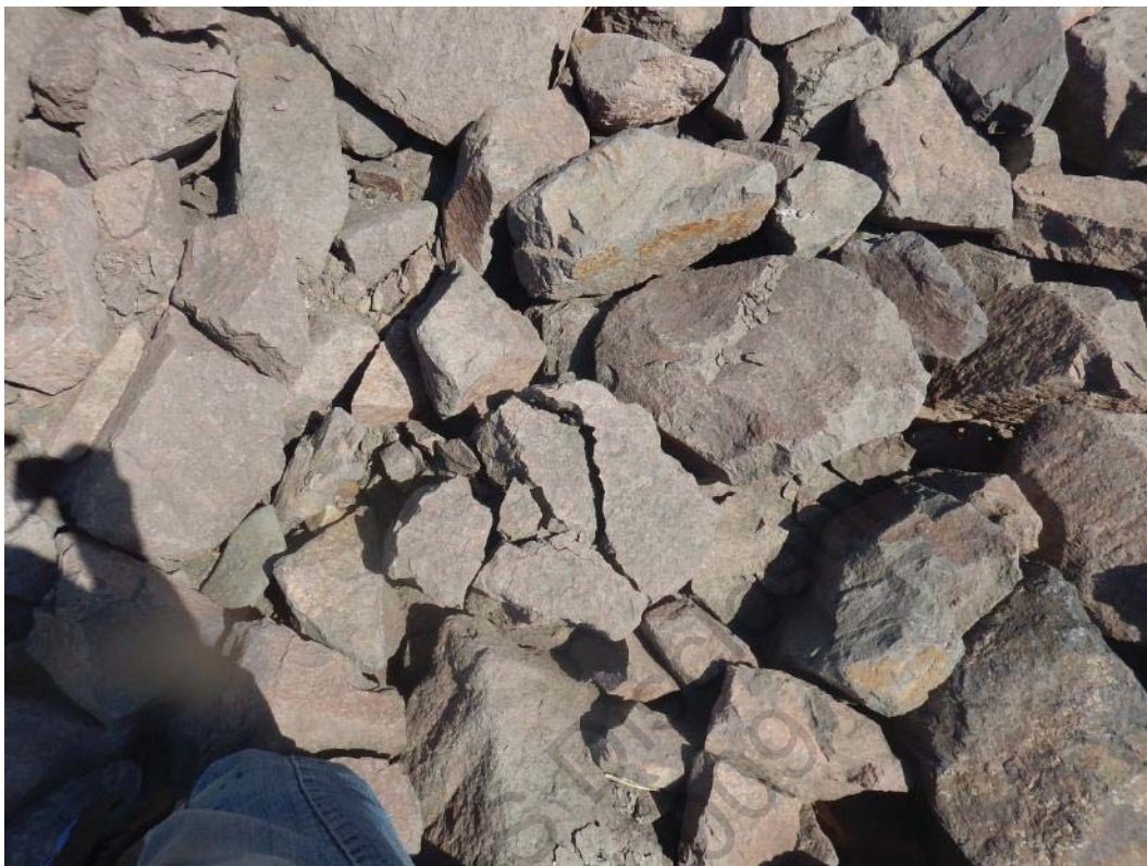
Photo 5 Rock Surface Treatment on Upstream Side of Plug
