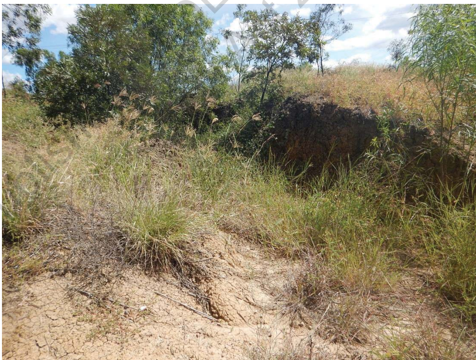
Figure 6.20 Secondary Smaller Erosion Gully Near Light Vehicle Road Crossing
