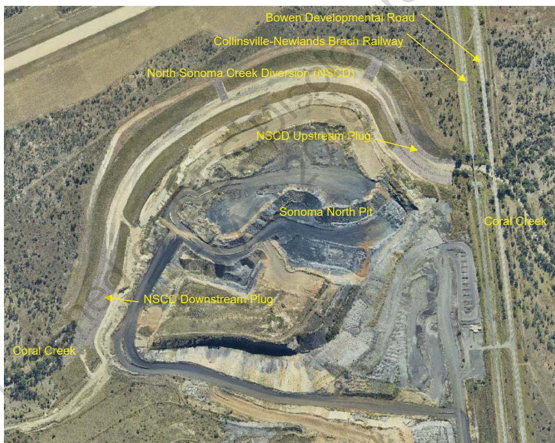
Figure 5.1 Aerial image of NSCD including Upstream and Downstream Plugs (aerial photo taken June 2019)
