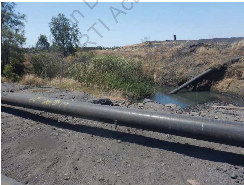
Photo 20 View Upstream Along Eastern Solution Trench from Road Crossing of Clean Water Drain and Eastern Solution Trench at North-Eastern Corner of Cell 3
