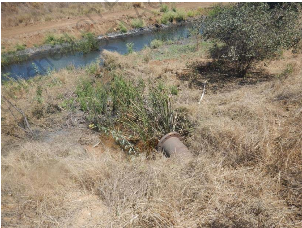
Photo 14 Discharge from Drainage Pipe Outlet into Western Solution Trench – Western Side of Cell 3
