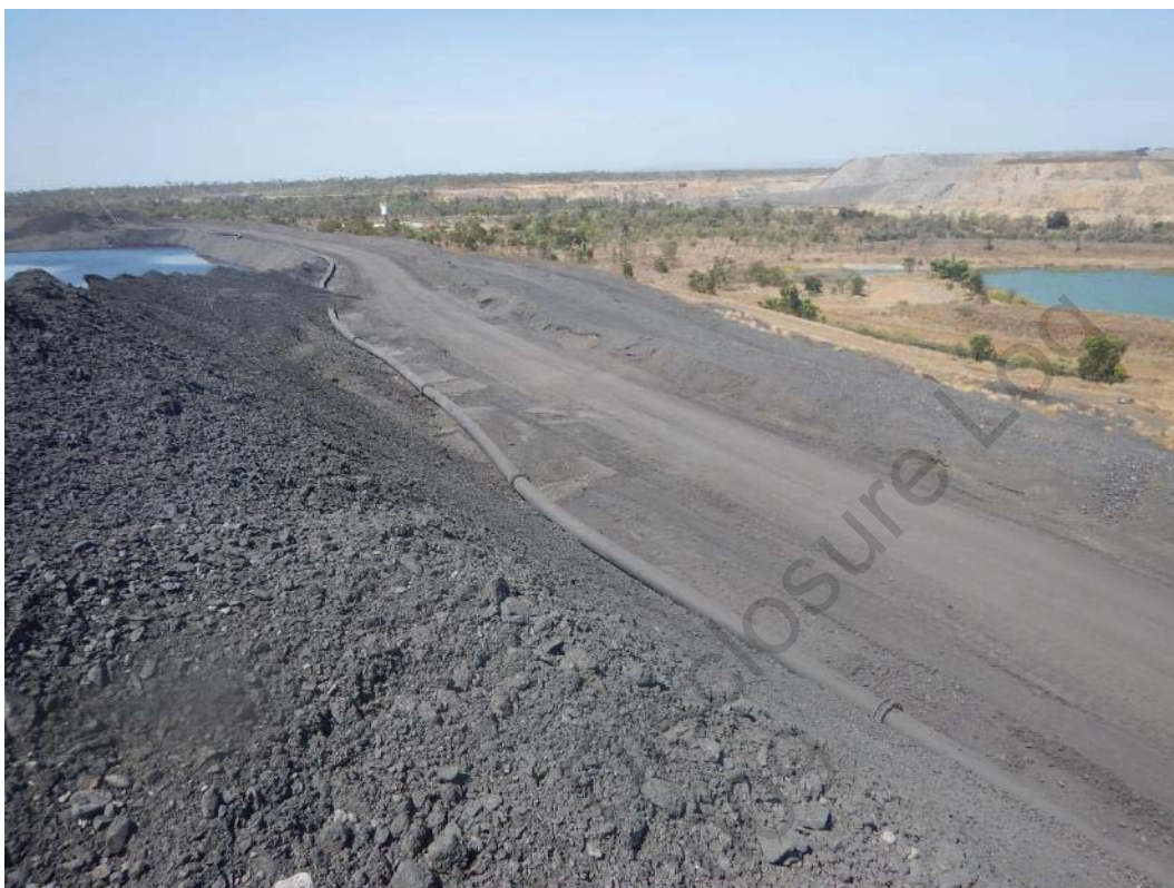
Photo 9 Western Side of Cell 3 Viewed from Top of Cell 3/4
