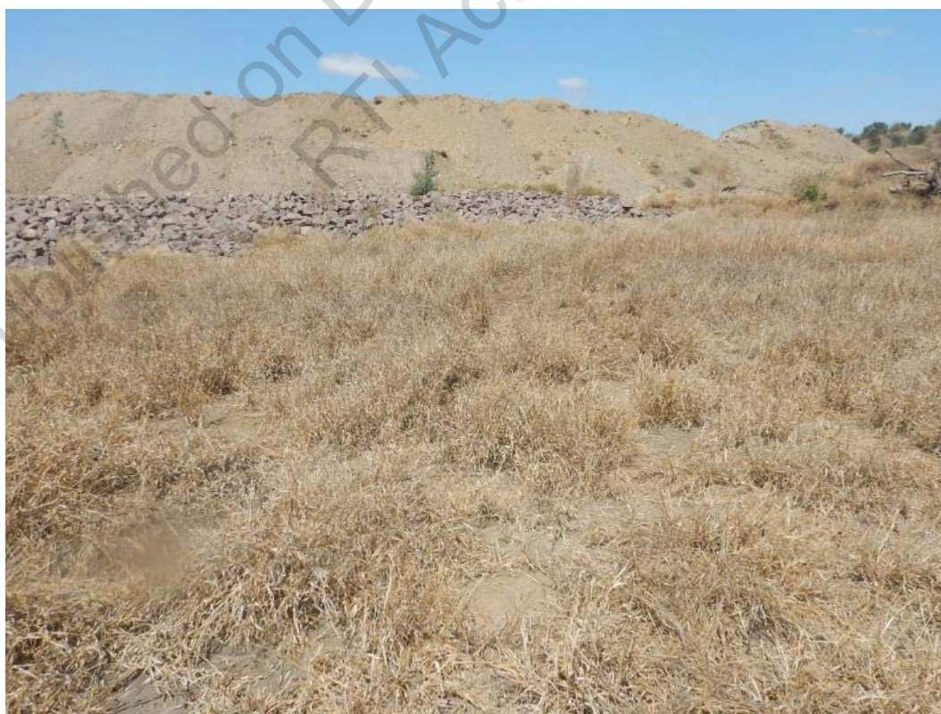
Photo 2 Upstream Side of Plug at Downstream End of Plug
