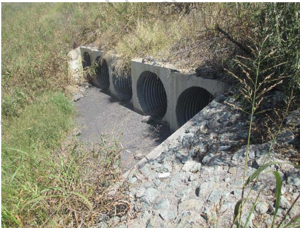
Figure 6.10 Low Flow Culverts At Upstream Side Of Haul Road
