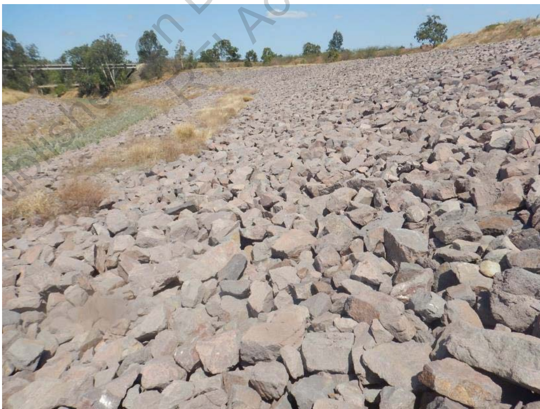
Photo 8 Upstream Side of Plug Viewed from Bench at Downstream End of Plug
