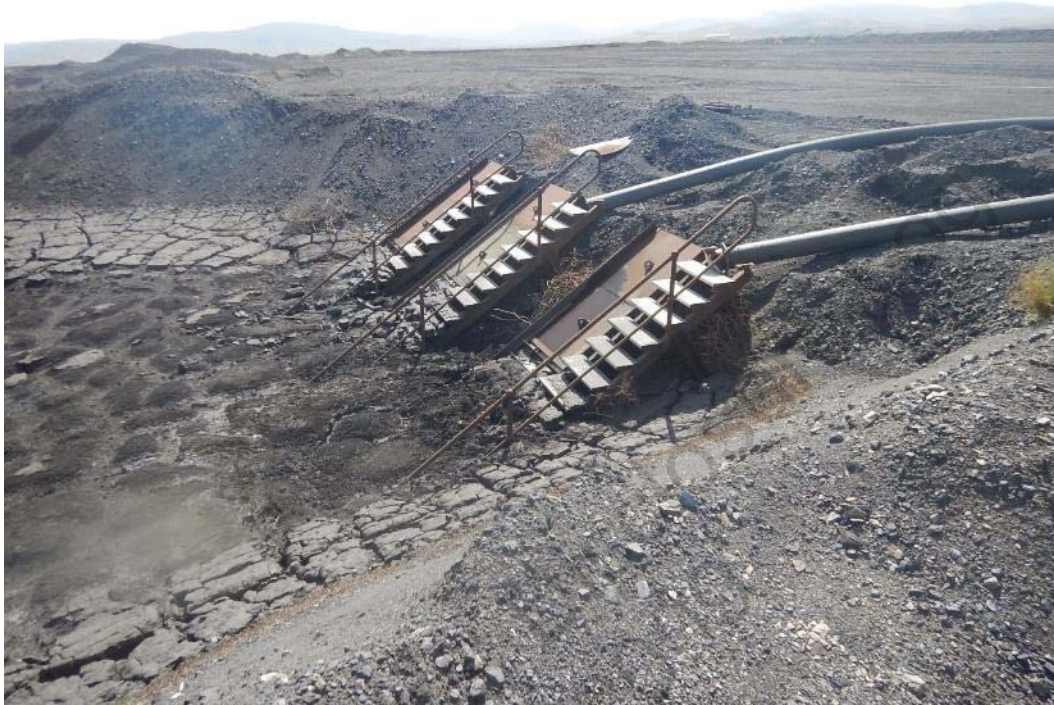
Photo 3 Decant Inlet Structure
