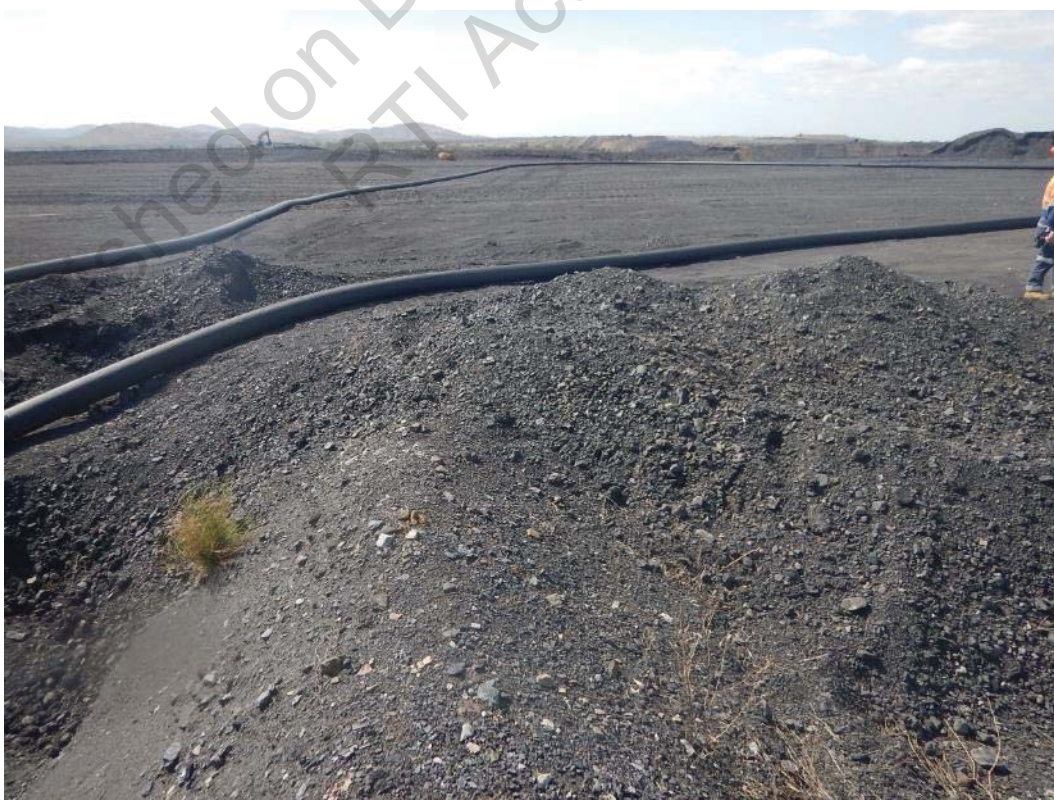
Photo 4 Re-shaping of Southern End of CDA1/2 to Form Overflow to Cell 3
