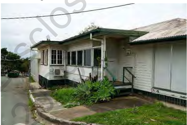
Building 6 with the added entry on the west— it is proposed to remove this later accretion and relocate this building marginally to the south
