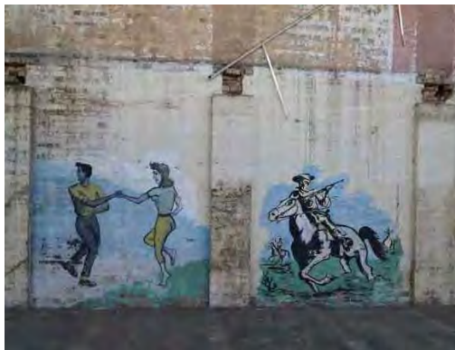
Building 2 the infilled opening in the northern wall (proposed to be re-opened), middle: the level difference and “gutter” at the western edge and RHS, the painted murals to be protected
