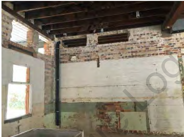
Building 1 southern wall with former openings to be infilled with contemporary windows and doors and RHS, smaller openings in early brickwork will be repaired with matching bricks and mortar
