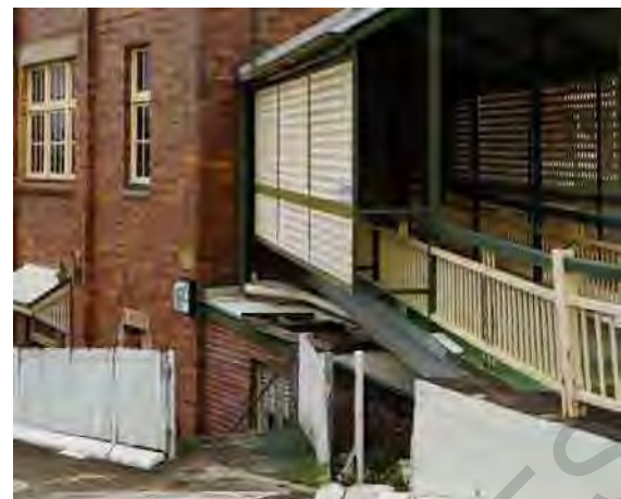
Building 1 with the later walkway to be demolished and ground lines lowered; note the fenced retaining wall to the adjoining driveway
