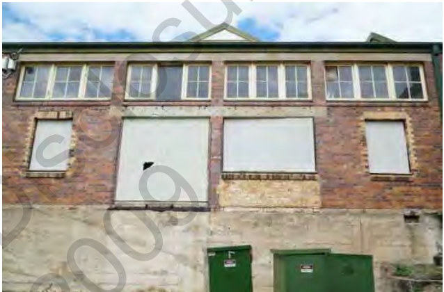
Building 3 from the east and north, temporary ply to be replaced with new glazed windows
