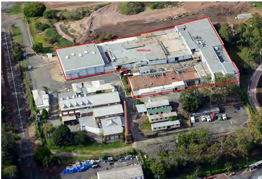
Aerial photo illustrating the extent of demolition (outlined in red) which was approved in April 2018. The roof additions to Building 6 are evident in this photo. The original building appears to have been a simple rectangular building with a hipped roof.
