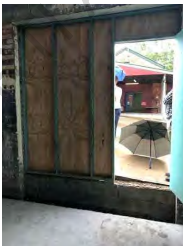
Building 2 the infilled opening in the northern wall (proposed to be re-opened), middle: the level difference and “gutter” at the western edge and RHS, the painted murals to be protected
