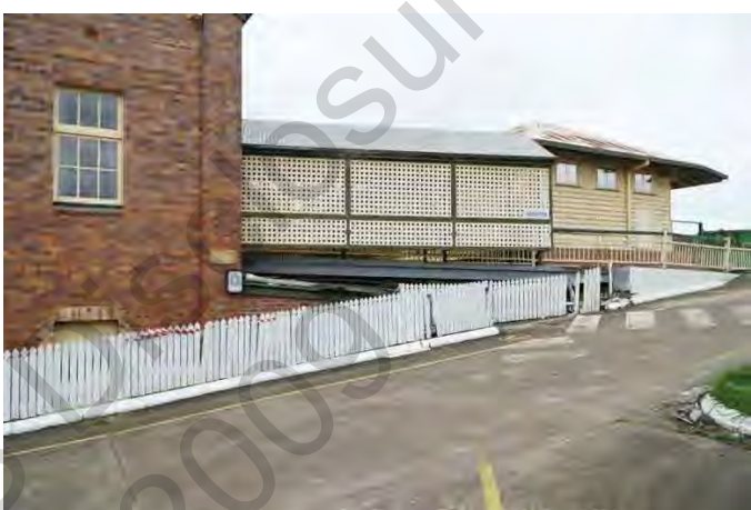
Building 1 with the later walkway to be demolished and ground lines lowered; note the fenced retaining wall to the adjoining driveway
