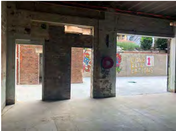
Building 1 southern wall with former openings to be infilled with contemporary windows and doors and RHS, smaller openings in early brickwork will be repaired with matching bricks and mortar
