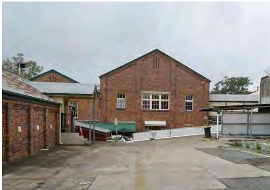
Building 1 from the west
