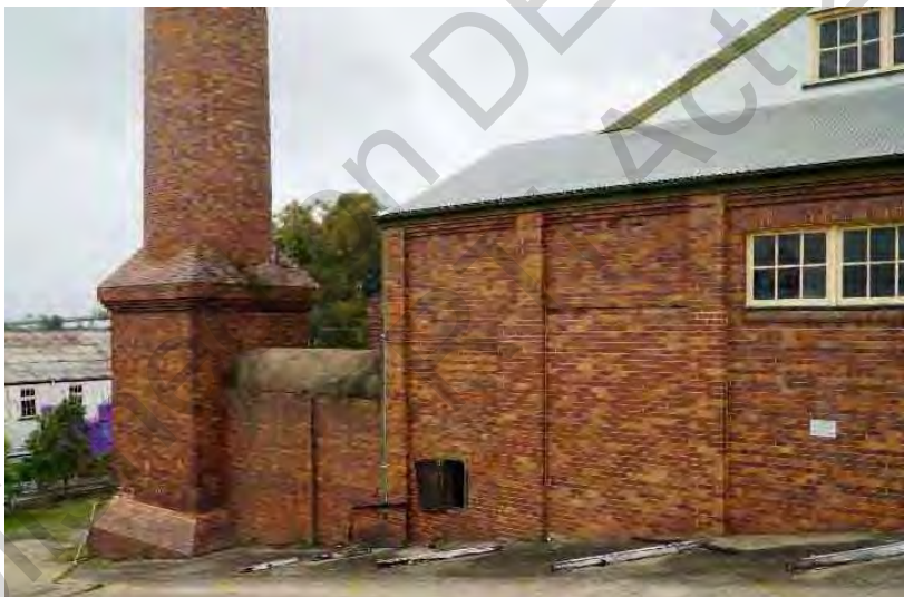
Building 3 west façade with later infill brickwork and RHS, infill from inside. Infill to be removed and new door B3.L1.08 inserted
