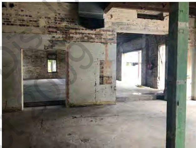
Northern wall of Building 1a and RHS, openings from Building 1a into 1b (to be infilled with rendered blockwork)
