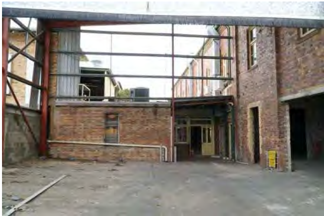
Building 5a at the lower level; openings to have new window and door inserted.
