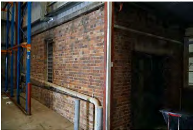
Building 5a at the lower level; openings to have new window and door inserted.
