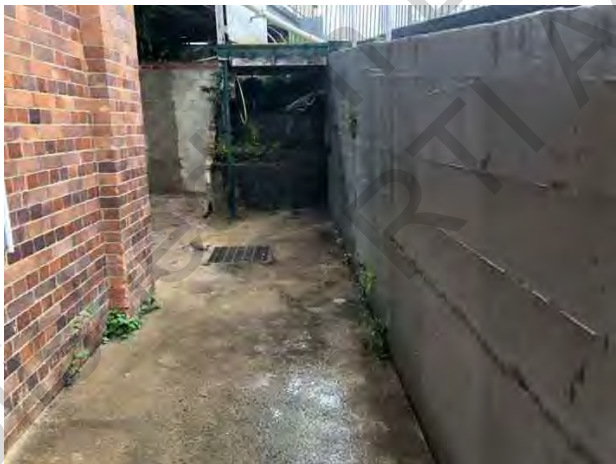
The existing retaining wall is later off form concrete
