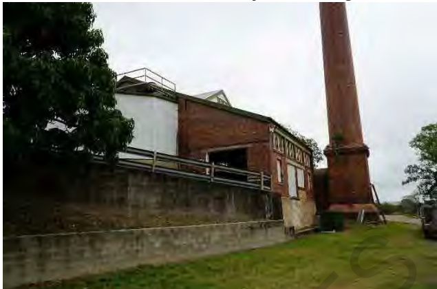
Building 3 from the east and north, temporary ply to be replaced with new glazed windows
