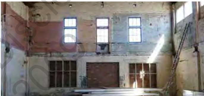
Later openings on the east to have a new infill door and windows; note that the timber frames are to be retained. The structural steel waler proposed will support the eastern and western brick walls along the line of the previous floor that has been removed. Note these photos were taken prior to the removal of the infill brickwork to the west (approved under previous EC)
