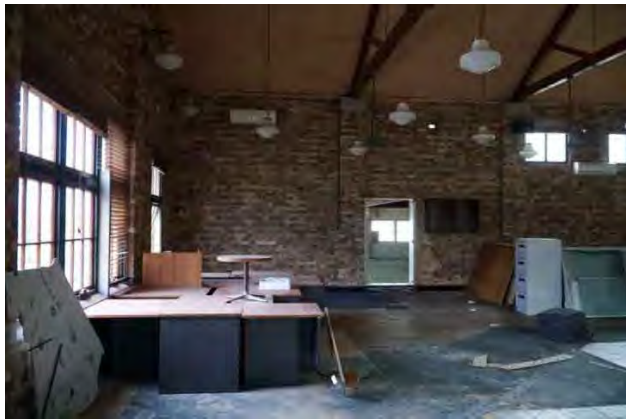
Northern wall of Building 1a and RHS, openings from Building 1a into 1b (to be infilled with rendered blockwork)
