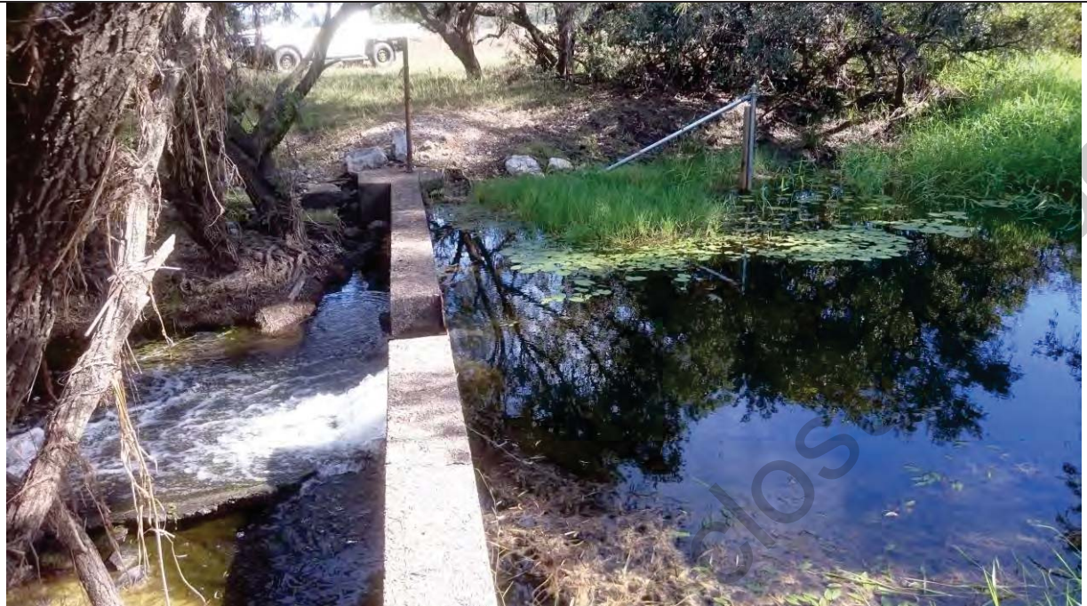
Photograph 3: Weir 7 on Larcom Creek – looking northward (refer to Figure 2 for the location of B21; Photograph taken on 5 June 2017).
