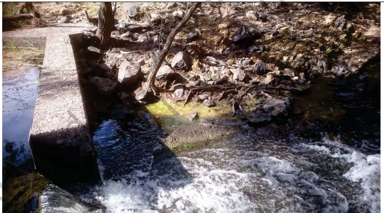
Photograph 4: Weir 7 on Larcom Creek – looking southward (refer to Figure 2 for the location of B21; Photograph taken on 5 June 2017).
