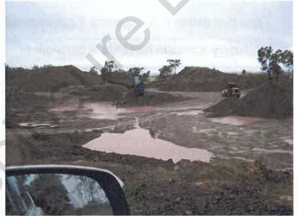
Koumala Quarry 4 – Sediment Drains
