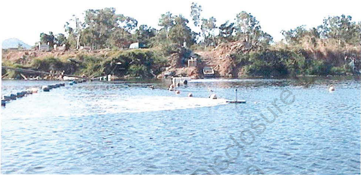
Plate 3 – Illustration showing the mechanical aerators.
