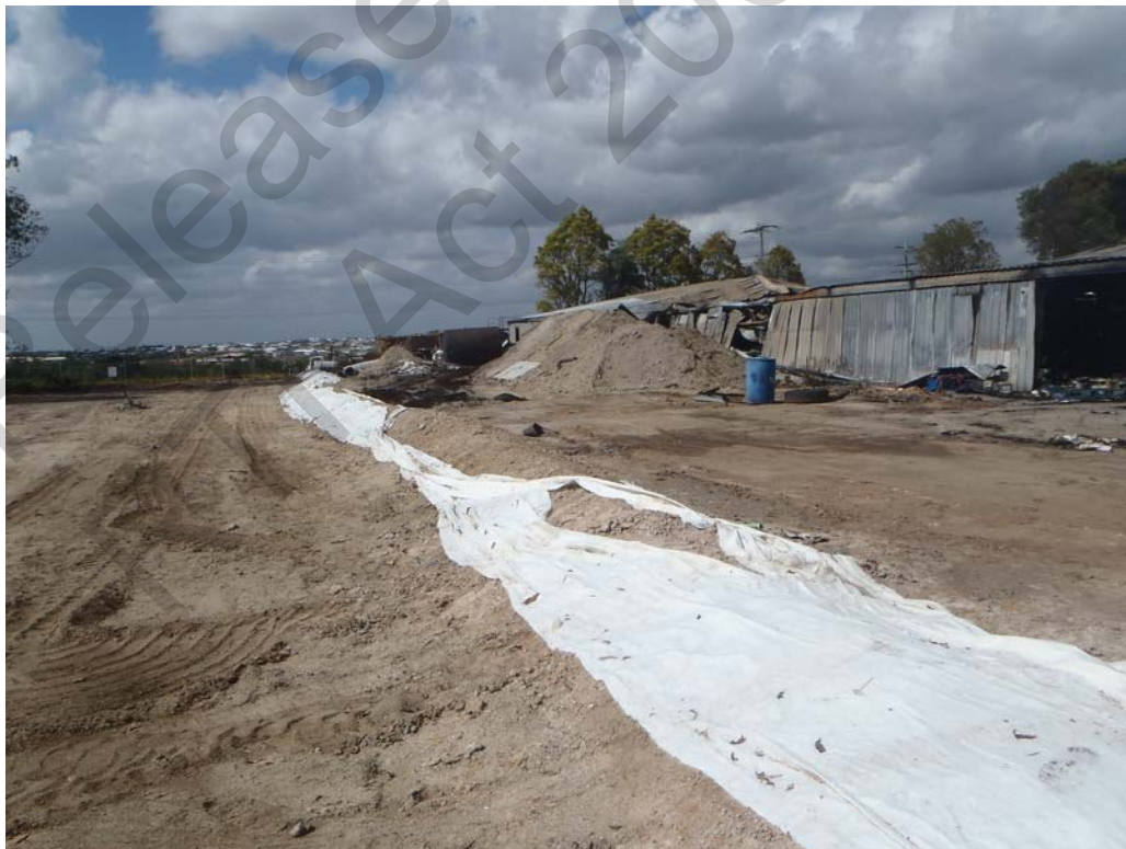
Photo 5 – The rear of the main building (facing south). No change from the site visit on 18 December 2012. Note some moisture on the ground, likely to be from rainfall.
