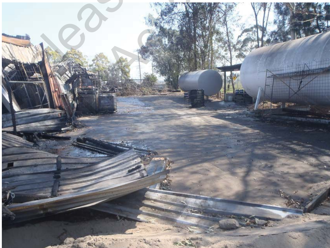
Photo 3 – This photo has been taken from the same location as photo 1 and 2 but facing south. Significant clean-up has occurred. Please note there is no contamination on the concrete.
