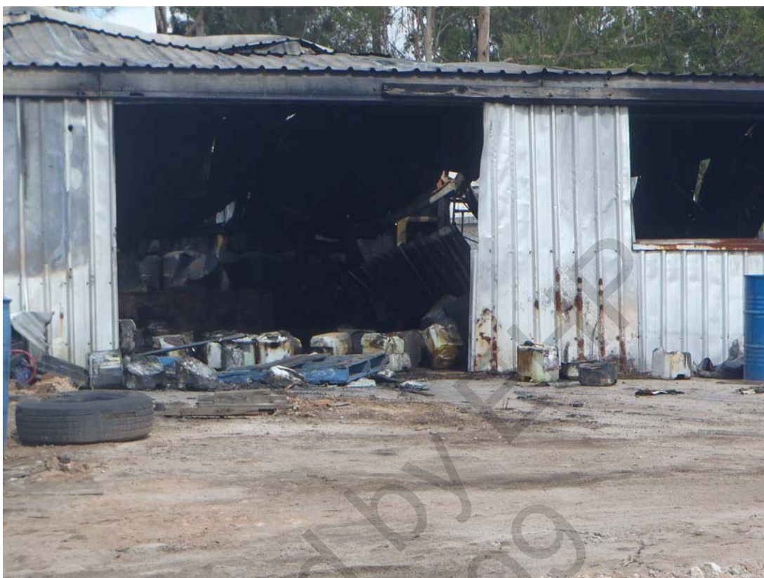
Photo 8 – Inside the main building from the rear of the property. No change from the site visit on 18 December 2012.
