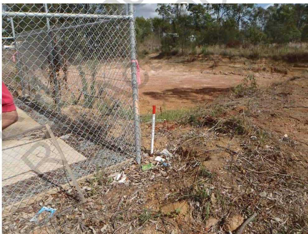
Photo 7 – The rear of the Telstra tower on the rear corner of the property. Note the white and red stake. This represents the boundary point from where DSDIP will construct a fence from towards boundary road.
