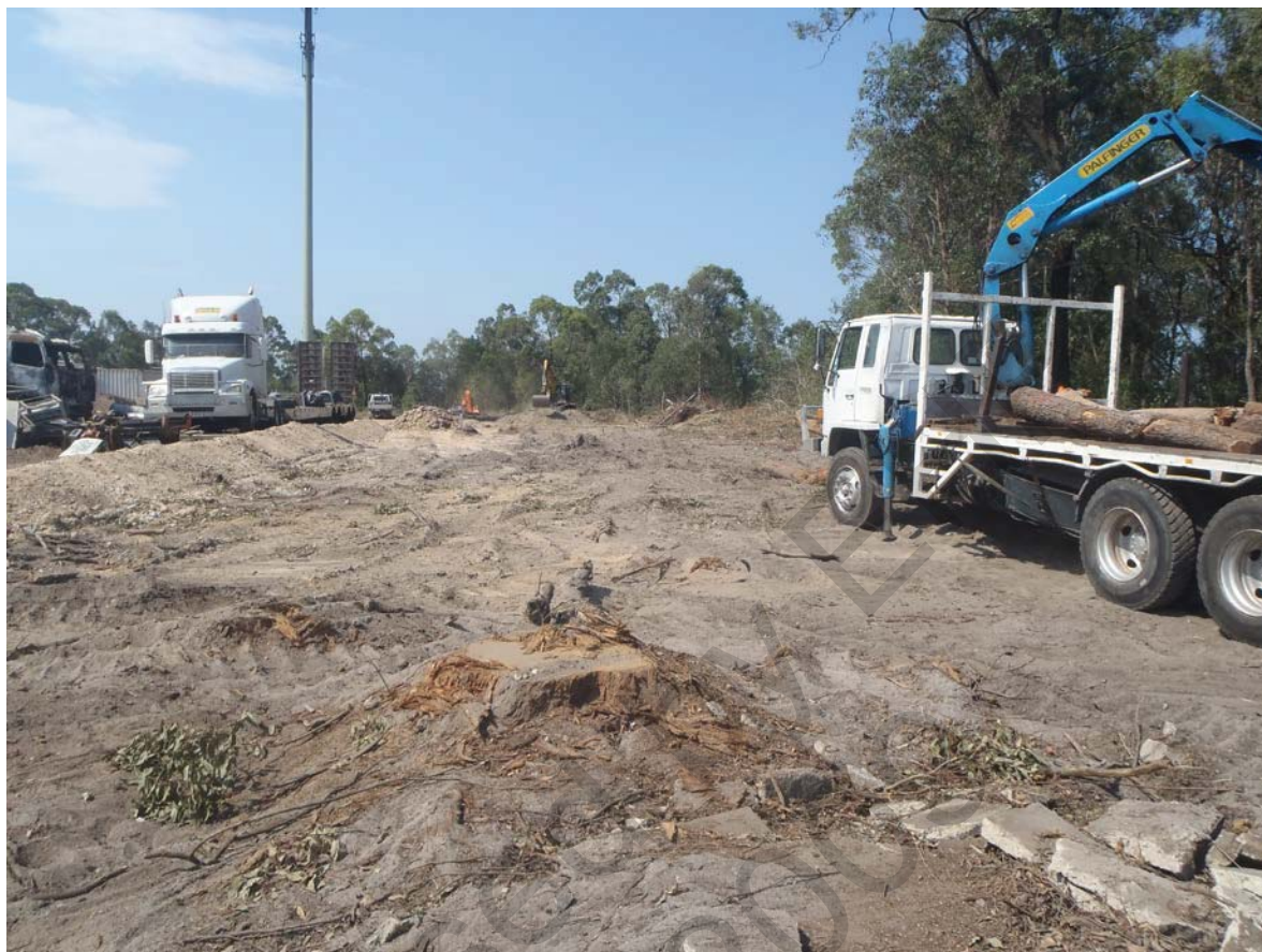
Photo 12 – This photo is taken from the site boundary along Boundary Road facing north. It shows the bund in place around the main building to the left and the remediation works by SDIDP on the right.
