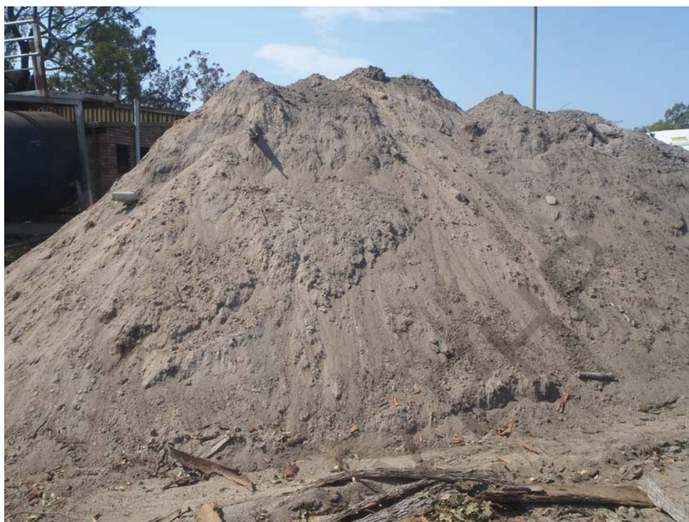
Photo 10 – The photo is taken from the rear of the site (behind the main building) towards the Boundary Road facing north west. Please note the large bund that has been placed around the building in the middle of the photo. This bund has been placed by SDIDP contractors to protect the adjacent state land from further contamination.
