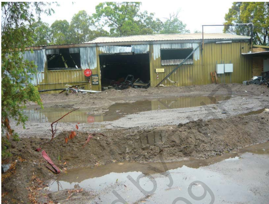
Photo 8 – Water pooling within the bunded area at the front of the southern end of the building (parallel to Potassium Street)
