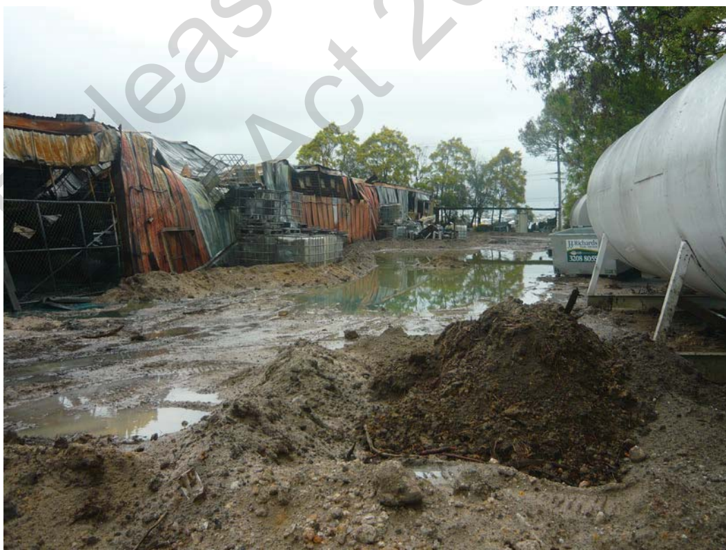
Photo 9 – Water pooling within the bunded area at the front of the building (photo is looking south from the northern end of the building – parallel to Potassium Street). Please note the blue sheen on the water indicating that contaminants are exiting the building due to the rainfall.
