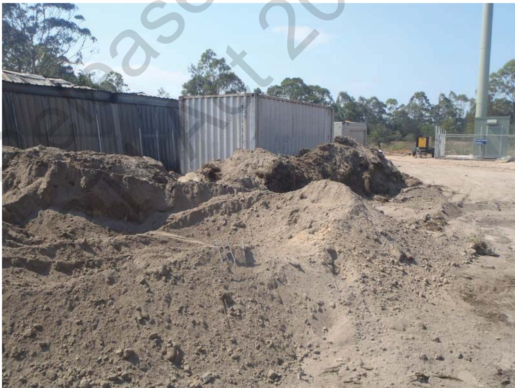
Photo 7 – The photo is taken from the rear of the site (behind the main building) towards the Boundary Road facing north west. Please note the large bund that has been placed around the building in the middle of the photo. This bund has been placed by SDIDP contractors to protect the adjacent state land from further contamination.
