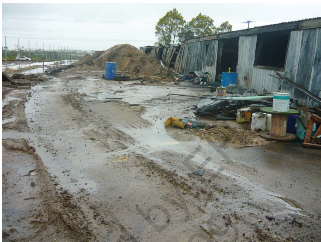
Photo 14 – The eastern side of the building. Please note no contaminants can be seen exiting the building on this side.
