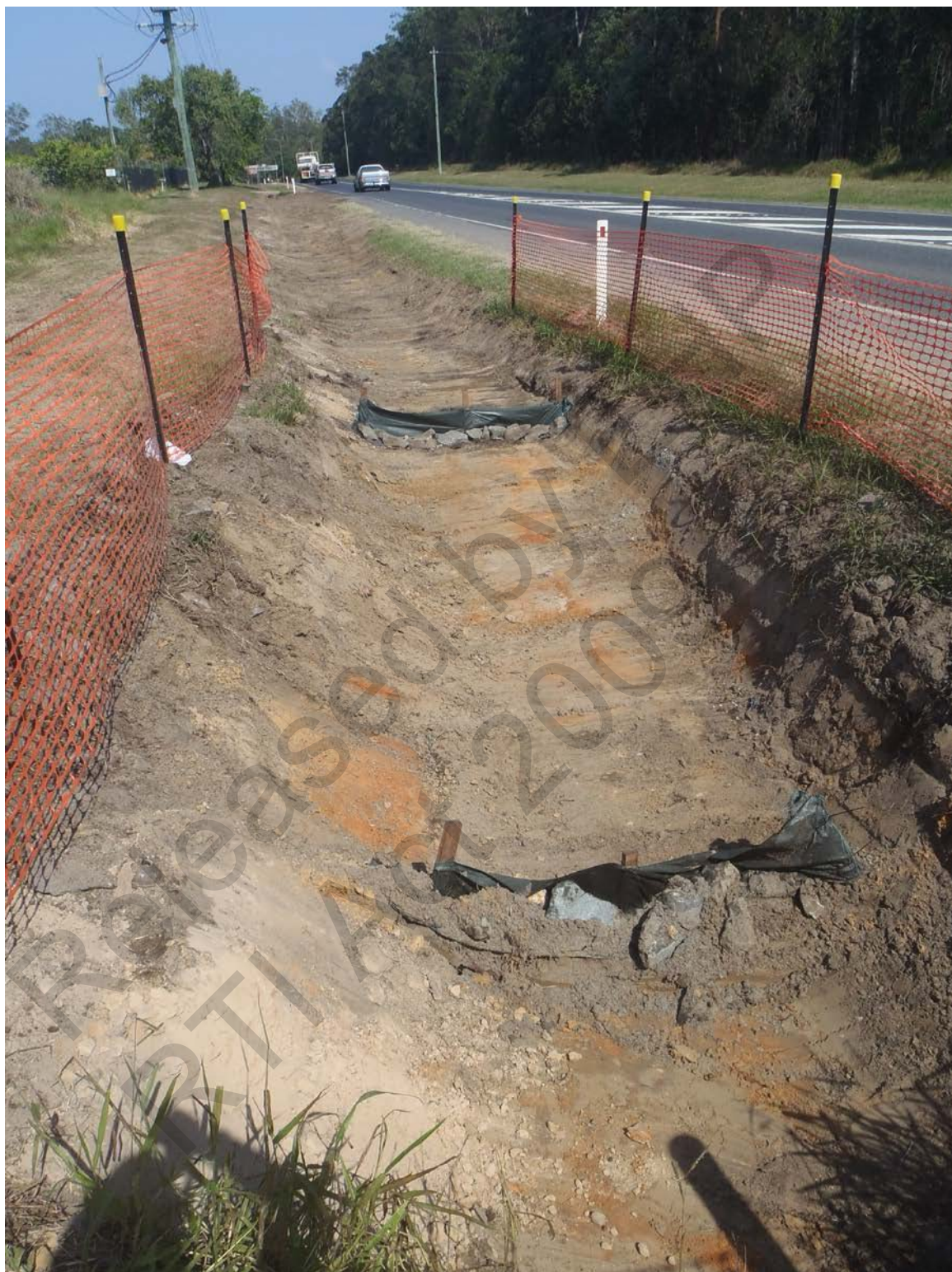
Photo 14 – This photo is taken where the concrete stormwater drain enters into a grass spoon drain approximately 200m done Boundary Road. Please note the remediation works completed by MBRC. This includes digging out the contaminated parts of the drain and installing sediment fences in the drain.
