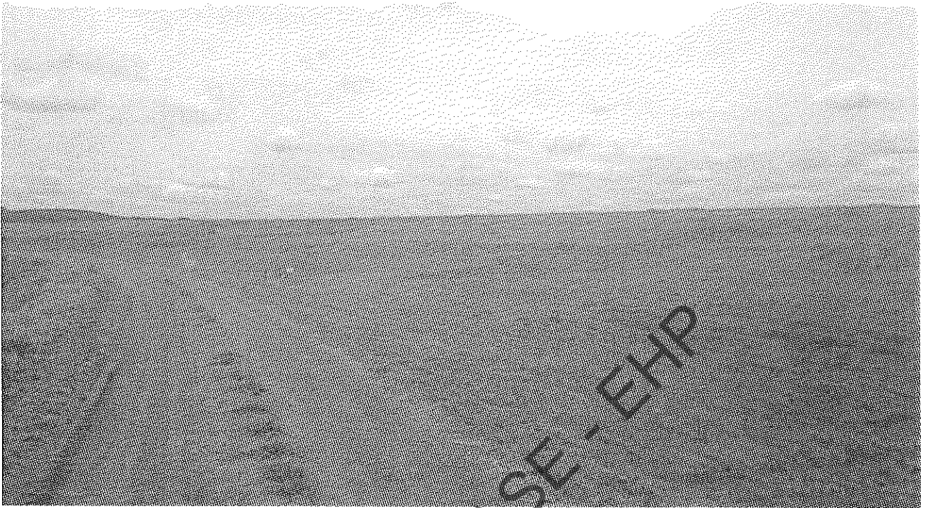
Photo 3. Capped and grassed area of ash storage area.
