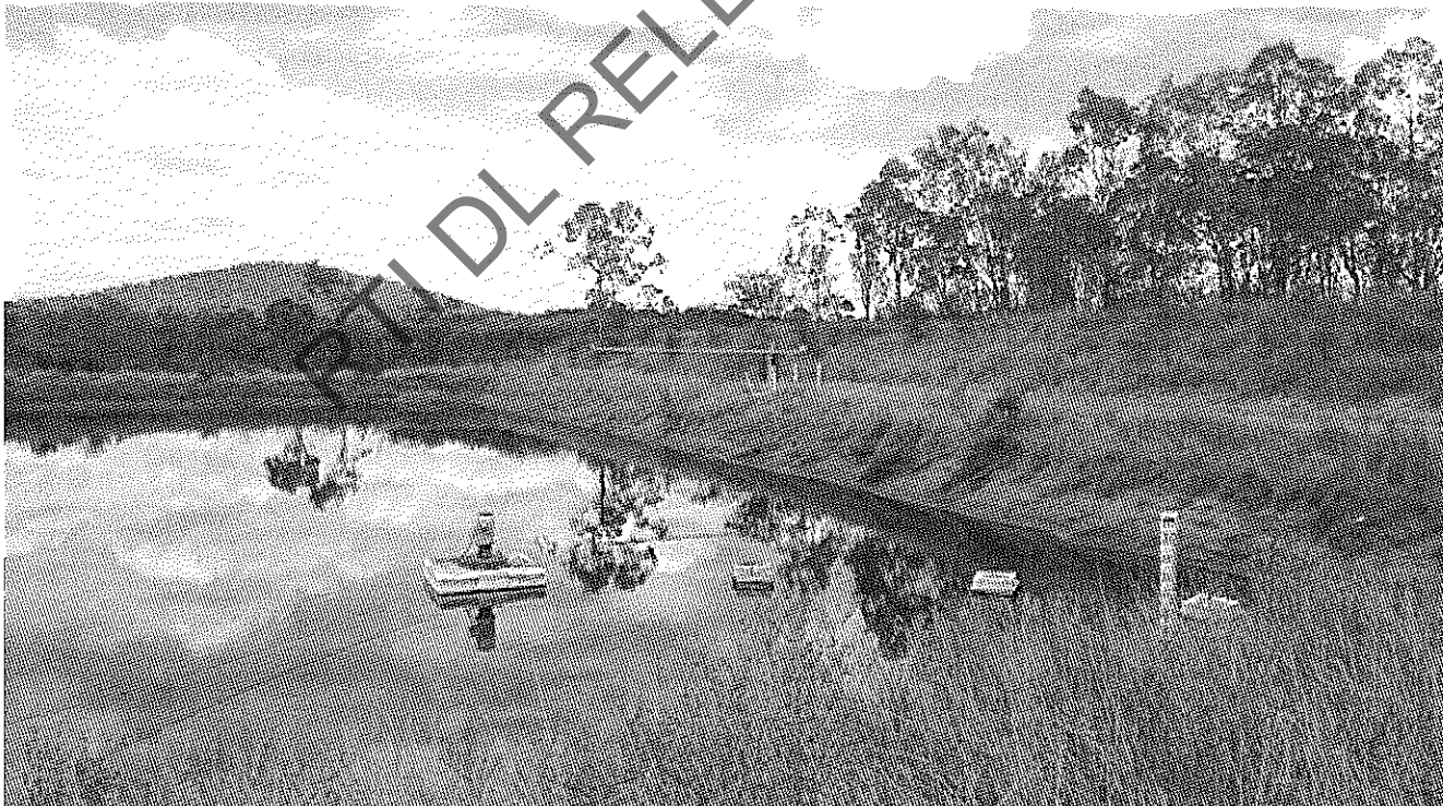
Photo 2. Coal Stockpile Runoff Pond. Pump visible floating on surface and ultrasonic height recorder in background.
