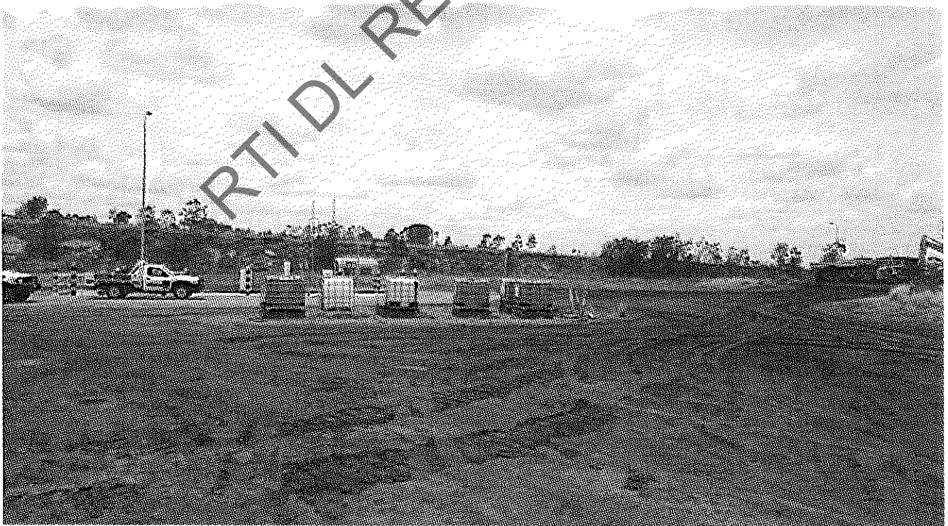
Photo 4. Vehicle fuelling point within coal stockpile catchment. IBCs individually bunded.
