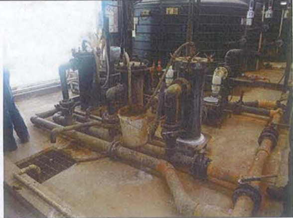
Picture 7-Inline filters for receiving of SSAA precursor materials
