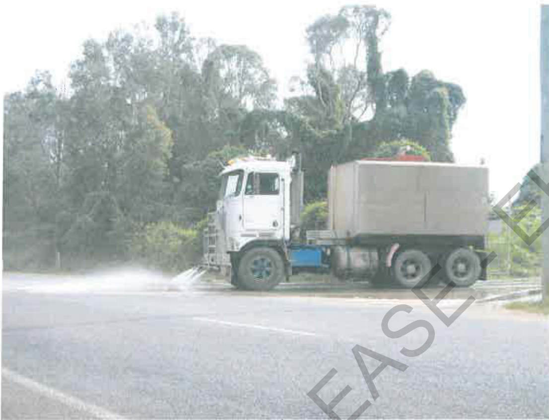
Figure 1 – Sediment being washed onto Pimpama-Jacobs Well Road Entry Point 2 (see map below)
