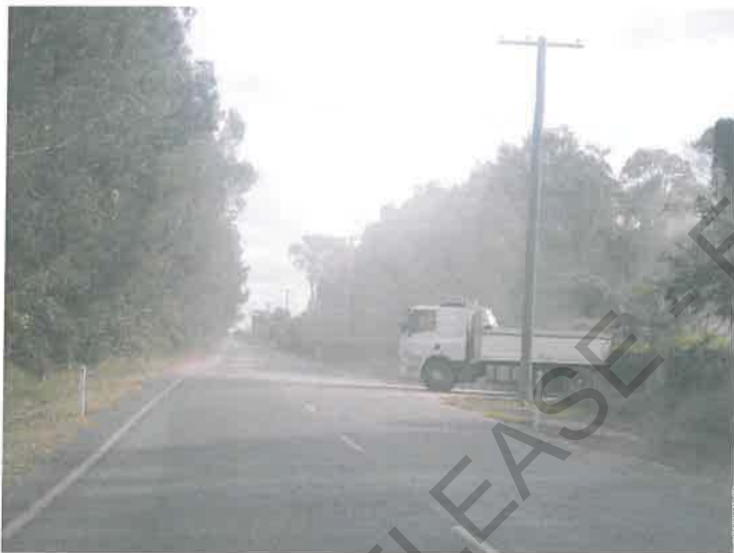
Figure 4 – Sediment on Road at Pimpama-Jacobs Well Road Entry Point 2 (see map below)
