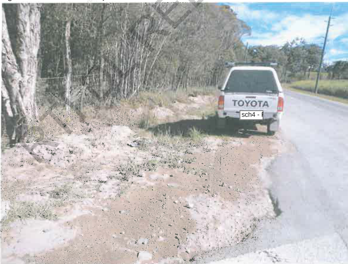
Figure 6 – sediment in gutter adjacent to waragap entry/exit point on Behms Road
