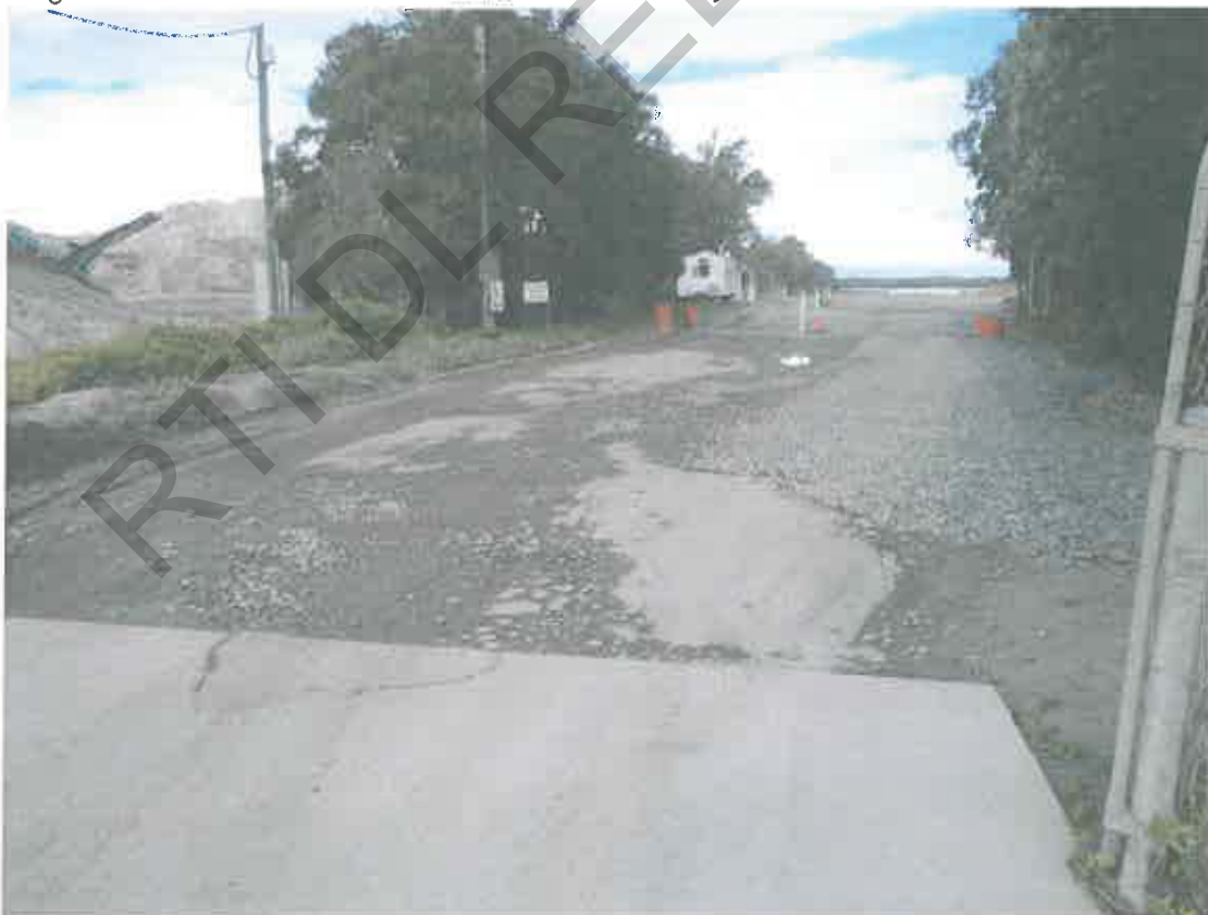
Figure 6 – Sediment on roadside at Behms Road entry/exit
