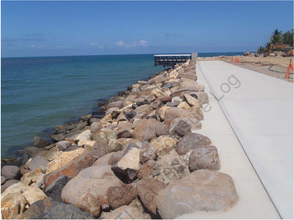
Seawall eastern end
