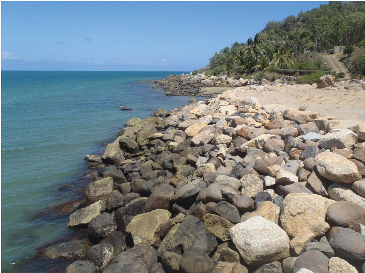
Seawall eastern end
