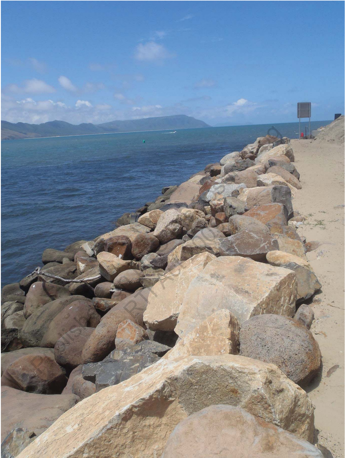
Seawall eastern end.
