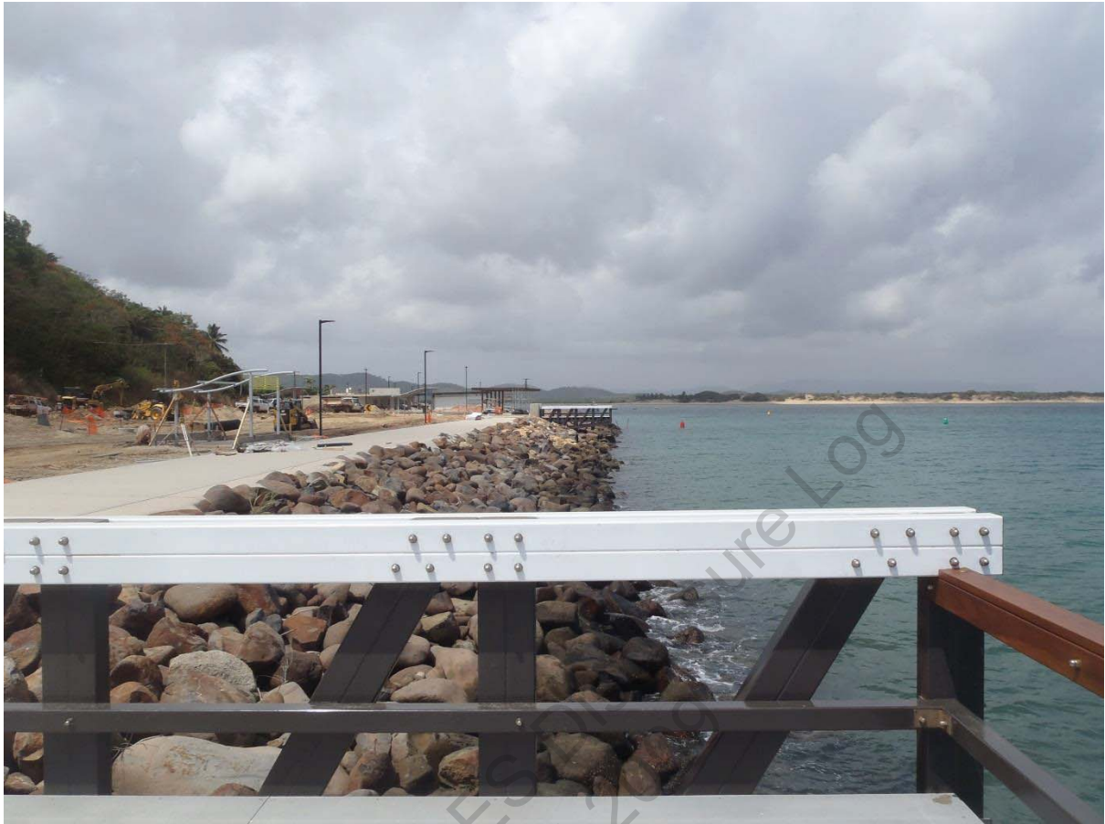
Seawall looking west
