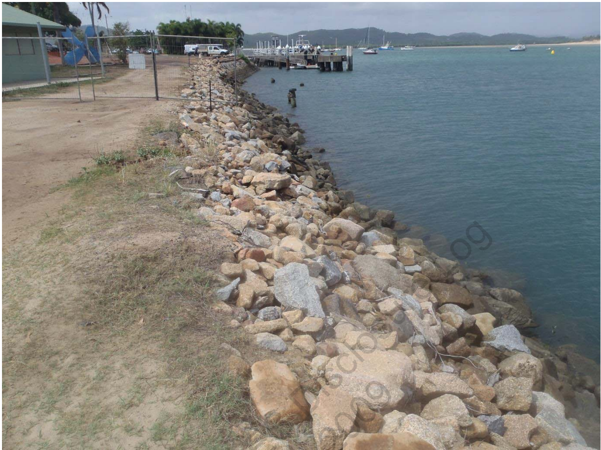
Seawall western end
