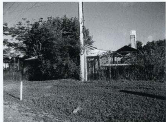
Photograph 4 - View of Workshops from Marara Street.
