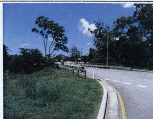
Photograph 4: Mary River Road/ Lower Mill Road intersection looking east towards Cooroy.
