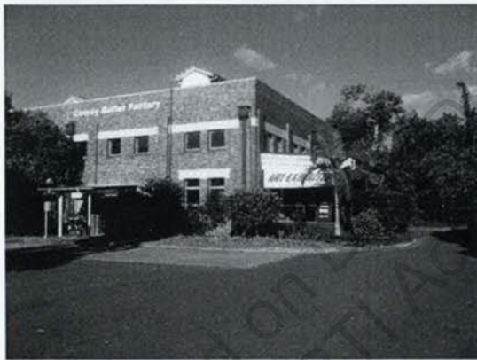
Photograph 1- Existing Butter Factory
