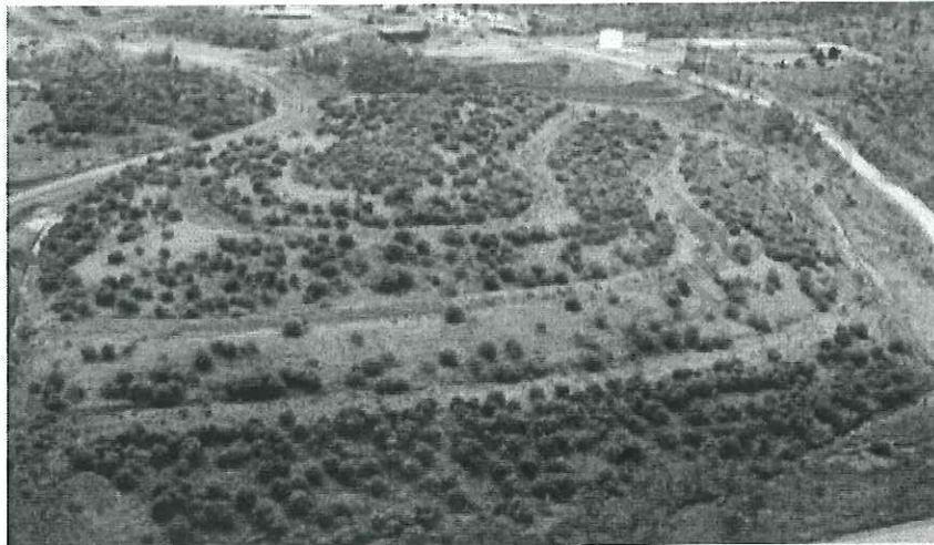
Figure 49 Example of a waste rock dump with catch berms installed.
