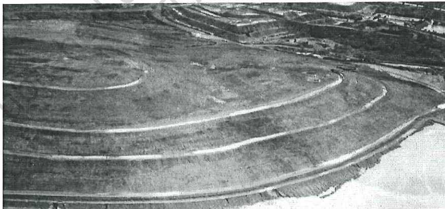
Figure 50 Example of a waste rock dump with recently installed graded banks.
