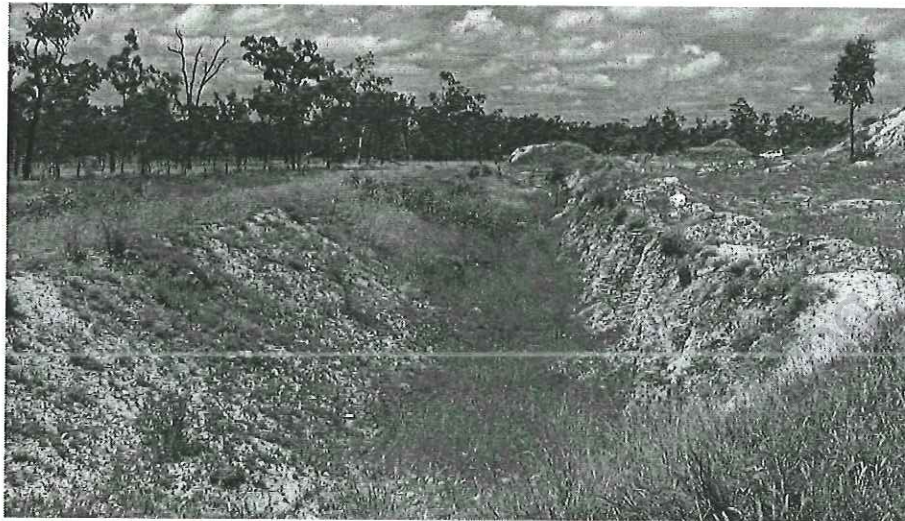
Figure 17 Broad shallow costean left open for a extended period of time
