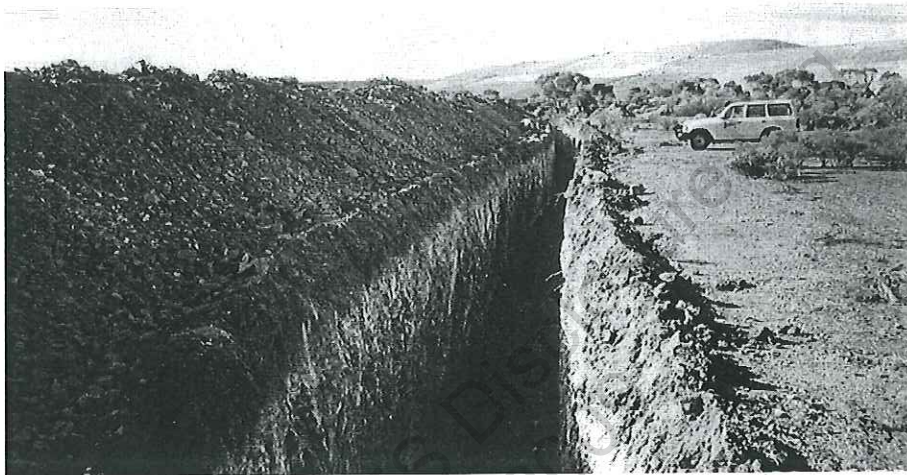
Figure 15 Example of a large costean - costeans of this size are a significant safety hazard.
