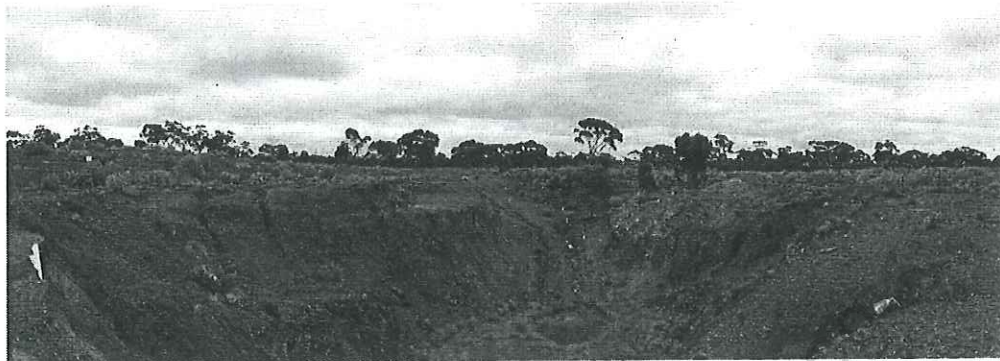
Figure 37 Example of shallow open pit with unstable batters and no bunding
