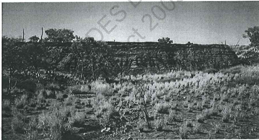
Figure 43 Old Valley Fill Tailings Dam with wall made from coarse tailings
