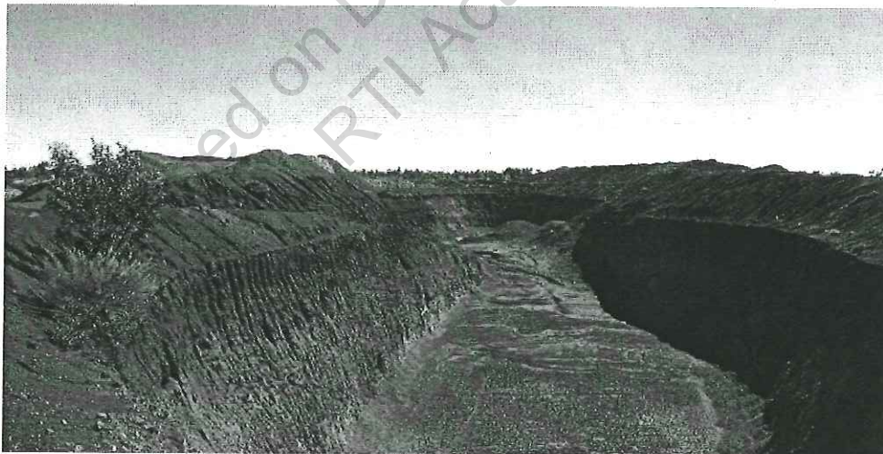
Figure 36 Example of shallow open pit with potentially unstable batters and incorrect bunding
