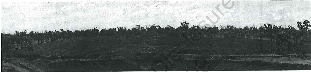
Figure 28 Example of moderate sized WRD after initial reshaping - prior to final works & revegetation
