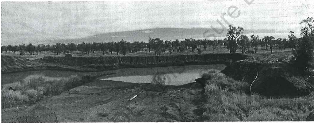
Figure 40 Dam with walls construct from material borrowed from the floor
