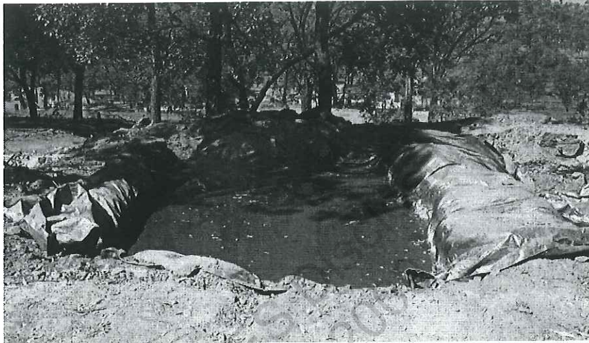
Figure 18 Example of an exploration drill sump using a plastic liner (photo: Qld EPA)
