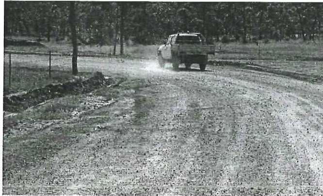
Figure 7 Moderate sized haulroad constructed without imported fill
