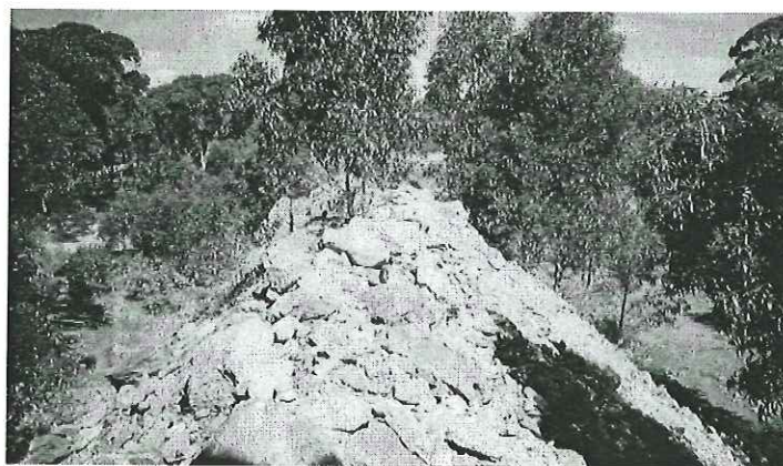
Figure 39 Example of a well constructed. Long-term stable pit bund
