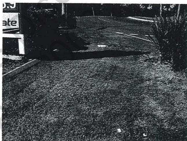
4. Energex excavation south east corner.
