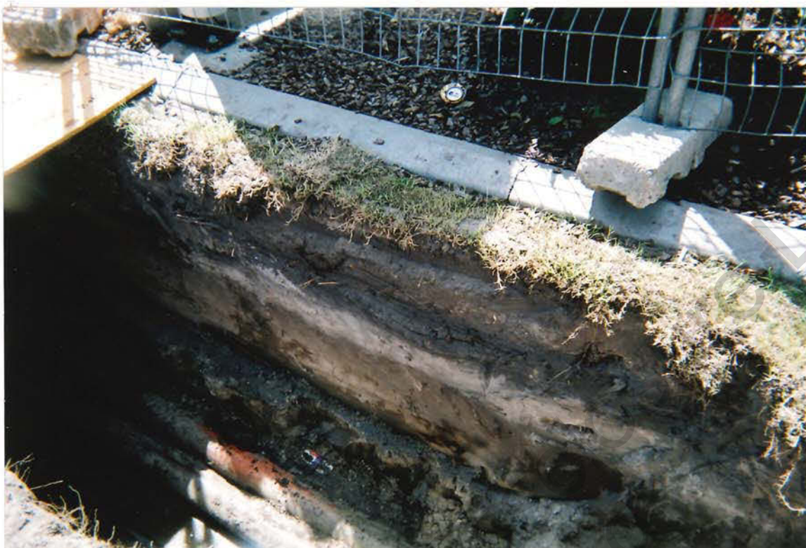
Photo 7 : 21/2/06 Energex pit on footpath Shows soil profile 0.1 - 0.4m Sandy silty topsoil (A horizon) 0.4m - 0.6m Silty sandy (B horizon), 0.6m - 1.5m sandy soil
