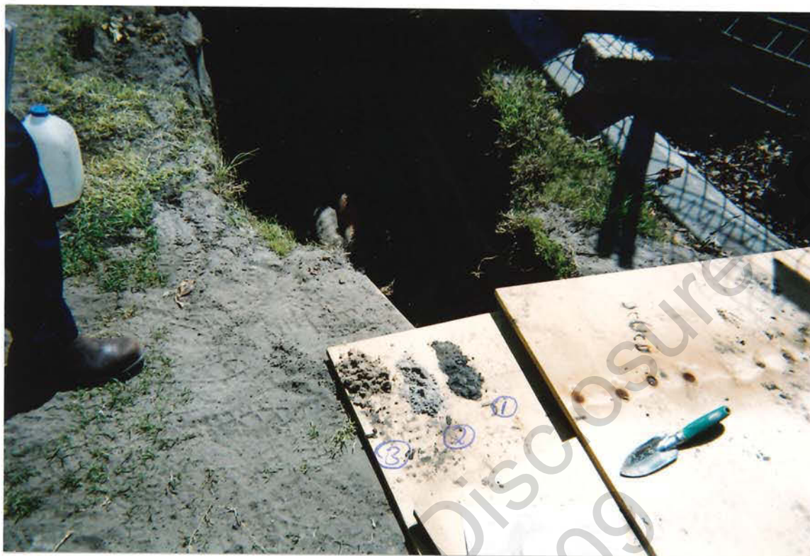
Photo 9 : 21/2/06. Three distinct soil types identified ① 0.1 - 0.4m Sandy silt/clay ② 0.4 - 0.6m Silty sand ③ 0.6 - 1.5m Sand
