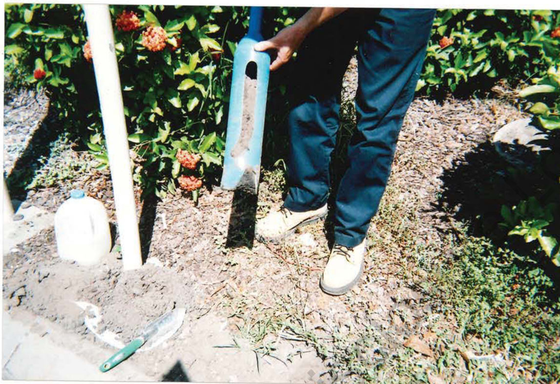
Photo 11: Borehole hand augered 2/2/06 near vent pipes in BP Mary St. garden bed. Visible staining & hydrocarbon odors @ 1m depth for sample ID TP005.
