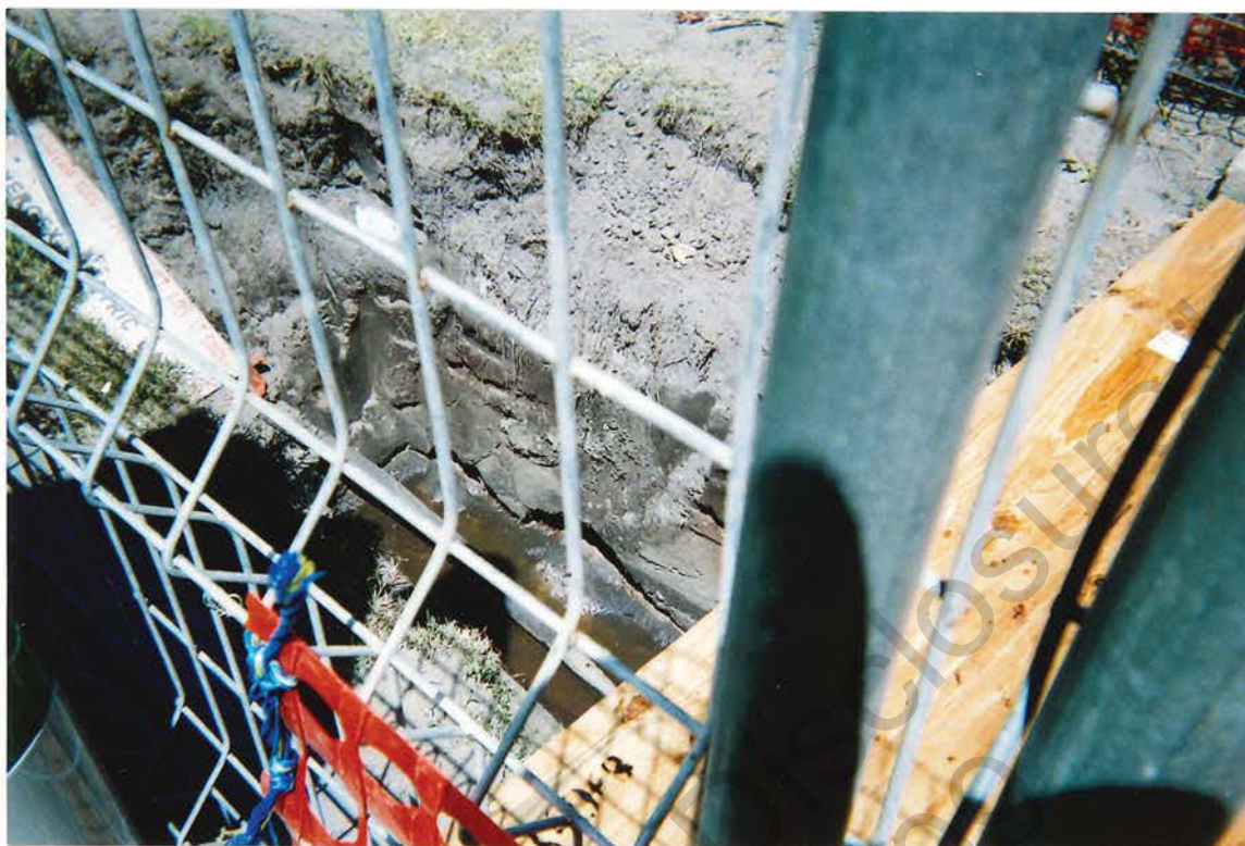
Photo 5 : 21/2/06 groundwater in lease of Energex pit @ 1.5m depth.
