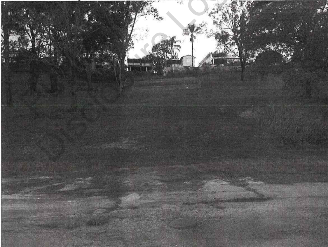
Site Photo 6 – Looking Upslope towards Sinkhole Area – Note Sandy Silt At Base of Hillslope
