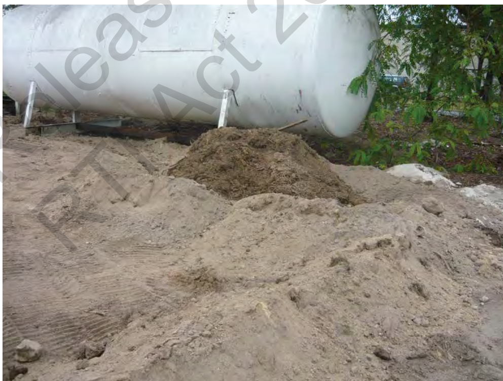
Photo 2 – Photo taken in the same location as photo 1. Looking more south east. Note that the existing bunding has been reinforced with further material. The pile in the centre of the photo is the contaminated soil which was scrapped off the Stockland land after the minor contamination incident on Tuesday. It is expected that this soil will be remediated as per the plan of operations.
