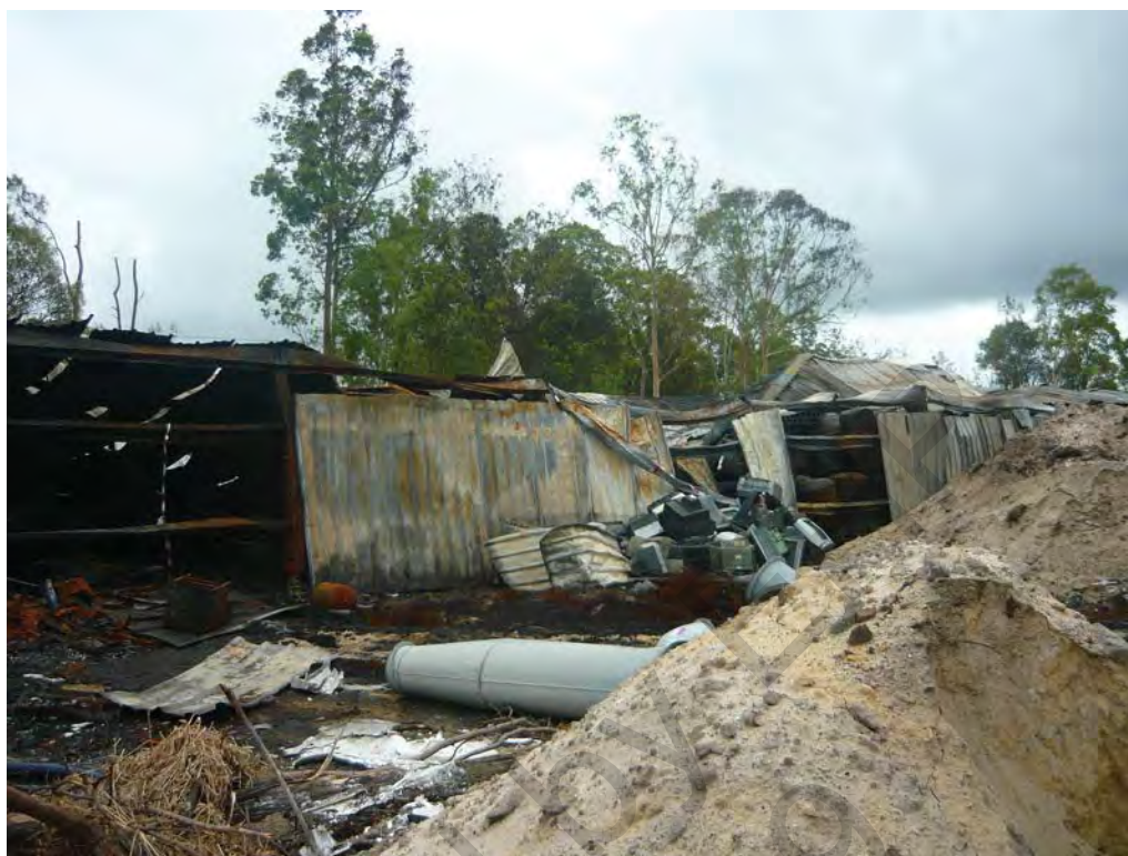
Photo 3 – The rear of the main building (facing north-west). No change from the site visit on 16 January 2013.
