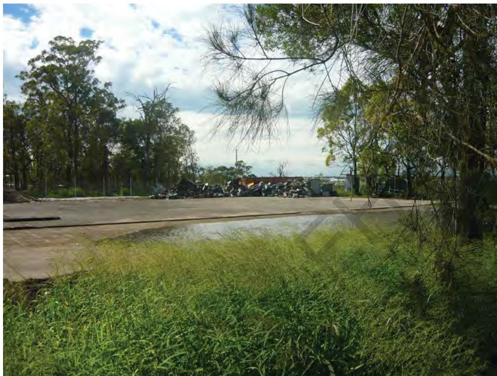
Photo 2 – Photo taken in the same location as photo 1. Looking more south east. The stock piles of television picture tubes are still located onsite. JP to contact Peter Moffat regarding their removal.
