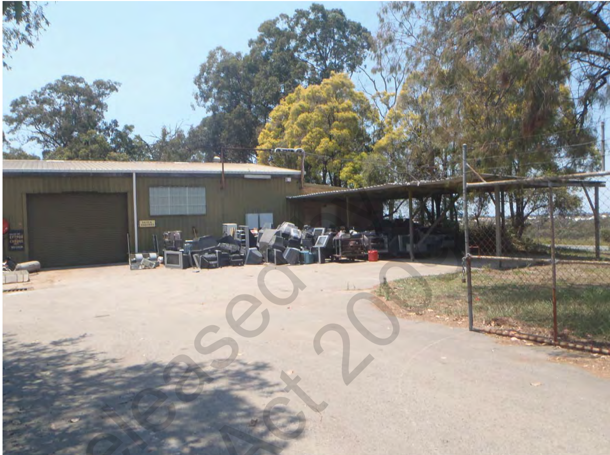
Photo 1 – Photo taken from Potassium Street looking at the southern end of the main building onsite. Note the large amount of tv's stored onsite. May indicate the operator is conducting a recycling service.
