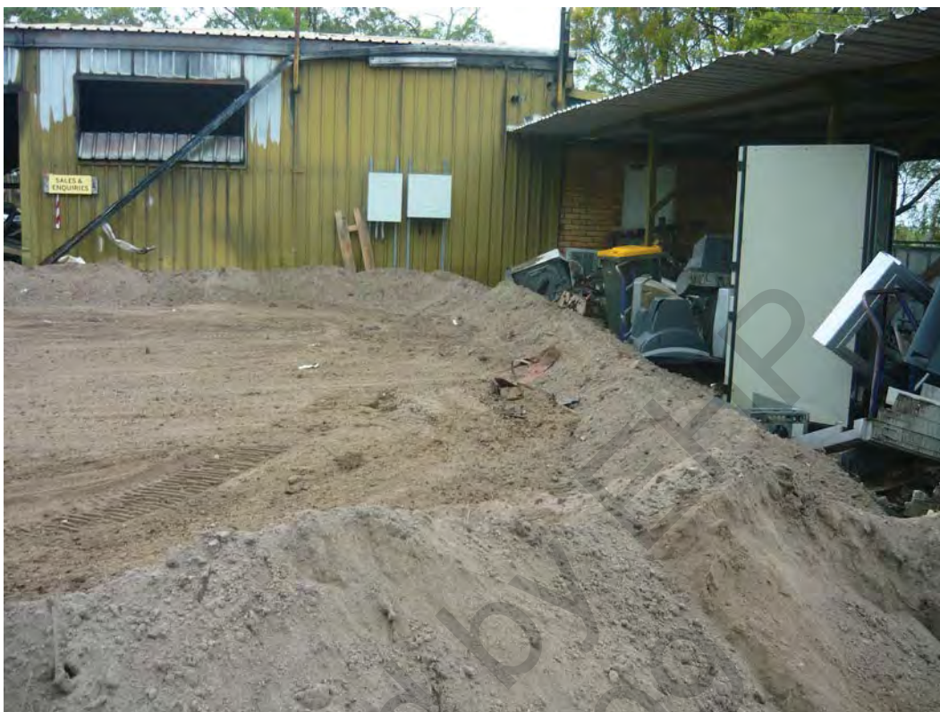
Photo 5 – The front of the main building (facing east) along Potassium Street. Note that the bunding has been reinforced with material and excess material has also been placed along the concrete slab to soak up any further containment in preparation for excess rainfall.
