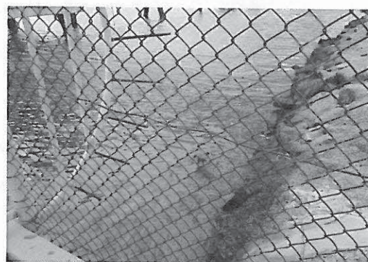
Figure 5-Area of Brisbane River impacted by the spill
