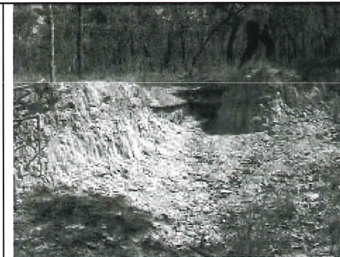
Erosion points, near Saltwater Pine Dam
