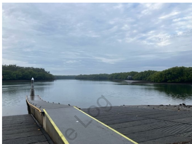
Plate 2: Shorncliffe boat ramp on 09/07/2024
