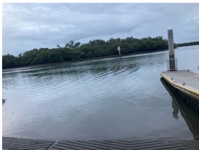
Plate 1: Shorncliffe boat ramp on 08/07/2024
