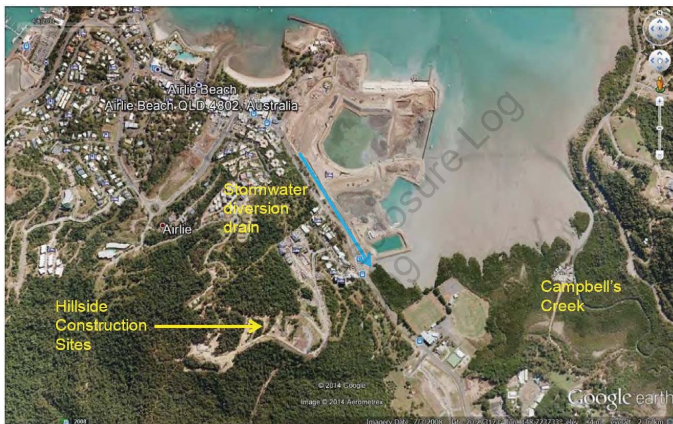
Figure F-1 Google Maps imagery on 7 th March 2008 showing a stormwater diversion drain
