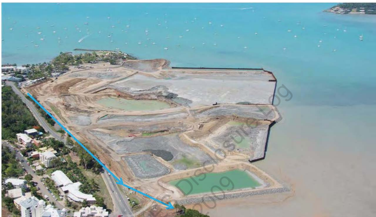
Figure F-2 Aerial photograph showing a stormwater diversion drain
