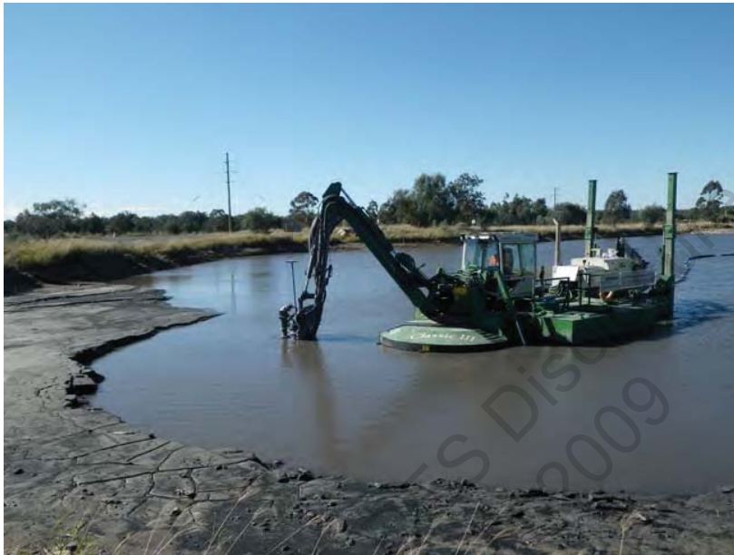
Pumping Coal - cutter suction pump
