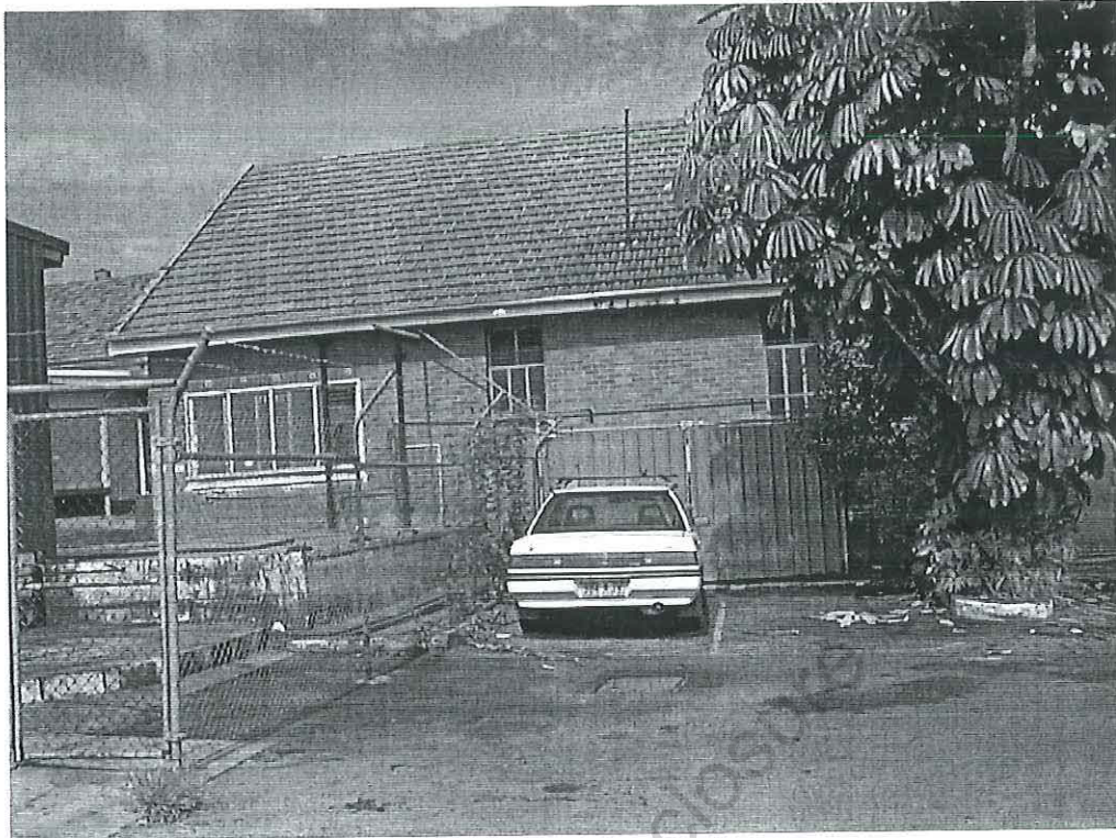
Photo 1 : Laundry boiler room located in background. Bulk fuel oil tank formerly located on a thick concrete slab to the left. Stand-by diesel generator and above ground storage tank formerly located on the thick raised concrete slab to the left.
