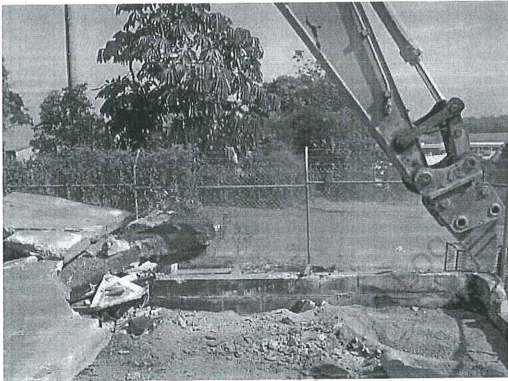
Photo 7 : Exposed thick concrete slab and soil (showing no signs of staining) below the former bulk fuel oil storage area.
