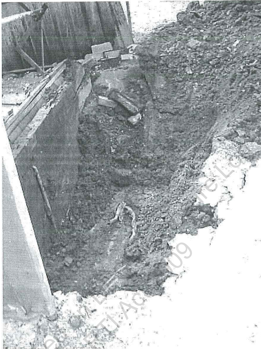
Photo 9 : Excavation of soil adjacent old ENERGEX transformer.
