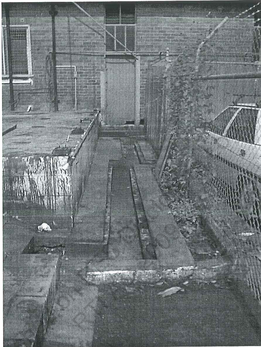
Photo 4 : Concrete lined channel containing the former fuel lines from the bulk fuel oil container to the boiler room.
