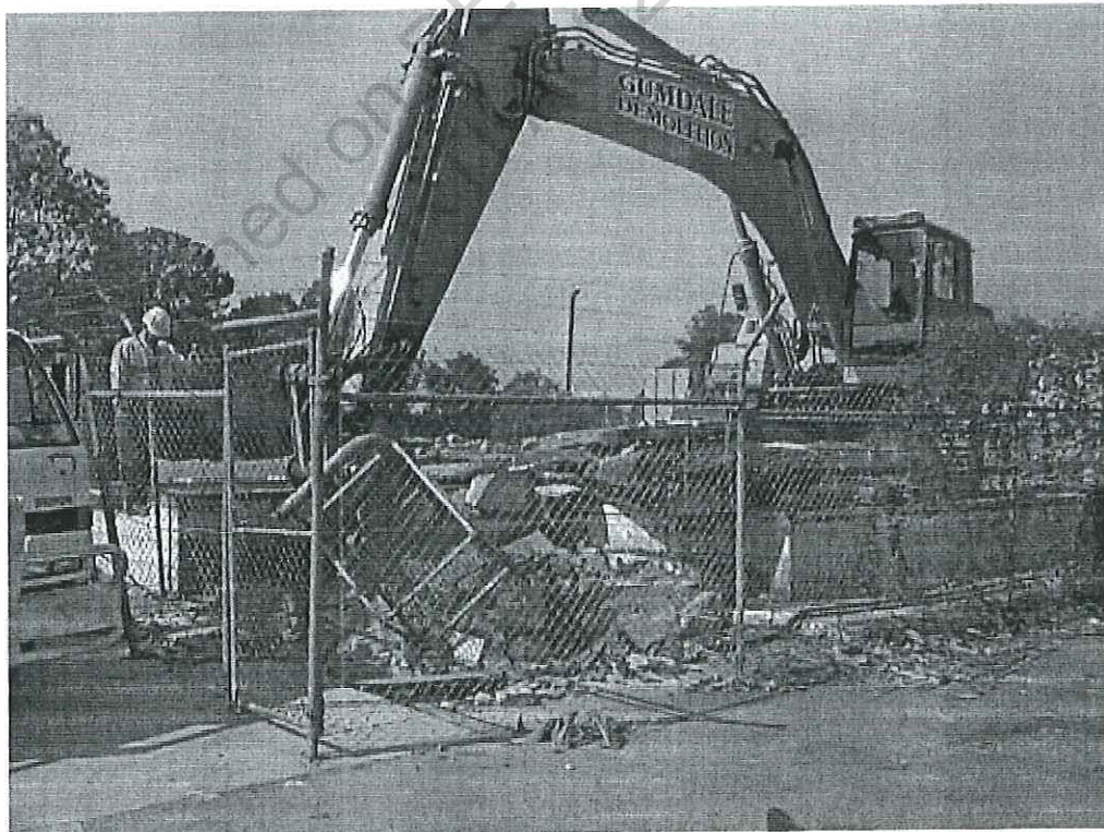
Photo 6 : Demolition of the slab below the former bulk fuel oil vessel.
