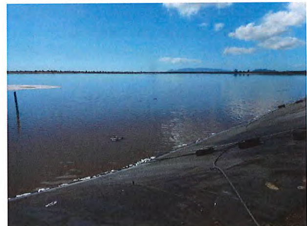
DSCN6685. Brine Pond Dam looking North East to spillway
