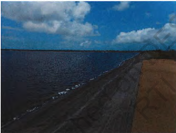
DSCN7798. Brine Pond spillway, looking north
