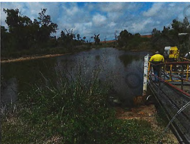
DSCN7765. Toe dam level
