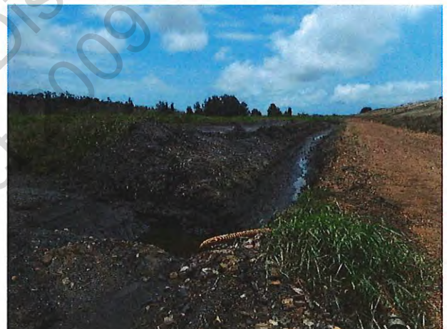
DSCN7782. Interception trench and sump west of the Brine Pond
