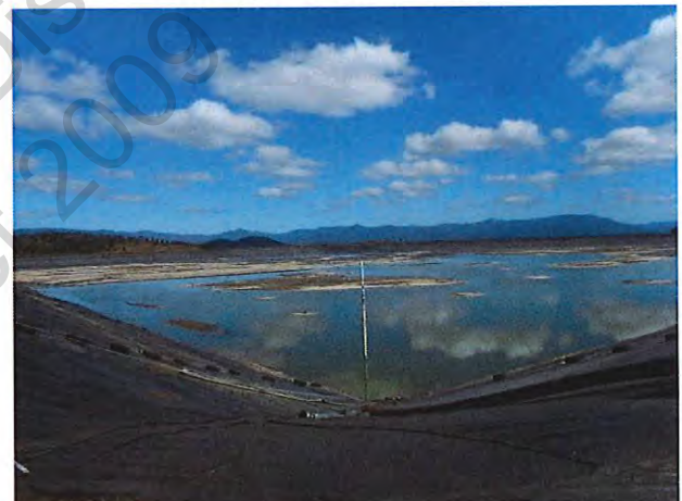
DSCN6681. Brine Pond Dam looking South West
