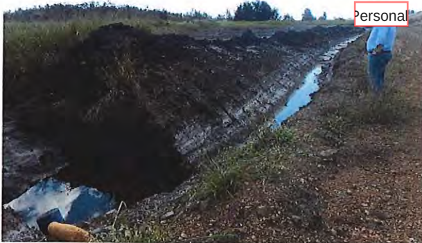
DSCN6687. Interception trench adjacent to West embankment of Brine Pond, looking north
