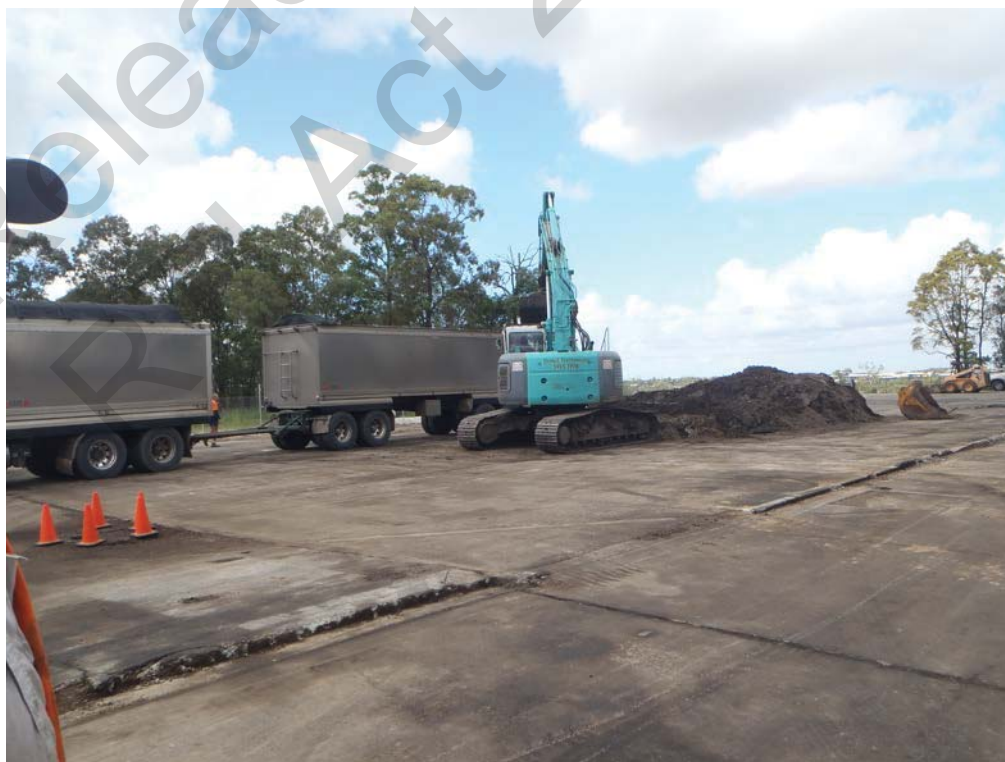
Photo 3 – Photo taken looking south-east from the potassium street entrance gate at the top of the property. Close up of the stock piles of contaminated soil were being loaded into a truck for disposal.
