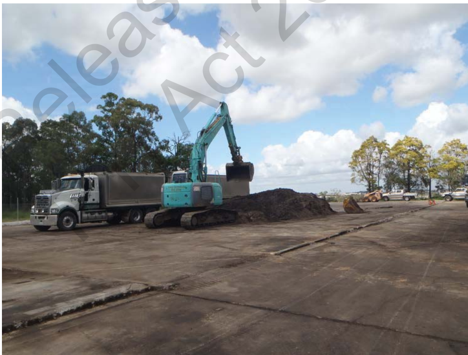
Photo 1 – Photo taken looking south-east from the potassium street entrance gate at the top of the property. Note that the stock piles of contaminated soil were being loaded into a truck for disposal.
