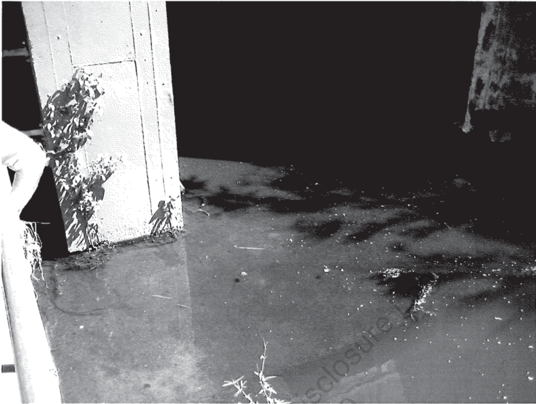
Figure 5. Monitoring point 5 at the junction of the stormwater drain and drains from ANZAC Avenue.
