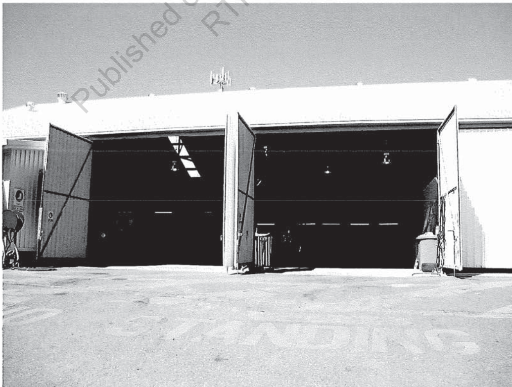
Photo 2 – The entrance of the motor vehicle workshop shed.
