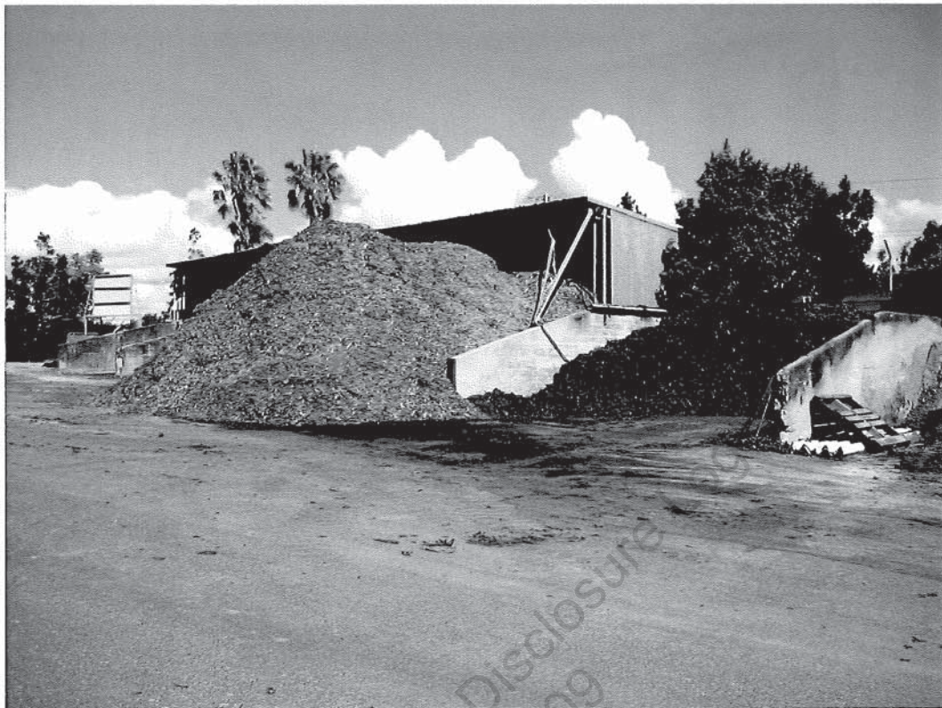
Photo 15 – Close up of the green waste (mulch) stock pile. Note the leachate pooling at the base of the pile.
