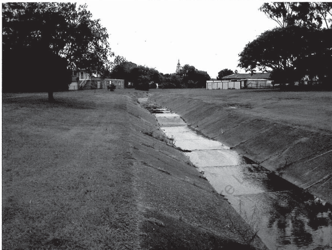
Figure 1. Monitoring site 1 and upper reaches of the stormwater drain.
