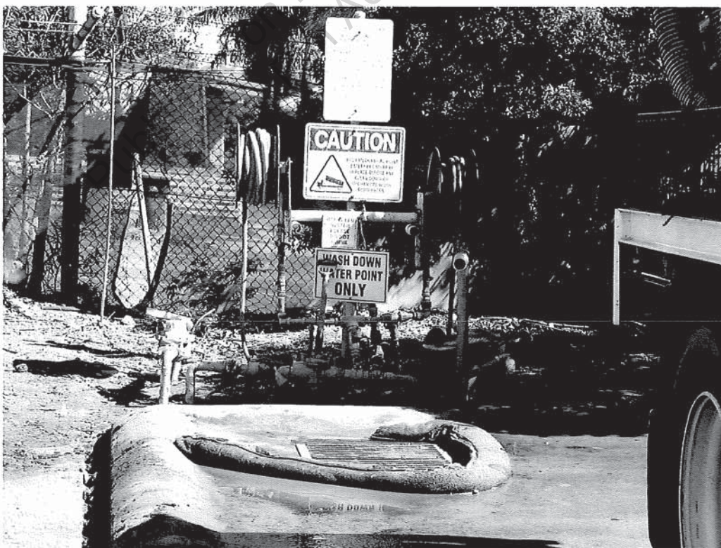
Photo 6 – The rear of the main wash bay showing the water system and sump. A temporary bund has been place around the sump.
