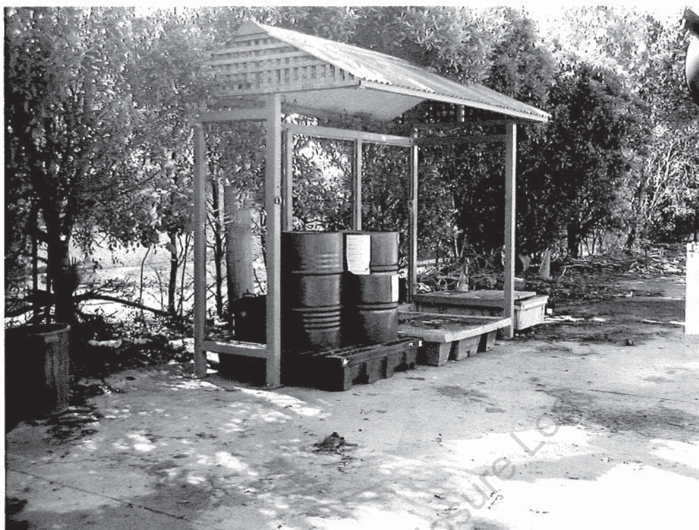
Photo 7 – Covered storage area for used drums and batteries. Used drums and batteries are then transported to a waste facility by a regulated operator. This area is situated to the north of the main wash bay.
