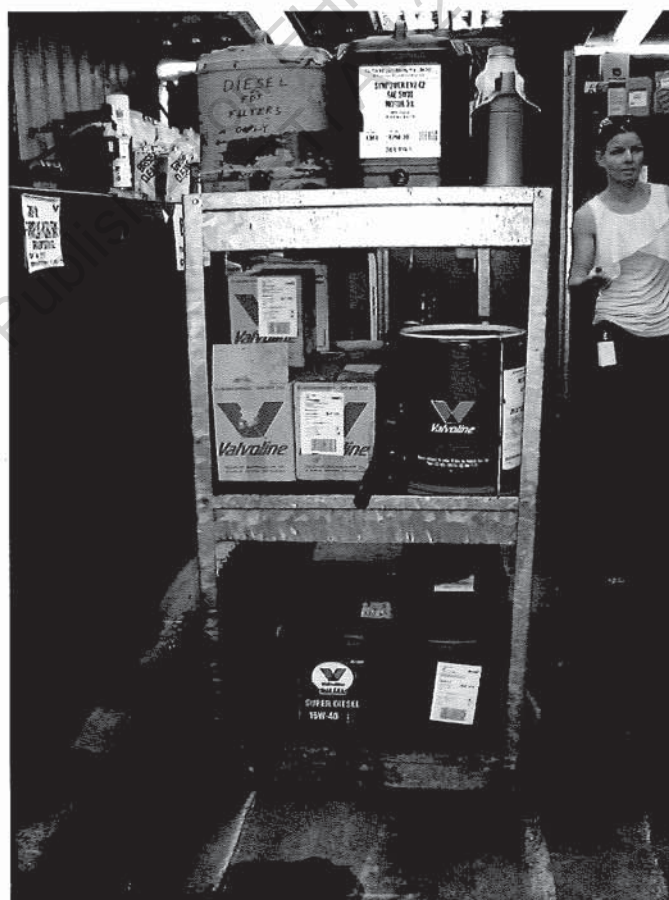
Photo 24 – Chemical storage room. Some chemicals are stored on a bunded stand. Note the asphalt bund on the left of the photo used for the larger tanks on the southern wall.
