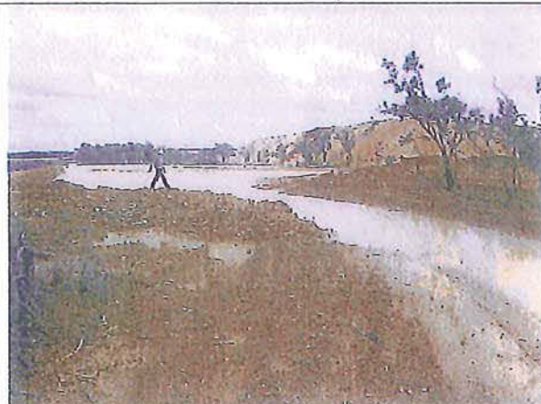
Figure 4- Sink hole diversion bund.
