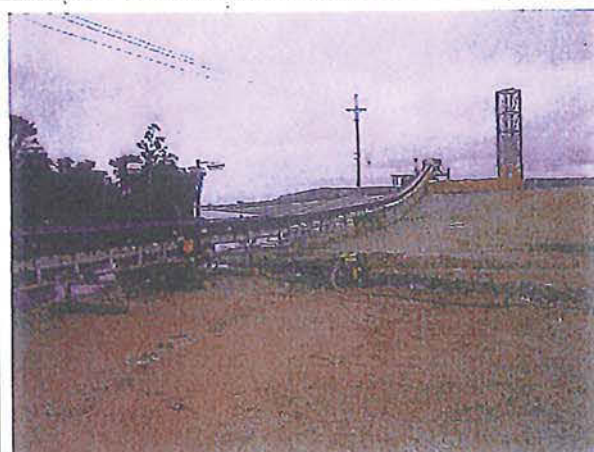
Figure 11- Pooled water adjacent to HLP.
