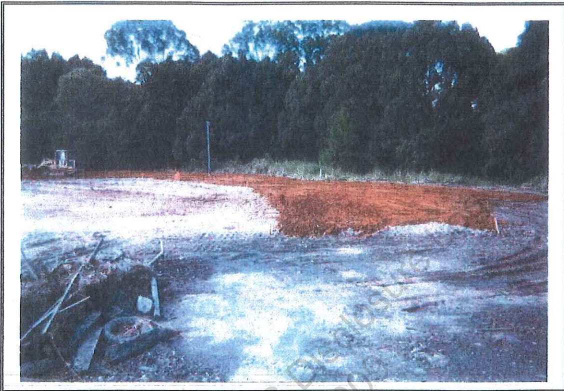
Photograph 1. Placement of soil cover (brown) over clay cap at evaporation pond (view looking north)
