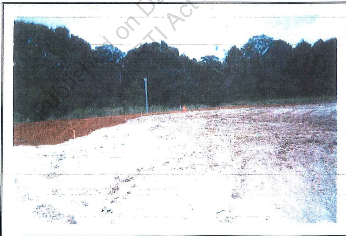
Photograph 2. Clean soil cover (brown) over clay cap at evaporation pond (view looking east)
