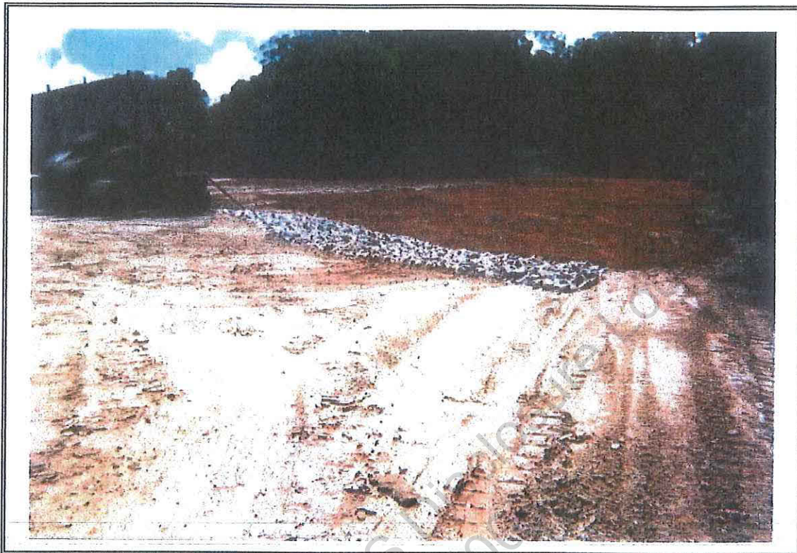
Photograph 3. Looking west into timber waste area – rock-hardened bank visible at centre, with clean soil (brown) spread throughout timber waste area.
