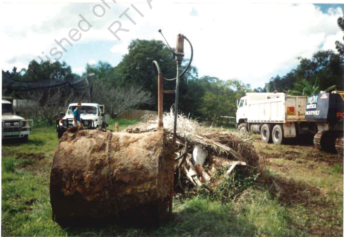
Photo 3. Fuel Tank (Removed)
