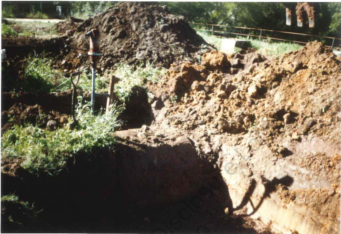
Photo 3. Fuel Tank (During Excavation)
