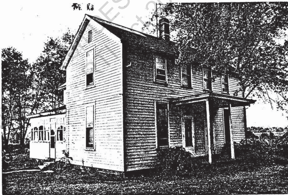
Figure 15.—Test structure 19, near a coal mine.
