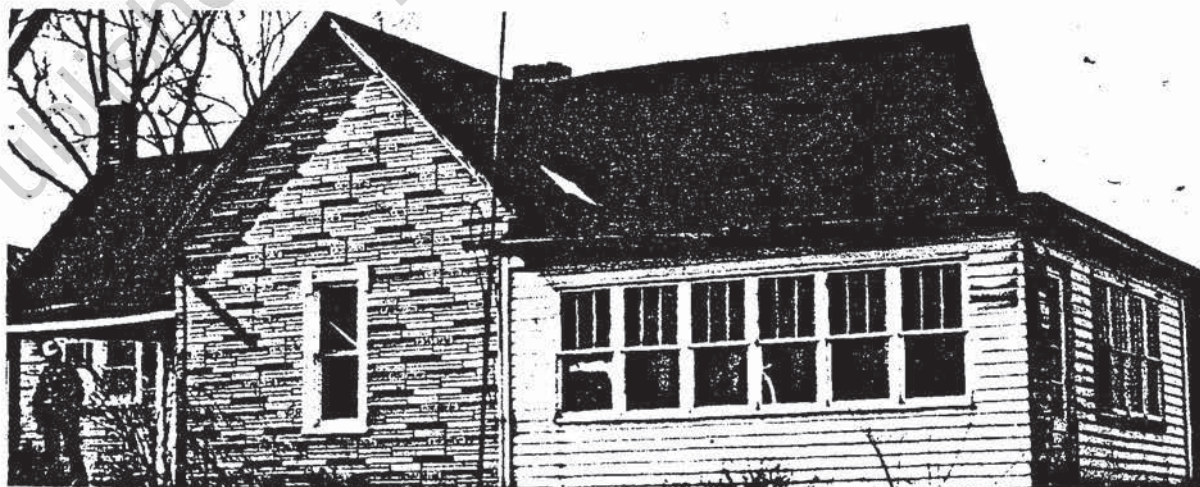
Figure 21.—Test structure 27, near a coal mine.
