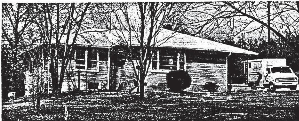
Figure 24.—Test structure 30, near a coal mine.
