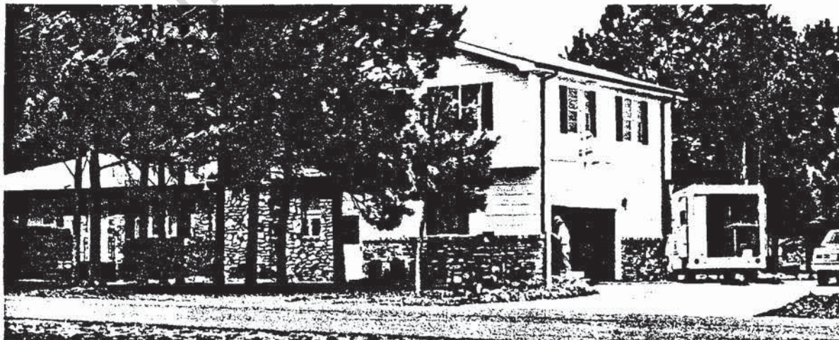
Figure 18.—Test structure 22, near a quarry.
