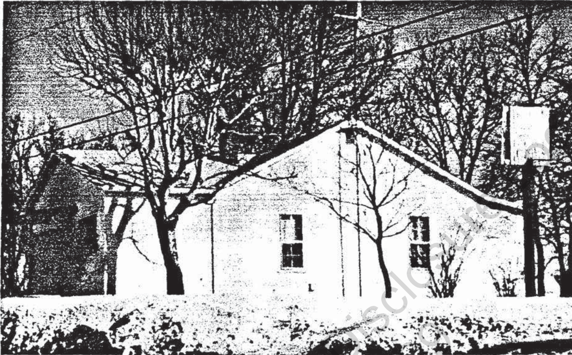
Figure 22.—Test structure 28, near a coal mine.
