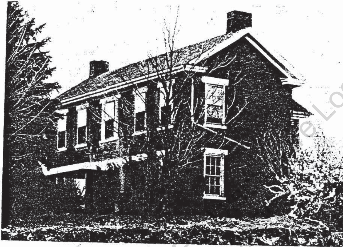
Figure 27.—Test structure 51, near a coal mine.
