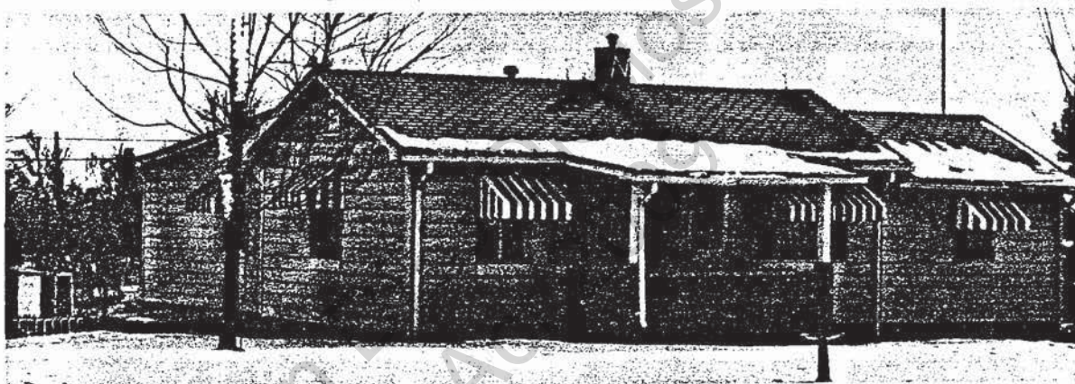
Figure 25.—Test structure 31, near a coal mine.
