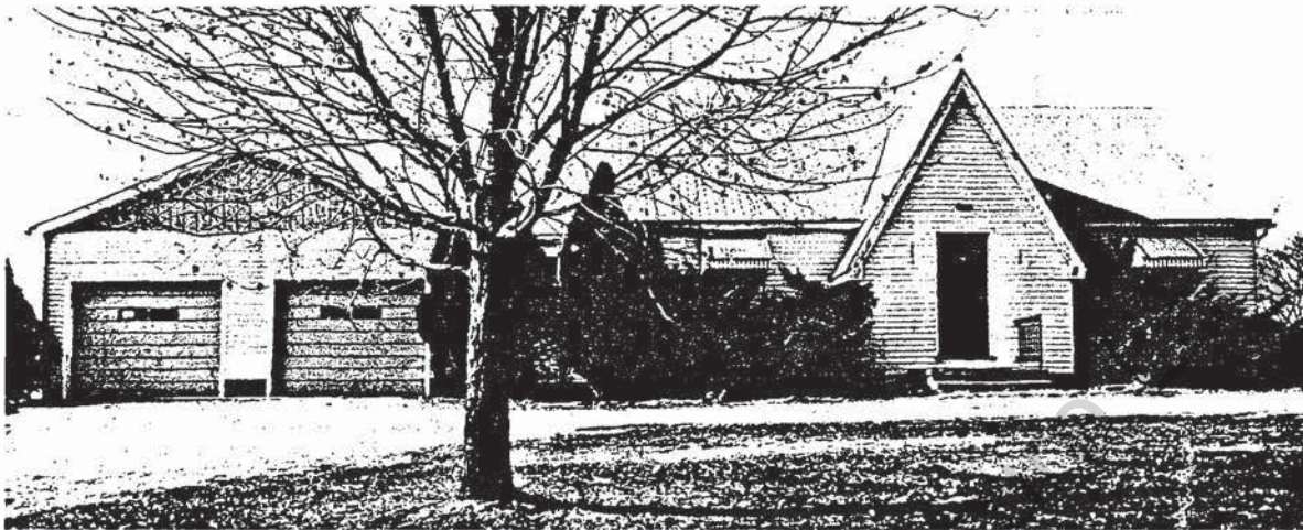
Figure 16.—Test structure 20, near a coal mine.
