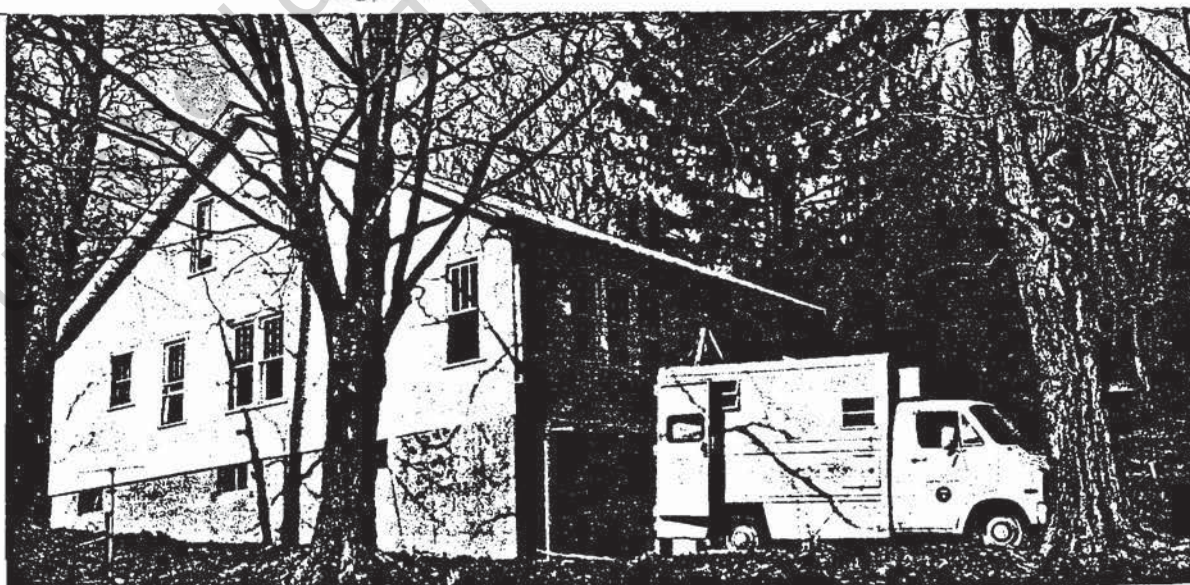
Figure 26.—Test structure 49, near a coal mine.
