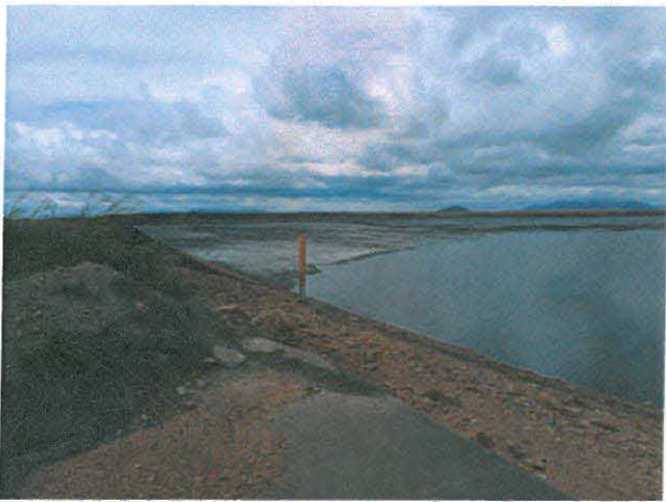
DSCN1919. MRL marker at spillway from Cell 3 of TSF
