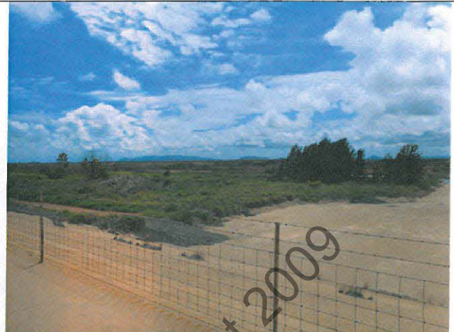
DSCN1903. Brine Pond spillway with stockpile area in background
