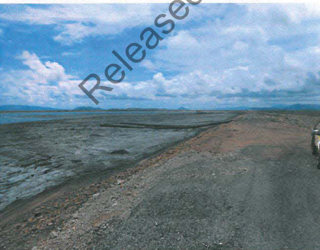
DSCN1909. Exposed tailings in TSF Cell 2.
