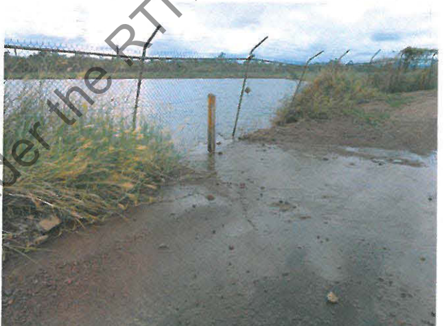
DSCN1907. Spillway of North West Pond, reporting to Levee banks
