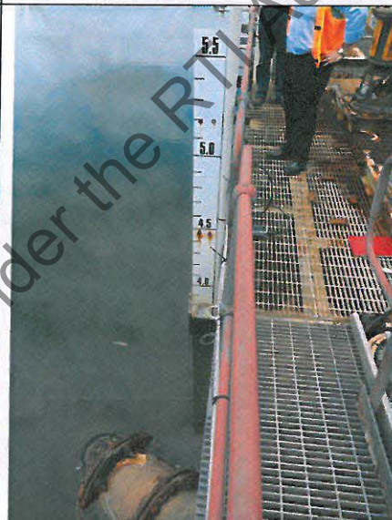
DSCN1927. Level marker in Toe Drain
