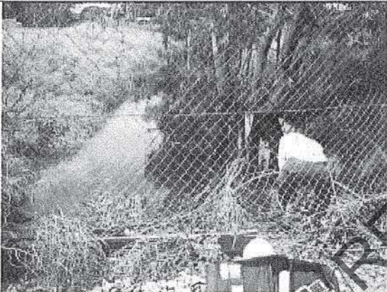
Figure 6: Upstream of the creek, just before the culvert crossing the railway.
