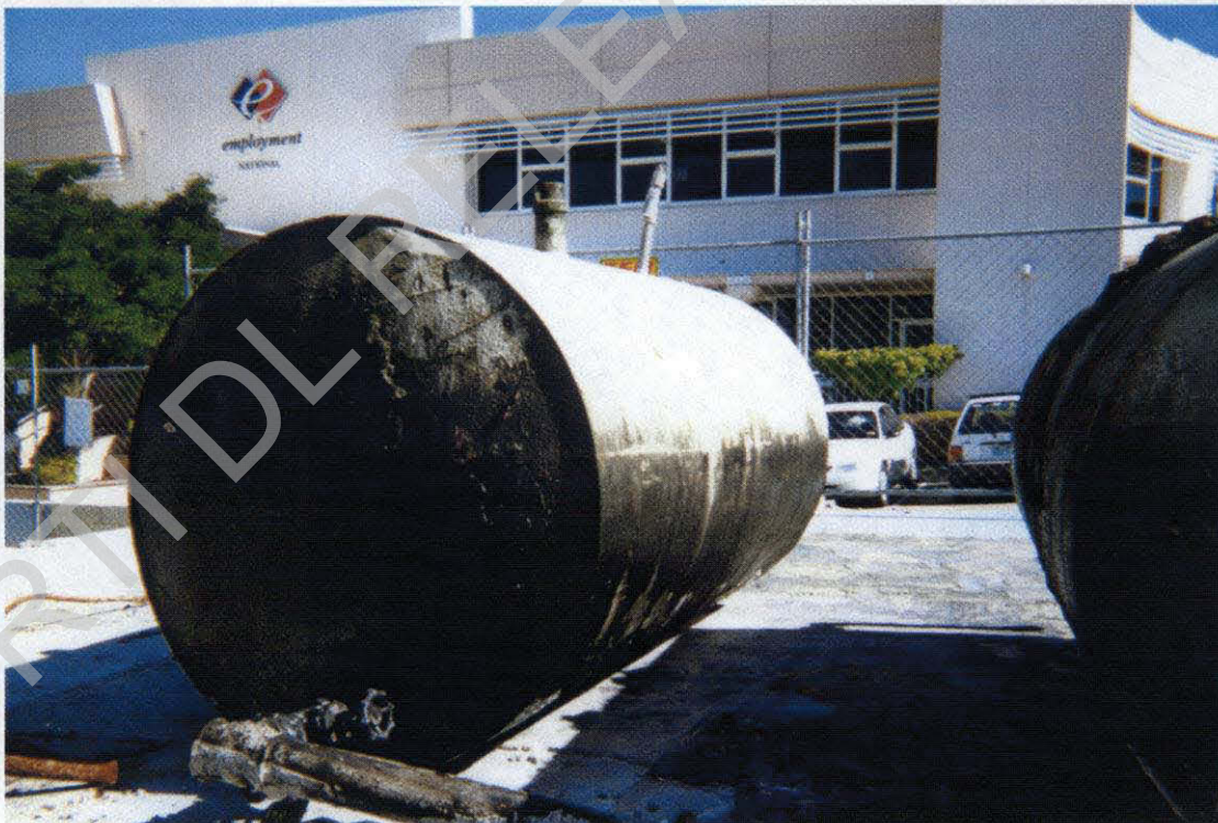
Plate 8: Photo of two 2,000L waste oil tanks prior to removal from site.
