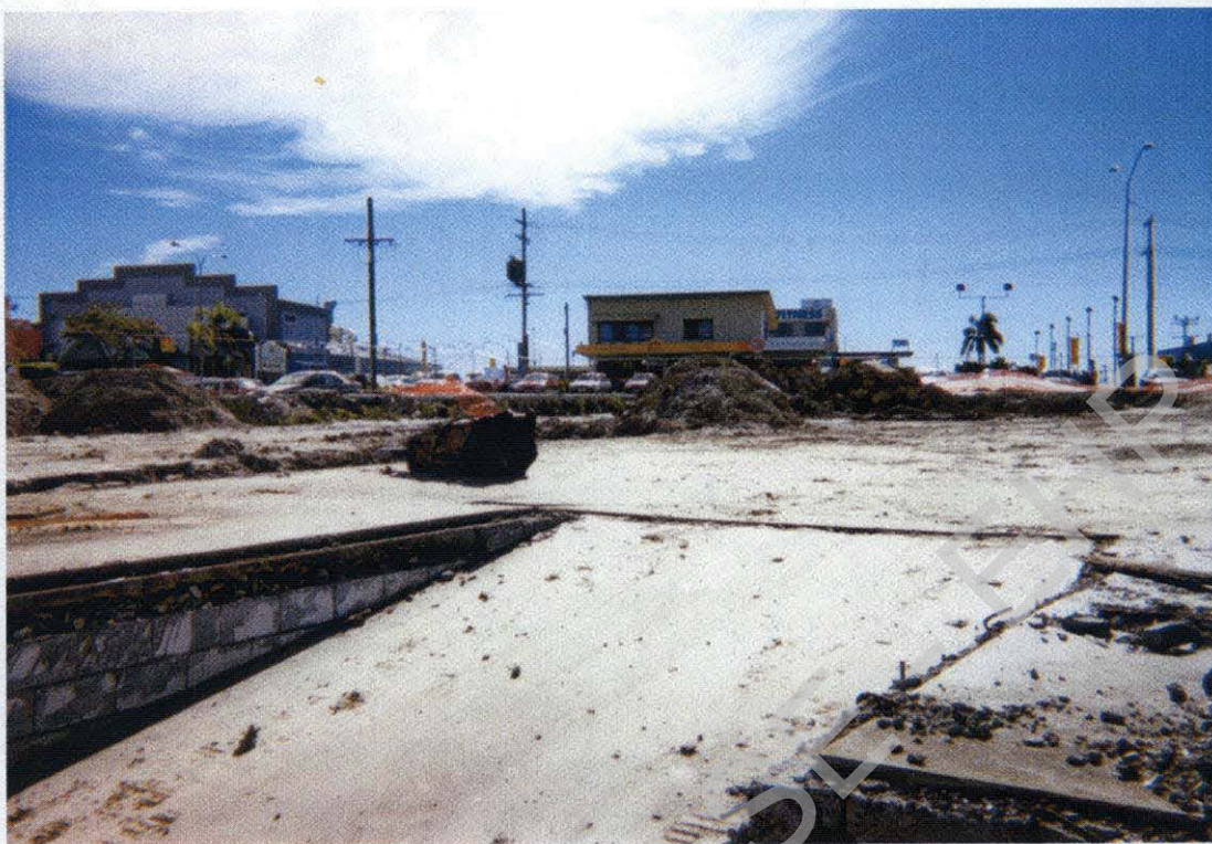
Plate 1: Photo of the site looking to the north showing commercial and retail buildings.
