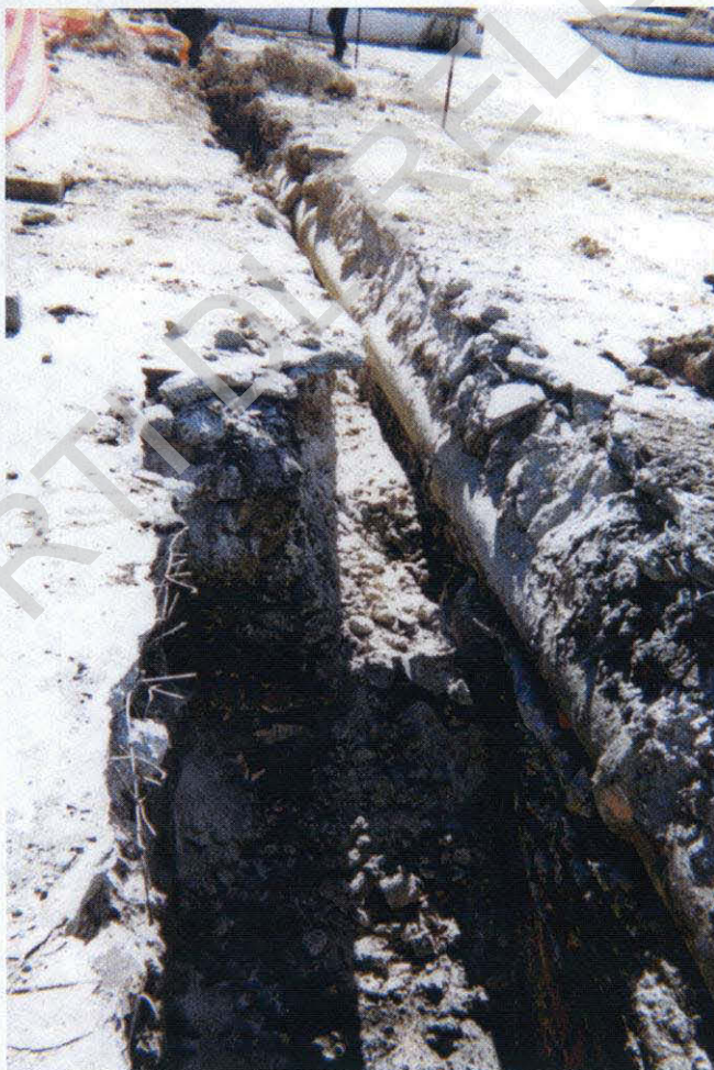
Plate 11: Photo showing the excavation of the waste oil line in the vicinity of sample location LL3. Note the damage to the concrete stormwater line.
