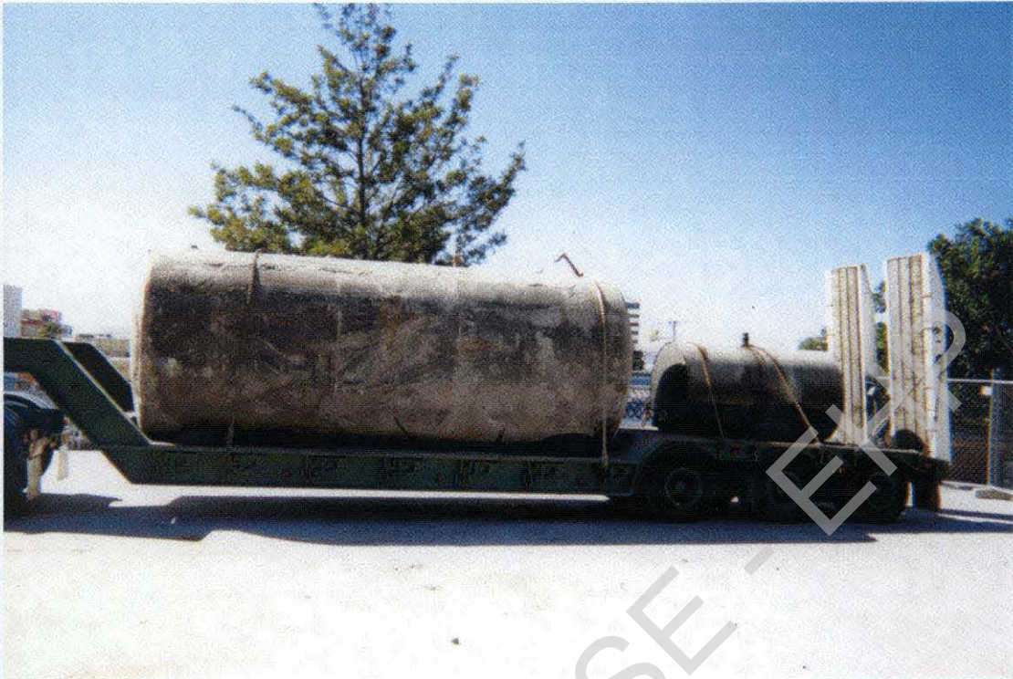
Plate 7: Photo of 15,000L and 2,000L USTs prior to removal from site.
