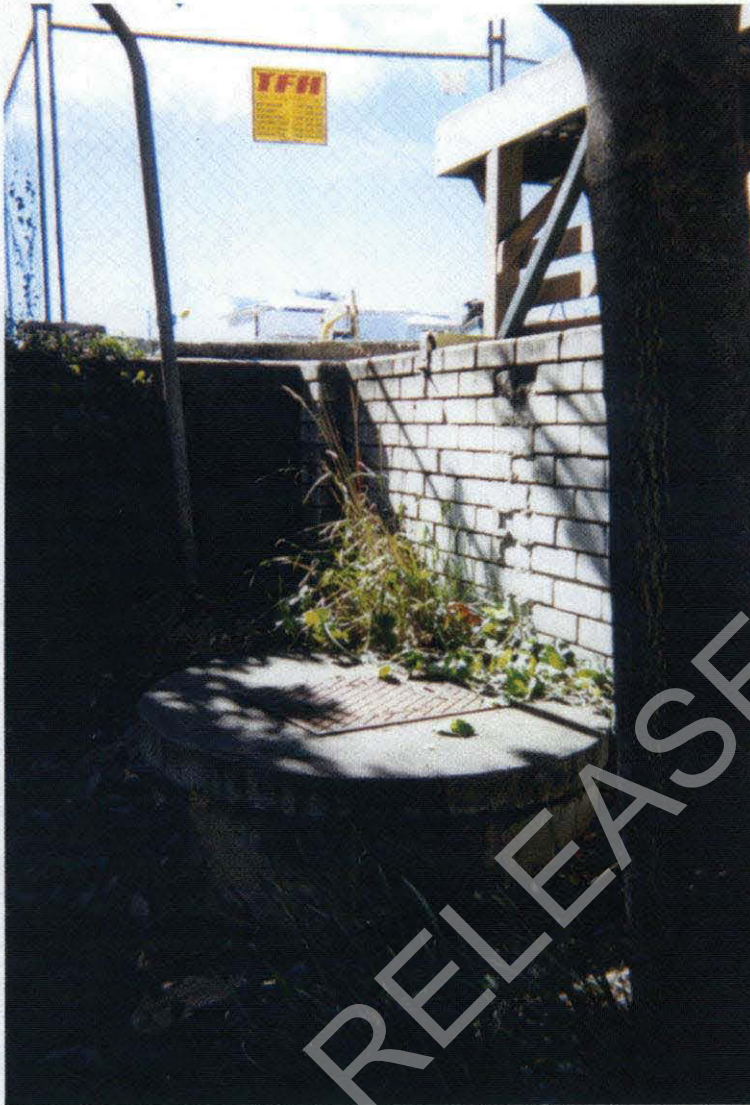
Plate 17: Stormwater manhole adjacent to southern boundary of the site.
