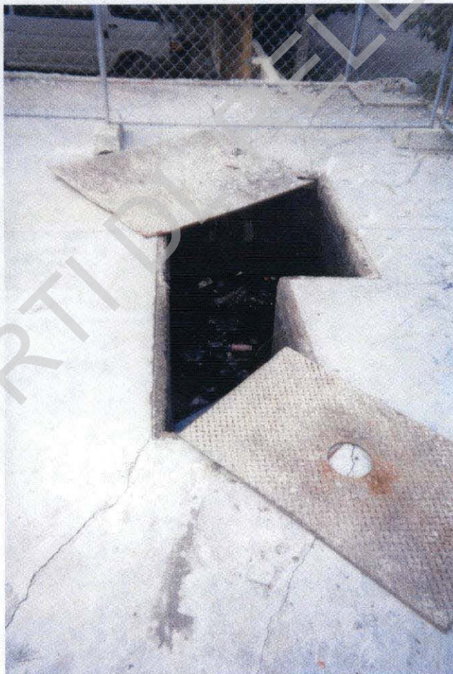
Plate 9: Waste oil pit prior to excavation of material and soil sampling. Note refuse is heavily contaminated with waste oil.
