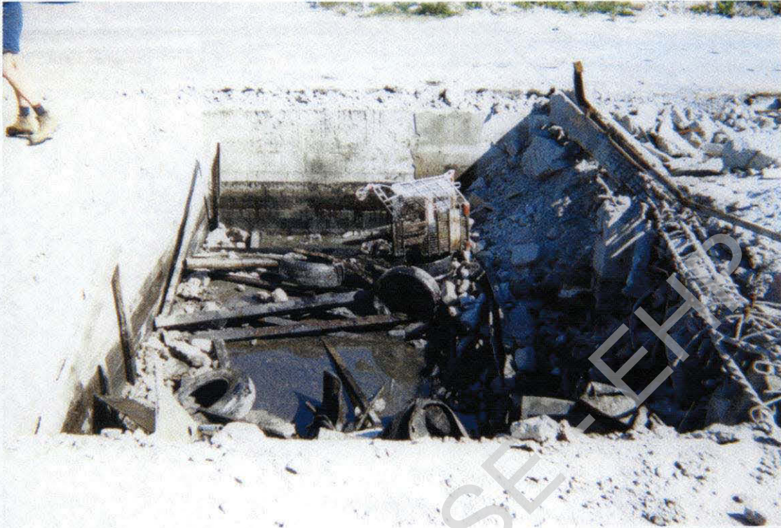
Plate 9: Waste oil pit prior to excavation of material and soil sampling. Note refuse is heavily contaminated with waste oil.
