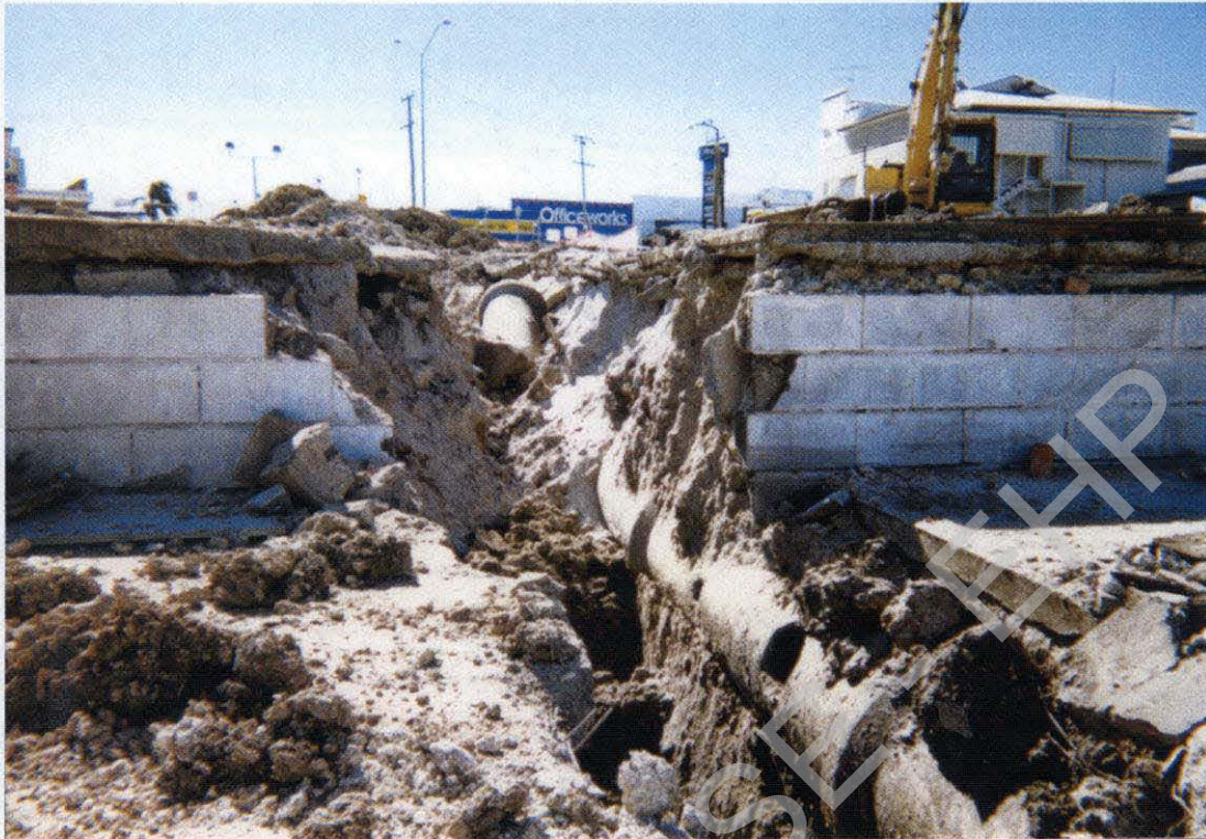
Plate 11: Photo showing the excavation of the waste oil line in the vicinity of sample location LL3. Note the damage to the concrete stormwater line.
