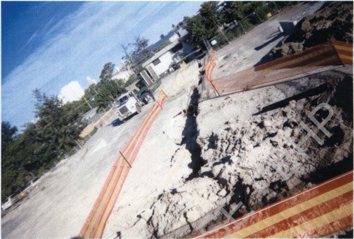
Plate 15: Photo looking south over site at the completion of JFT contracted removal of infrastructure phase of works. Note that the site is temporary fenced, gates locked and all excavation pits have high visibility barricading in place.
