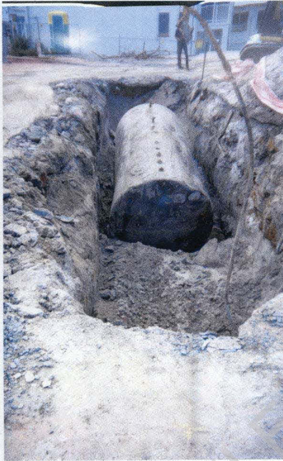
Plate 5: 15,000L UST uncovered at northern end of the site.
