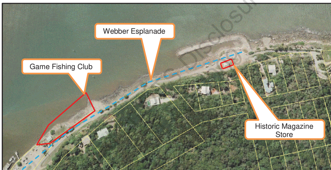
Figure 1: Aerial showing key infrastructure and start of construction of the revetment wall (May 2011)
