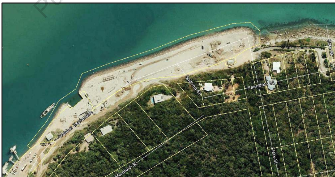
Figure 2: Aerial showing progressed construction of wall as at July 2015
