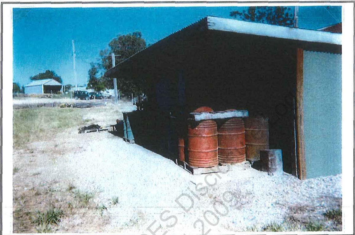
Photograph 7. Ash and Sawdust drum storage shed. Drums are removed from site by contractor. Monitoring Well MW6 is located to right of telegraph pole at rear (Area F - view south).
