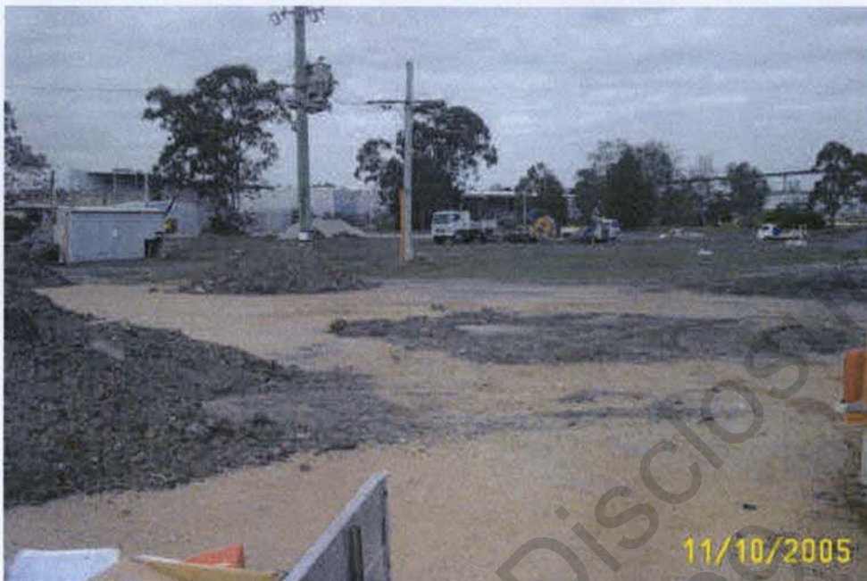
Photo 1: View of small substation, power poles and topsoil stockpiles looking west across Lots 2, 3 and 4.
