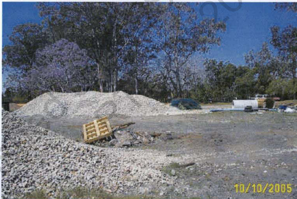
Photo 2: Stockpiles of cobbles and gravel
