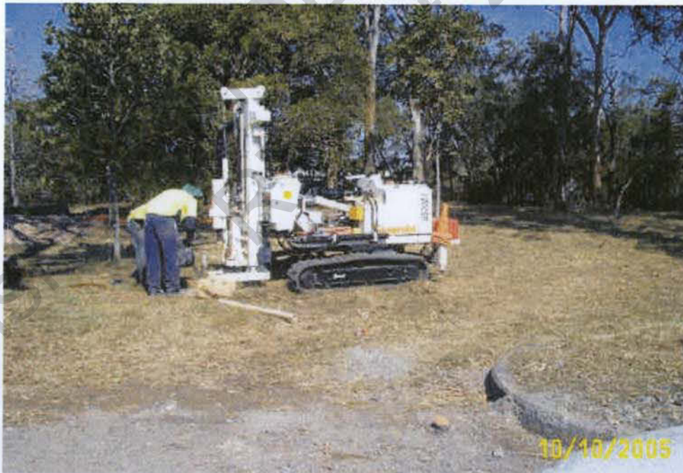
Photo 4: Bore hole 20 and groundwater monitoring well on Lot 5 looking south toward Aquarium Passage.
