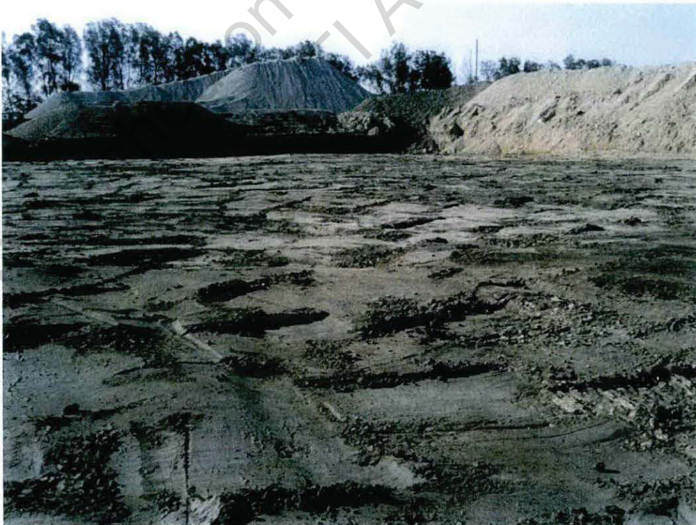
Photograph 2: View of excavation base, December 2009
