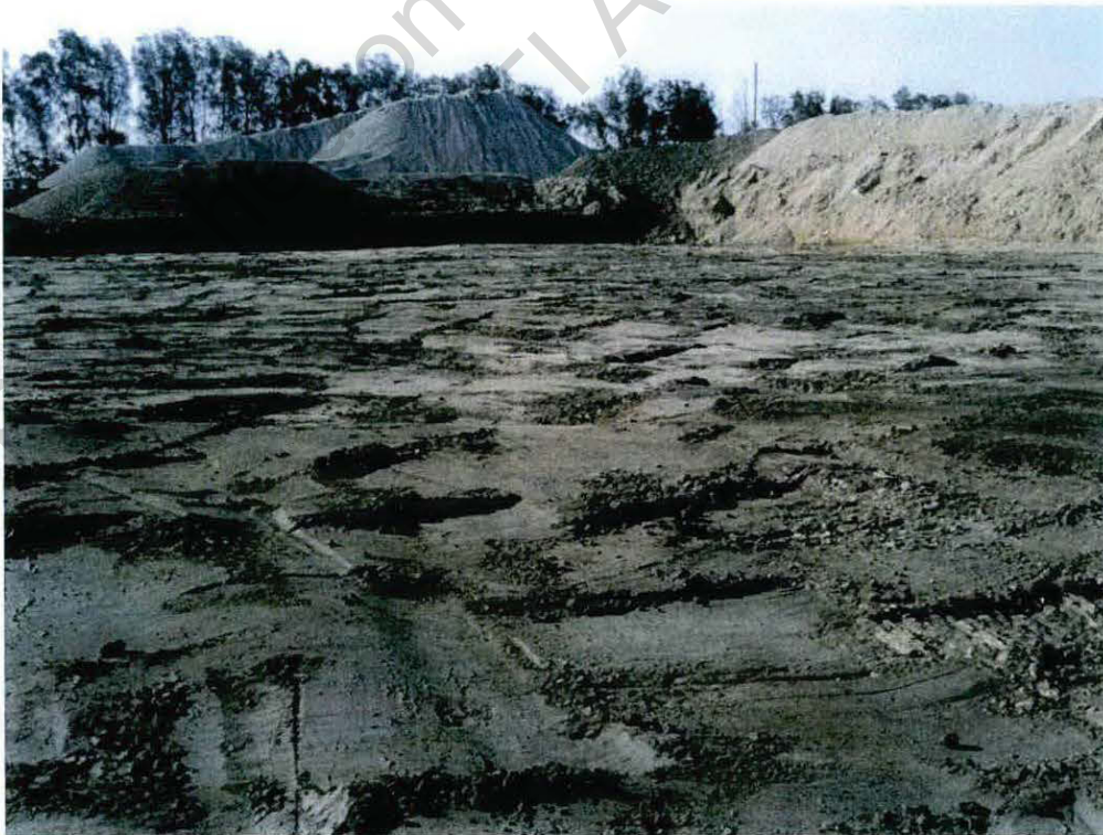
Photograph 2: View of excavation base, December 2009
