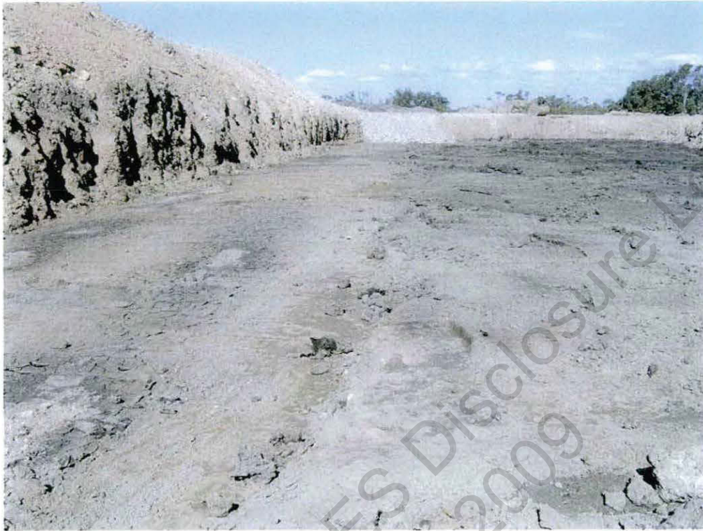
Photograph 1: View of excavation base, September 2009
