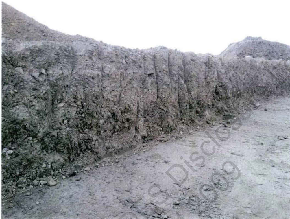
Photograph 3: View of excavation base and imported fill material placed following the remediation and validation of an adjacent area
