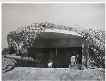
On 9 July 1943, Army engineers mounted the 4.7 inch gun in the second emplacement (lower on the hill slope). Note the tent in the background, most likely soldiers' sleeping quarters.
