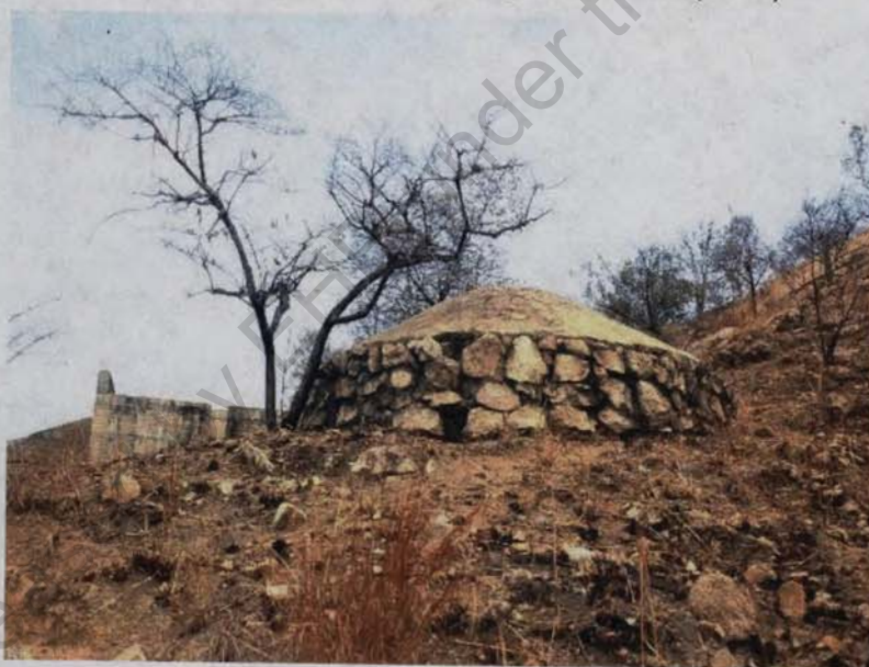
2. Former Operations and Signals Bunker (1996)
