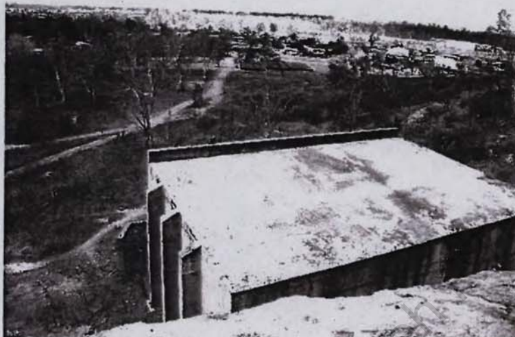
1. Former Operations and Signals Bunker (1996)
