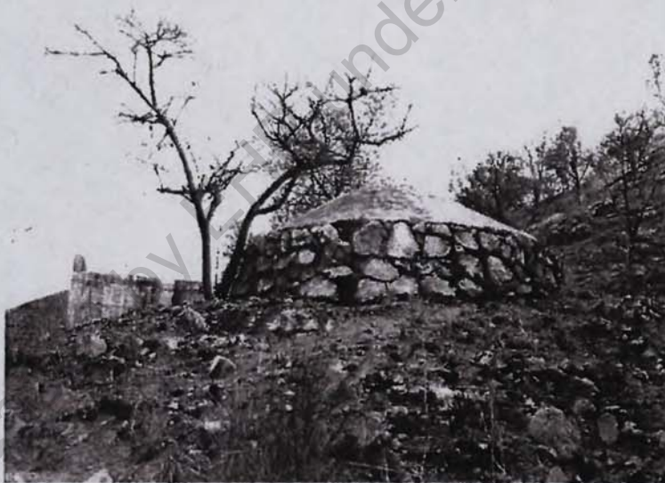
2. Former Operations and Signals Bunker (1996)
