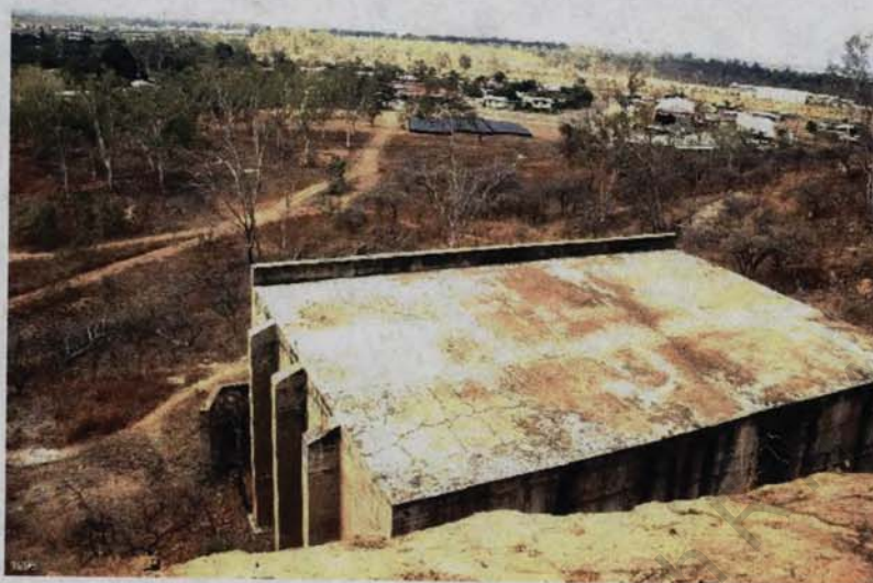
1. Former Operations and Signals Bunker (1996)
