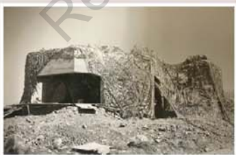
The first searchlight position with light installed inside. These lights were used to sweep across the ocean at night, not to search the sky for aircraft. Photo taken in July 1943.
