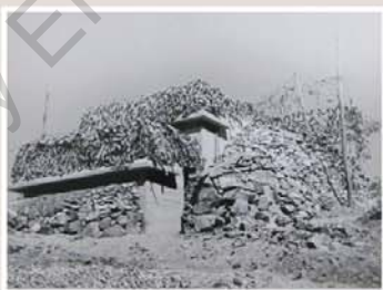
The observation post, or command post and ELDS (Electric Light Directing Station), was the nerve centre of Pallarenda Battery. It was connected to the gun emplacements and searchlights by telephone and directed all surveillance and operational tasks. The range chart on the wall inside shows they used a wreck in the bay between here and Magnetic Island as target practice. Photo taken in July 1943.
