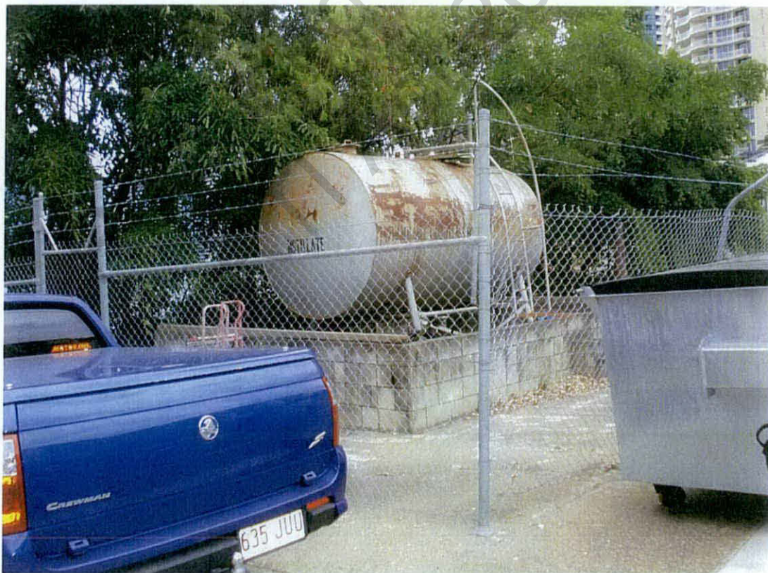
View of disused diesel AST (Lot 3).
