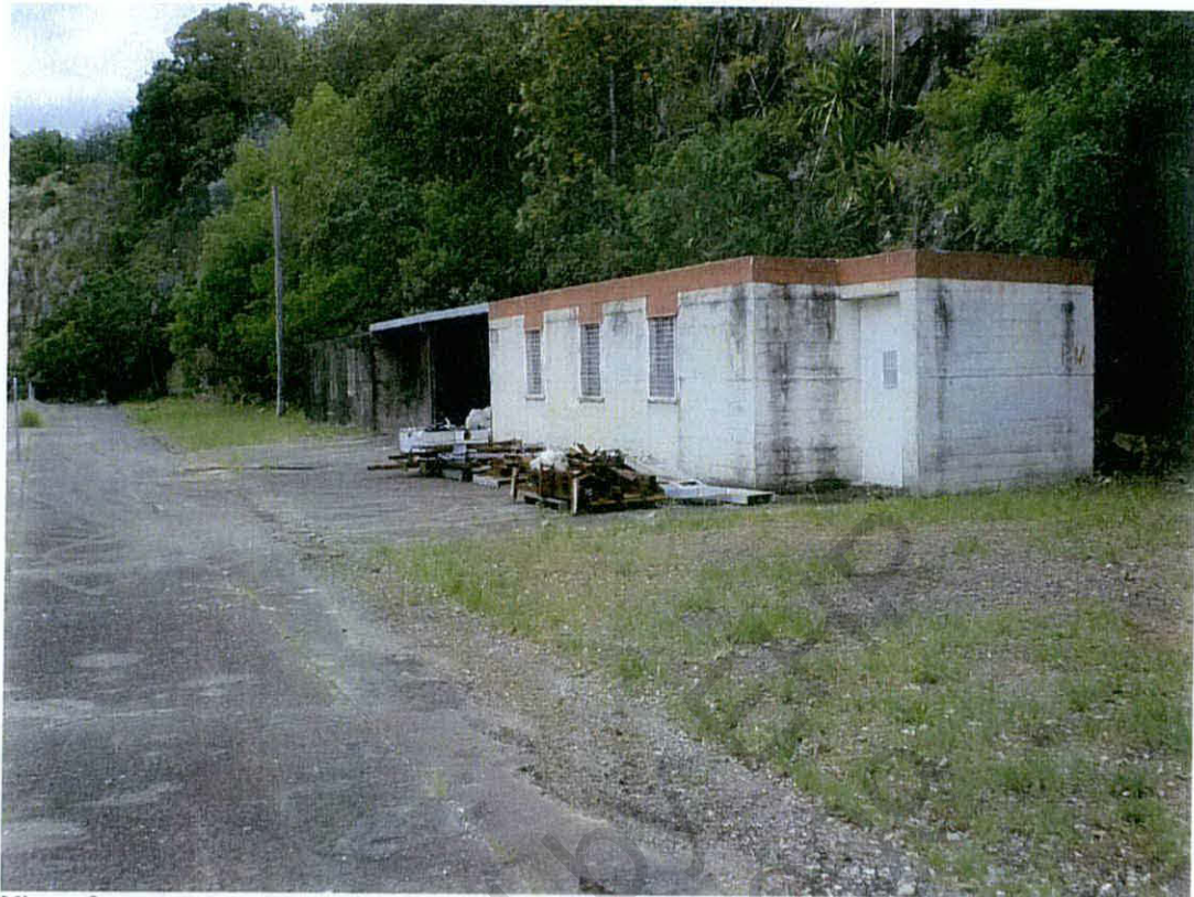
View of masonry structure on Lot 4
